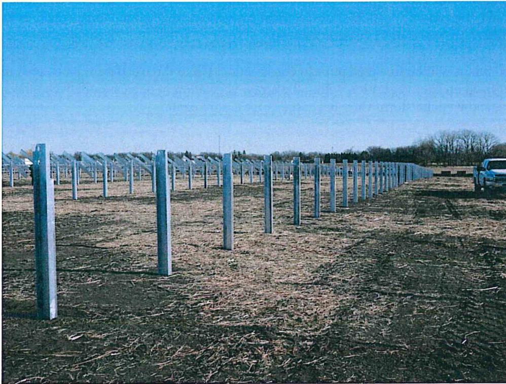
Image 5 – Standard Steel Pier Foundations
