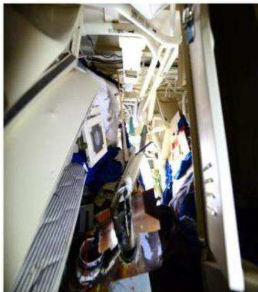
Figure 16 – Berthing 3 facing port after collision
