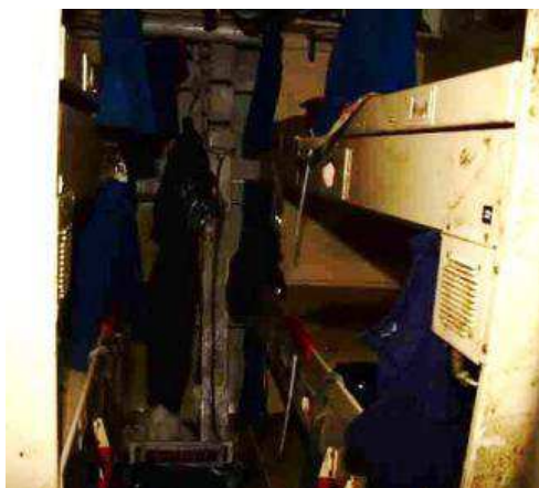
Figure 18—Berthing 4 racks after dewatering
