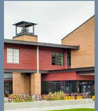
Newest School Buildings 2019
