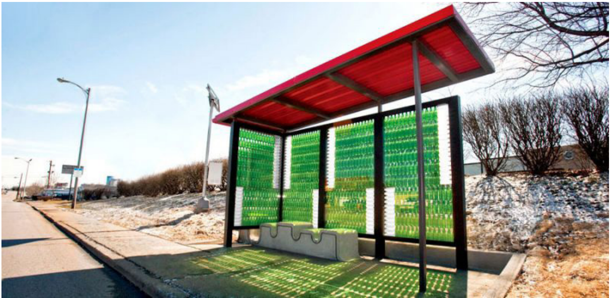
Figure 3.5. “Trash to Treasure” transit stop reuses soft drink bottles in Lexington, Kentucky. SOURCE: HTTPS://NEXTCITY.ORG/DAILY/ENTRY/PUBLIC-ART-BUS-STOPS-PHOTOS
