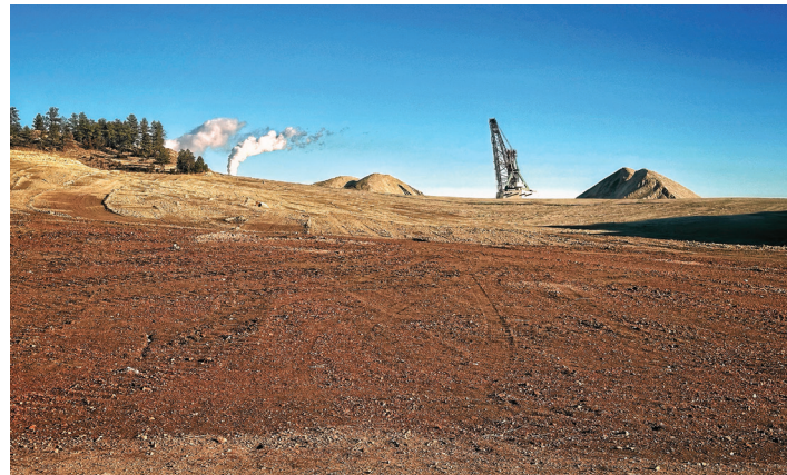
Reclamation activities at the Rosebud Mine near Colstrip. The mine is owned and operated by Westmoreland. The steam rising over the horizon is from the Colstrip power generating station. You can also see the contrast between the cover soil and the ground being reclaimed.
