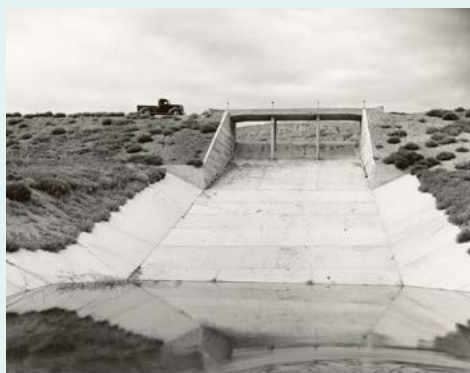
The overflow spillway at Anita Reservoir on the Huntley Project, built by Civilian Conservation Corps workers ca. 1934 MHS PAC 2003-47-135
