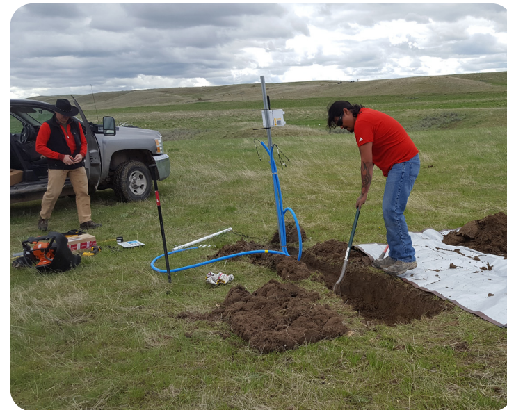
Installing a weather station Photo courtesy of John Doyle
