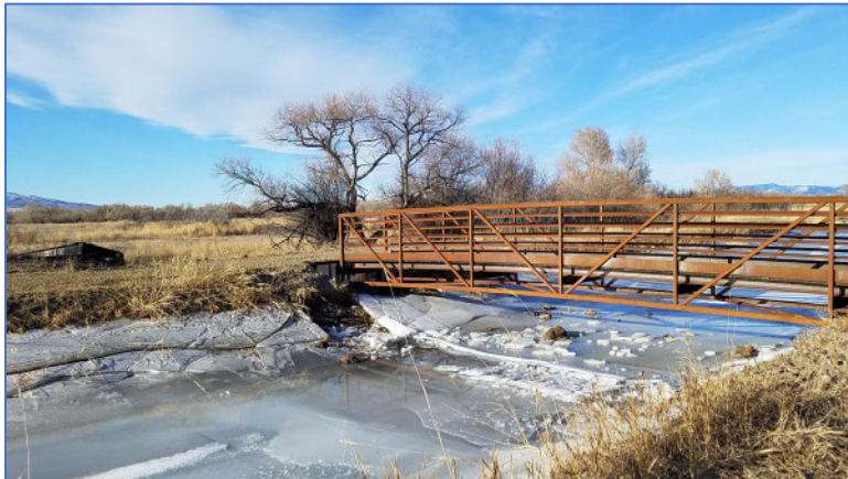
Recently installed pedestrian bridges on Canyon Ferry Wildlife Management Area near Townsend (Image: K. McDonnell).
