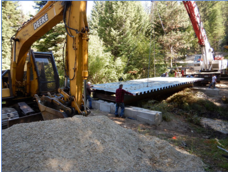
Bridge replacement (2020) on Threemile Wildlife Management Area near Florence, funded using Habitat Montana and Forestry Program dollars (Image: J. Parke).
