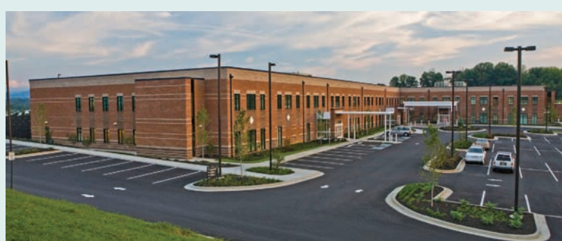
State of Franklin Healthcare Associates main campus, 301 and 303 Med Tech Parkway, across from Franklin Woods Hospital.
