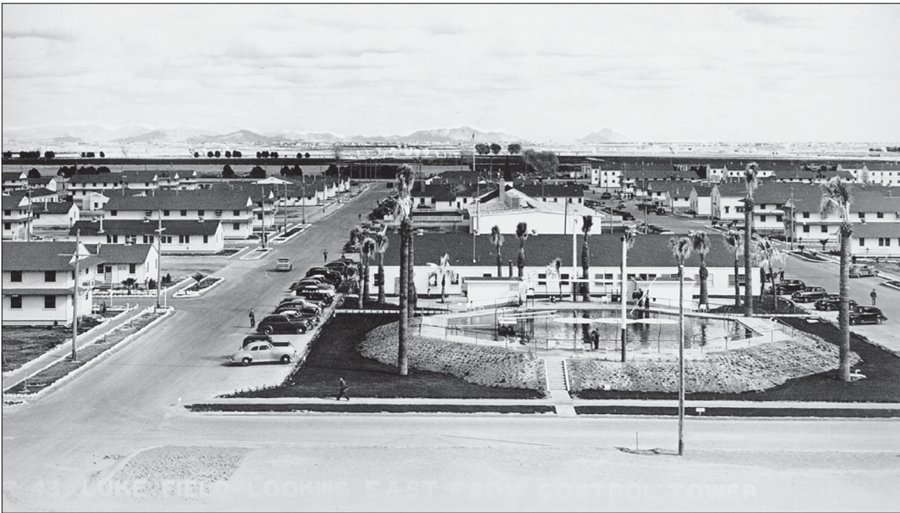
A view to the east from the control tower of Luke Field on Feb. 9, 1943, revealed completed construction of the base.
