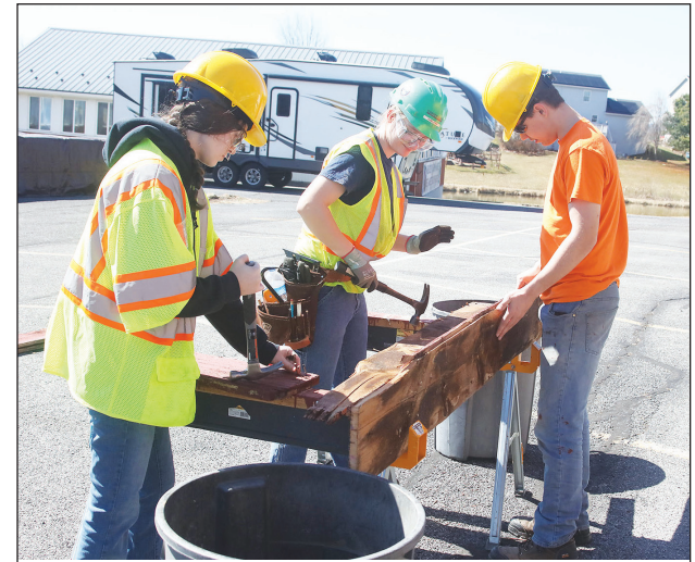
From left, Emma Haines, Isabella Fair and Keegan Yost remove nails from the old siding that was taken off the Ditzler Barn in Biglerville. (Darryl Wheeler/Gettysburg Times)
