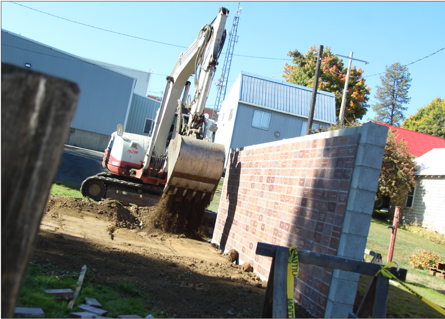
A contractor works to fill in around the foundation of the new wall behind the Hughes House Museum. The wall will now display the bricks bearing the names of Hughes House supporters that were previously set in a walkway behind the museum.
