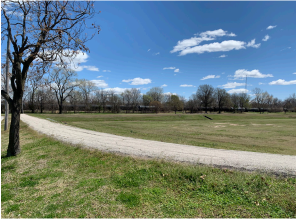
Stormwater Detention Basins (WRT)
