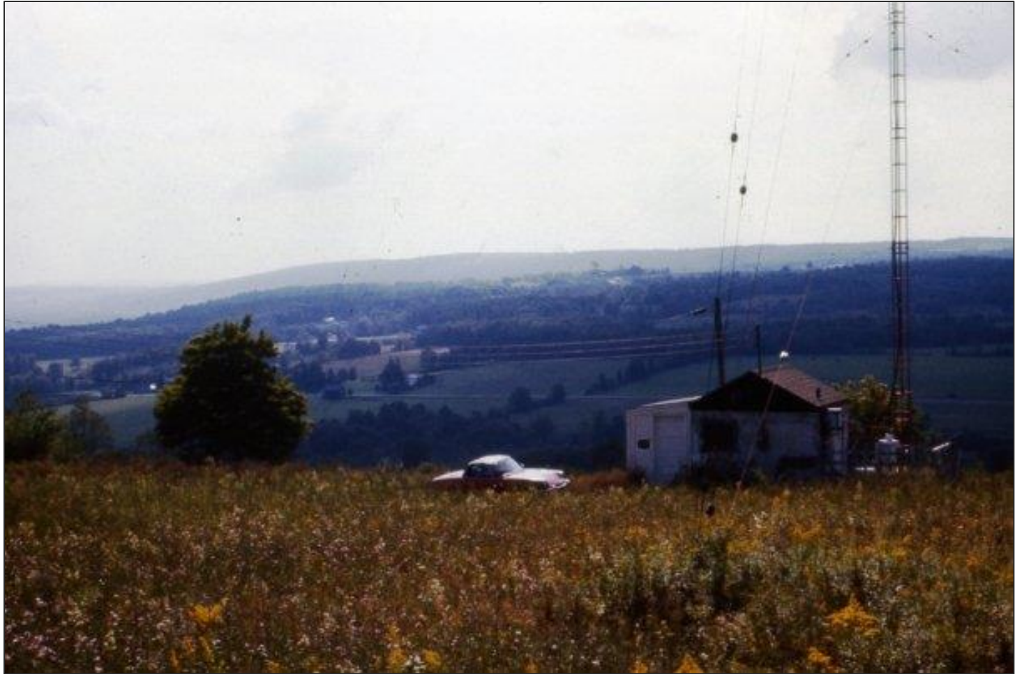
The WFLR transmitter and tower location near Dundee.
