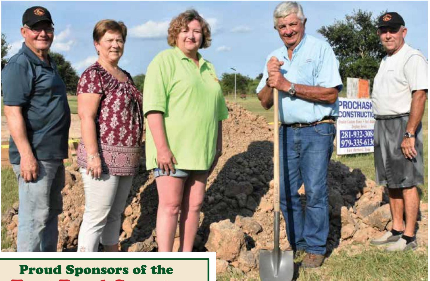
The newest addition to Harvest Park in Needville got under way in August. On hand to watch the start of construction on a new covered pavilion alongside the jogging trail were, from left, Harvest Festival Committee members W. Lee Hedt, Sandra Wendt, Sherry Winkelman, Tommy Stavinoha and Chris Janicek.
