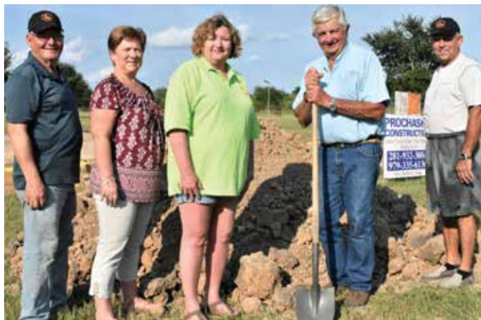
The newest addition to Harvest Park in Needville got under way last week. On hand to watch the start of construction on a new covered pavilion alongside the jogging trail were, from left, Harvest Festival Committee members W. Lee Hedt, Sandra Wendt, Sherry Winkelman, Tommy Stavinoha and Chris Janicek.
