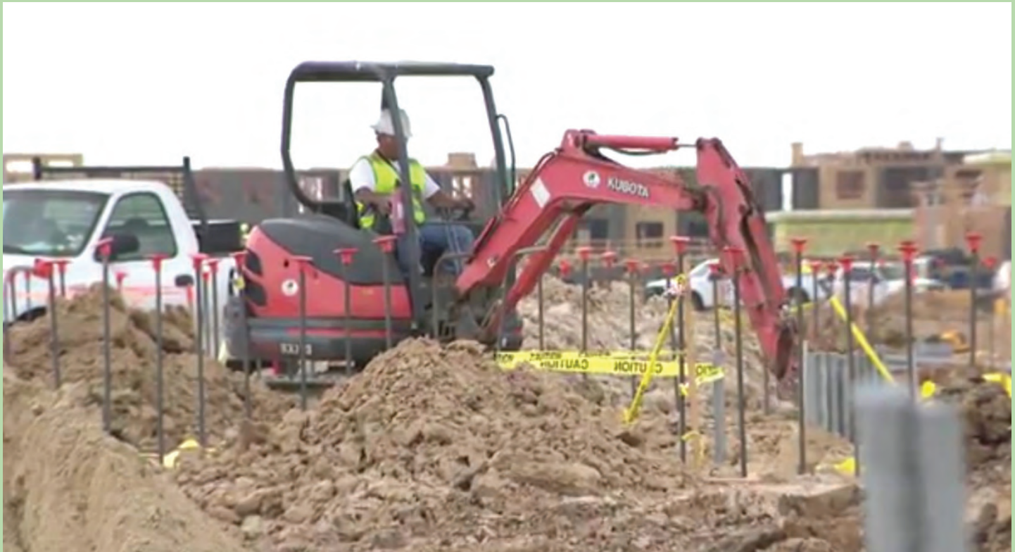
Construction has already begun on the new school, which will open for the 2020/2021 school year.
