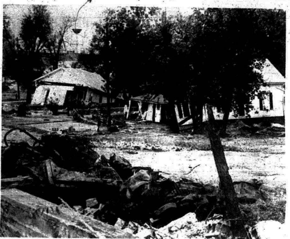
In Wake Of Flood Surging flood waters ravaged this area just blocks from End's downtown square. 15.62 inches of rain between 4 and 6 p.m. Wednesday and 2 a.m. today caused heavy flooding in several sections of the city. The houses above, on the 400 block on N. Third St., appeared to have been hoisted from their foundations by the flood and resettled after heavy damage as floodwaters receded.
