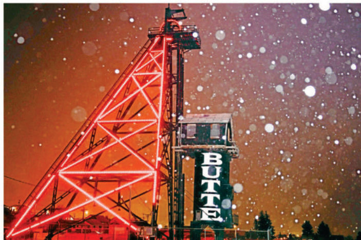
The historic Travona mining headframe lights up a snowy night in Butte, Montana.
