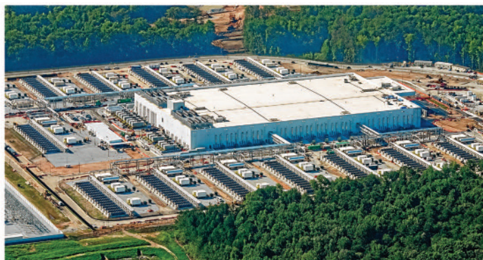
The QTS Fayetteville Data Center complex in Fayetteville, Ga. on July 18.
