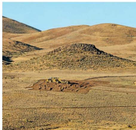
Pre-construction work began at the South Railroad Project southeast of Carlin in Elko County the day after the U.S. Bureau of Land Management gave the project its approval.
