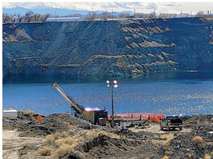
Angle drilling at the Yerington pit.
