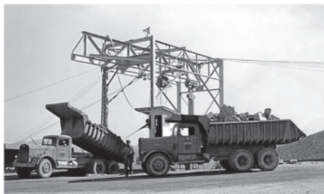
Trucks unload ore at the Basic Magnesium, Inc. plant in Gabbs, Nevada.
