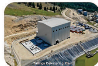
Tailings Dewatering Plant
