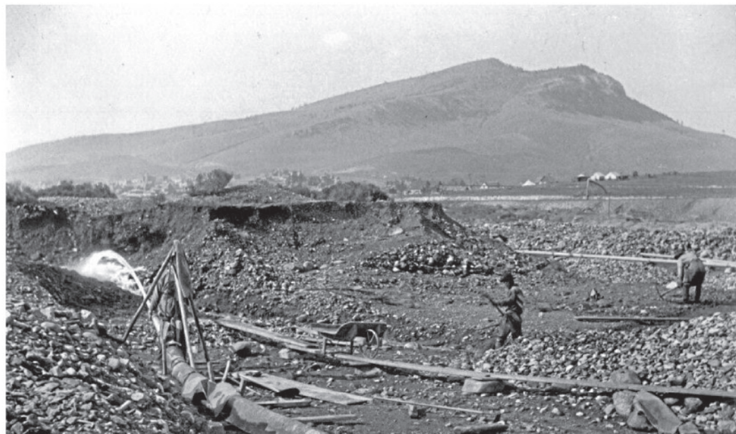
View of a hydraulic mining operation in Last Chance Gulch north of Helena, Montana, with Mount Helena and the city in the background. A few men are visible working, one with a wheel barrow and one with a pick axe. Another miner operates the water hose shooting a stream of water at the dirt and rocks.
