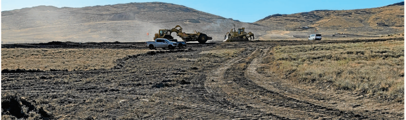
Equinox Gold started initial construction work on Aug. 15, the day after the U.S. Bureau of Land Management issued a decision record approving the South Railroad gold and silver mine project in Elko County.
