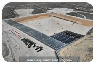
New Heap Leach Pad progress
