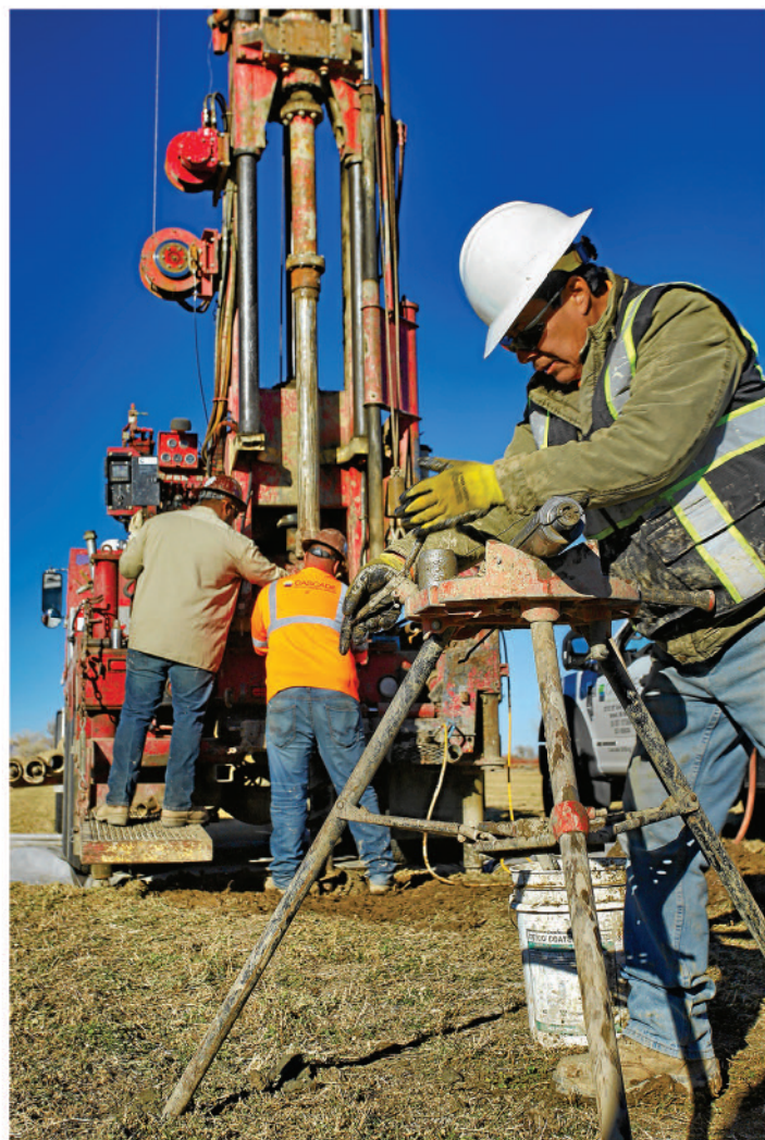
Drilling teamwork at the Yerington Copper Project.
