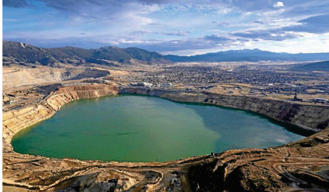
The open pit mine by Butte, Montana filled with water after the dewatering pumps in the underground mine network were shut off in 1982. Researchers are now looking at options for extracting critical minerals from the water in the Berkeley Pit.
