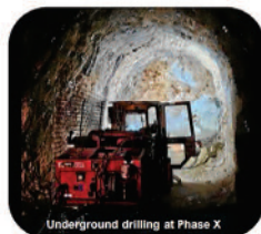
Underground drilling at Phase X
