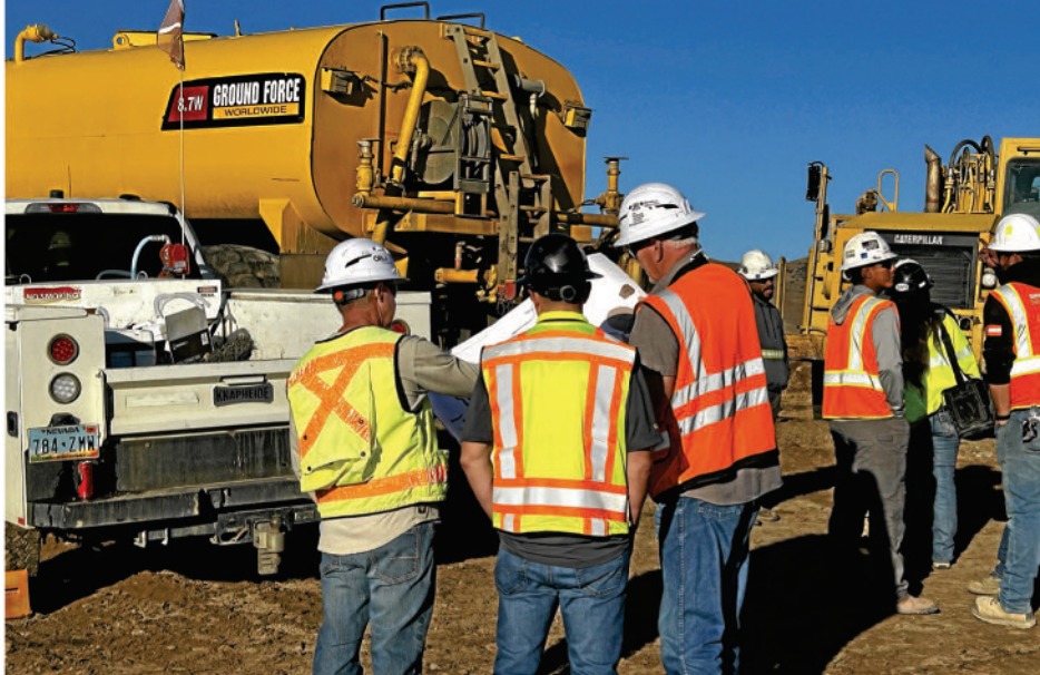
The U.S. Bureau of Land Management approved construction of the South Railroad Project in Elko County on Aug. 14, and on Aug. 15 Equinox Gold people were reviewing plans following a pre-start construction meeting.
