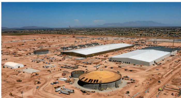
Construction of Meta Platforms' data center complex in far Northeast El Paso, Texas on July 23.
