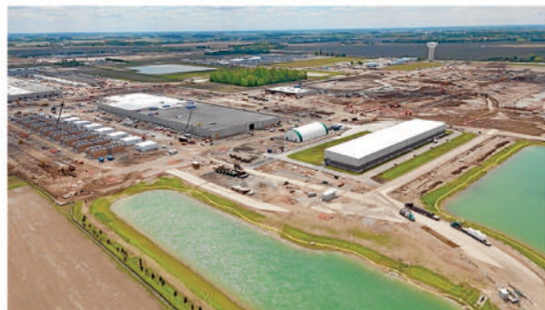
A drone view shows construction underway on Meta's new data center May 13 in Middleton Township, Ohio.
