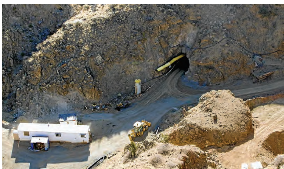
An underground portal at American Pacific's 100%-owned Madison Copper-Gold Project in southwest Montana.
