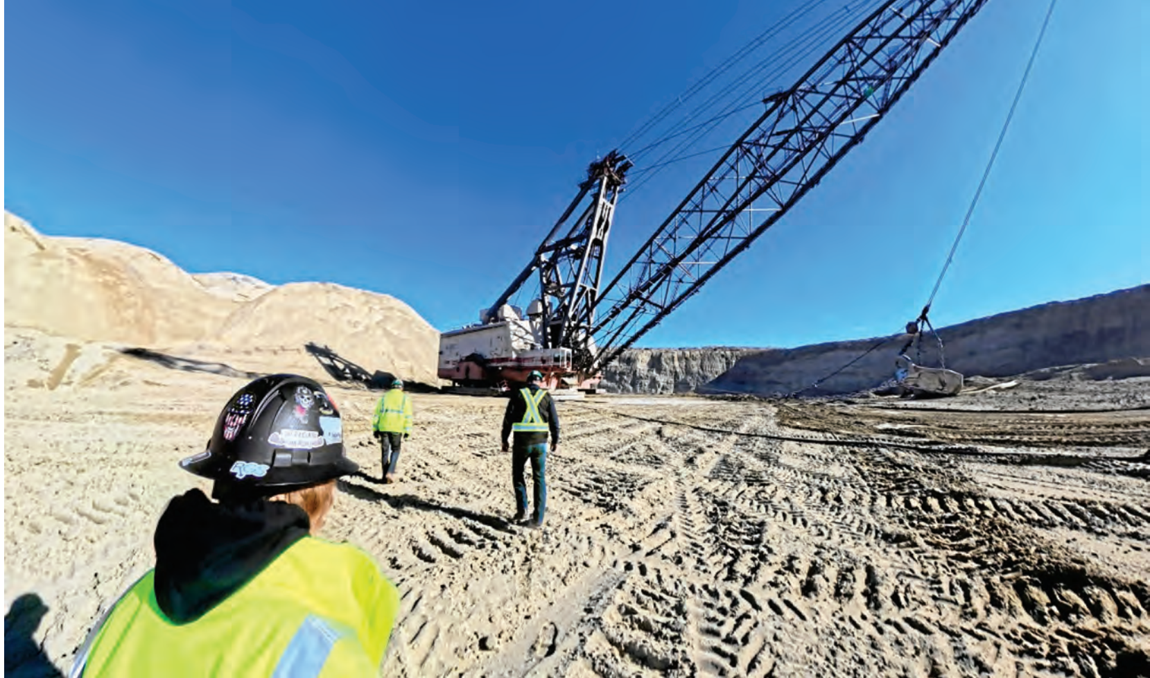
Walking to the dragline excavator during the interactive video tour of the Westmoreland Rosebud Mine.
