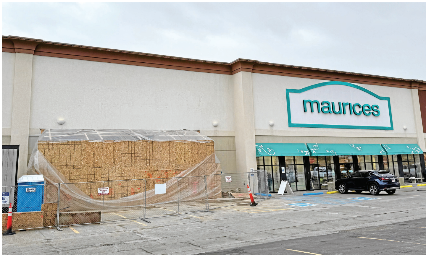
Elko VA Clinic under construction (to the left of Maurices) on Feb. 2, 2025.
