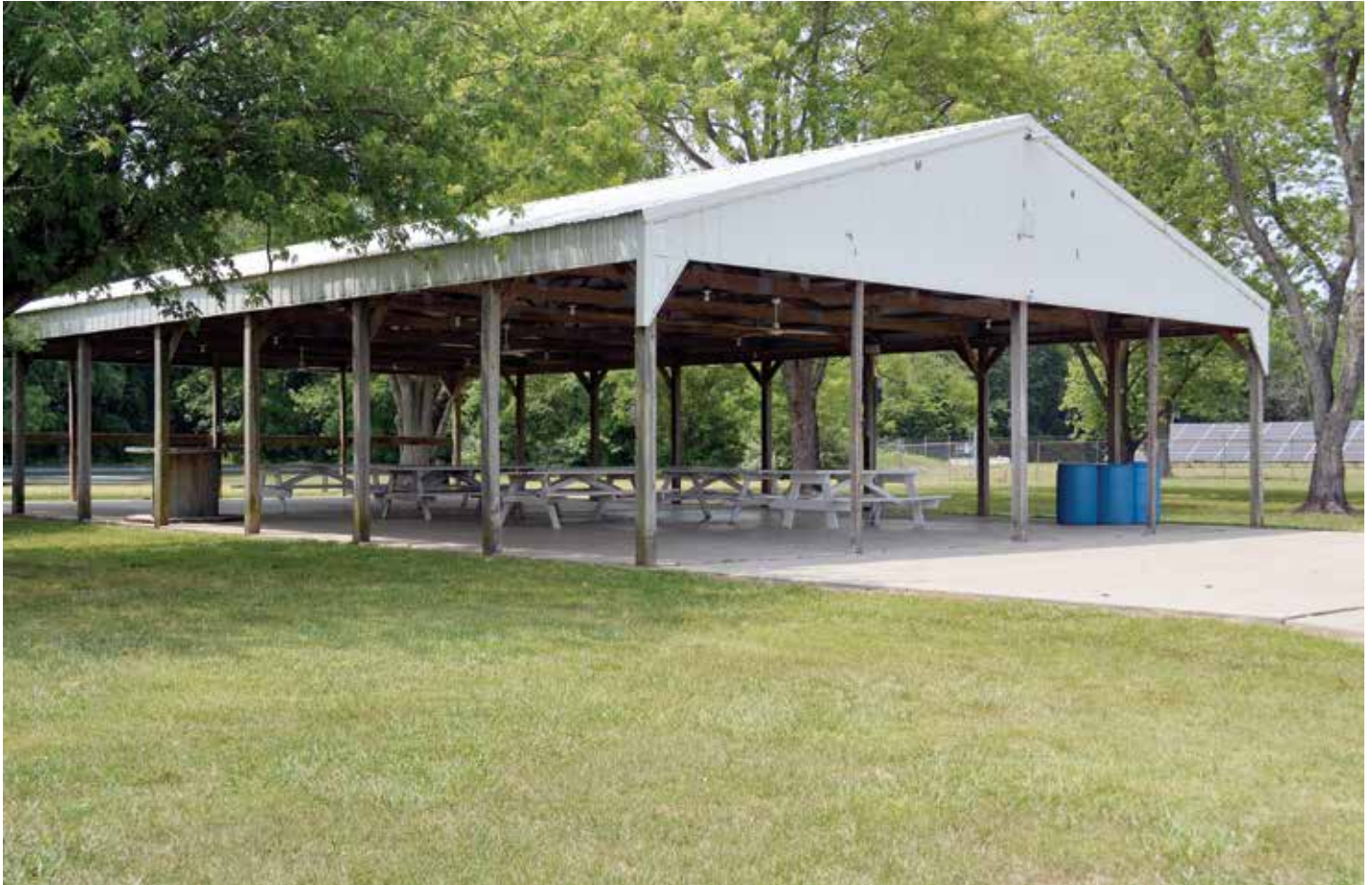
This pavilion in Montrose will get a makeover as part of a state parks grant the village received. Cathy Griffith photo.
