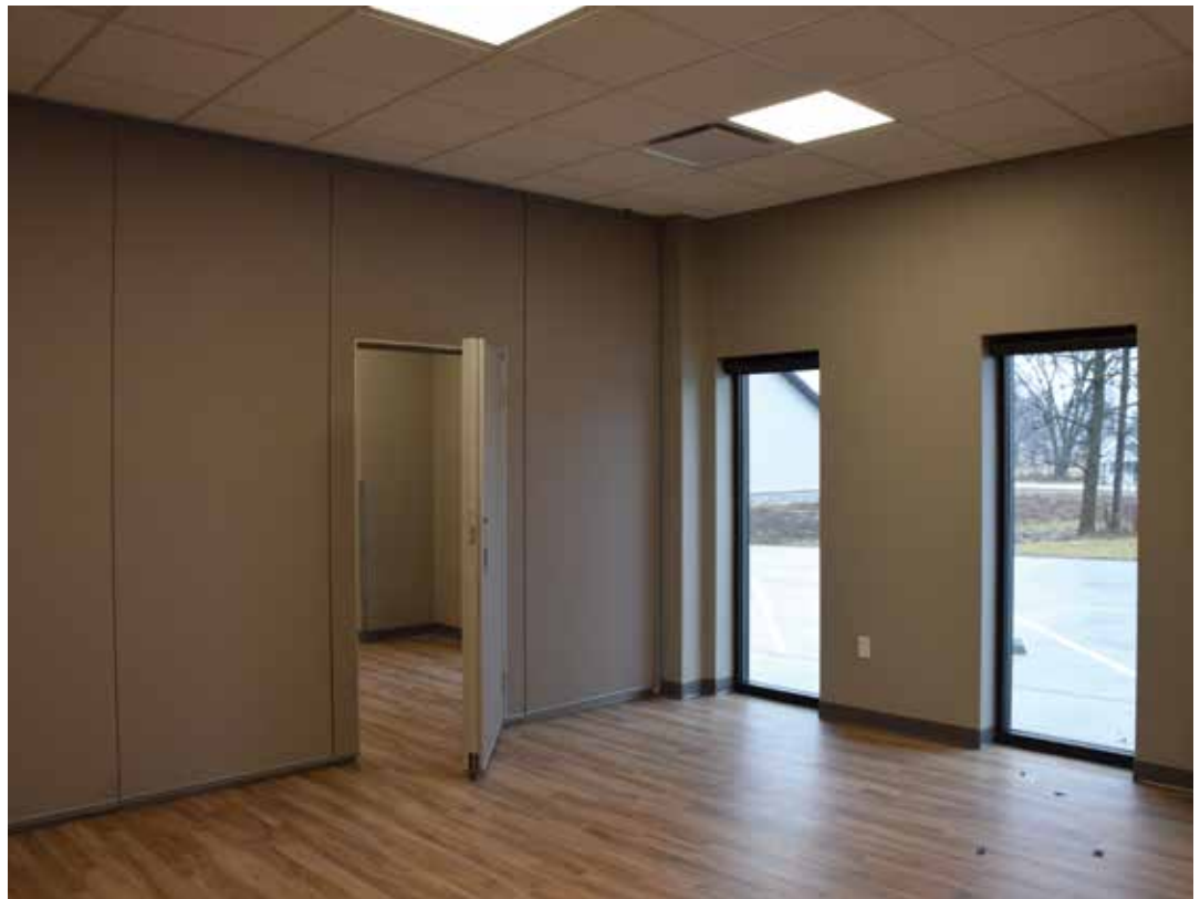
The community rooms inside the Wright Family Center have walls that can be opened up to make event spaces larger when needed.
