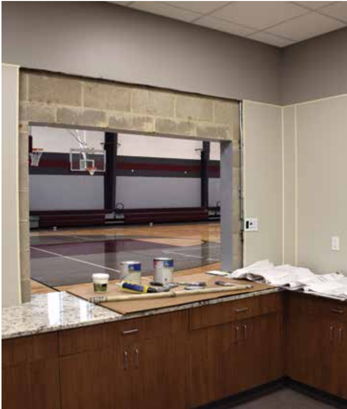
Construction on the Wright Family Center is nearly complete, but a few things, including the installation of a sliding metal window in the center's concession stand, still need to be finished before the new facility is ready for public use.
