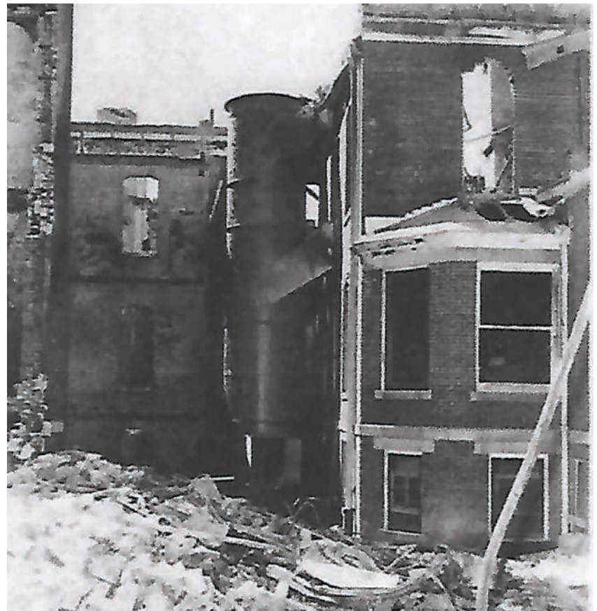
Tubular slide escapes were invented in the 1930s. St. Anthony Hospital installed them after an inspection and at the insistence of the state of Illinois around 1940. Shown is the unused slide escape after the fire. Submitted photo.
