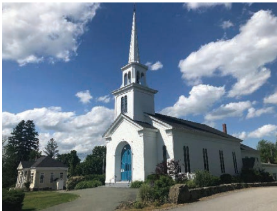
Hampstead Congregational Church, built in 1861.
