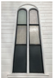
Detail of a pair of windows from the exterior showing.
