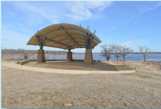
AMPHITHEATER SHELTER SHELTER IMAGE FROM POLIGON
