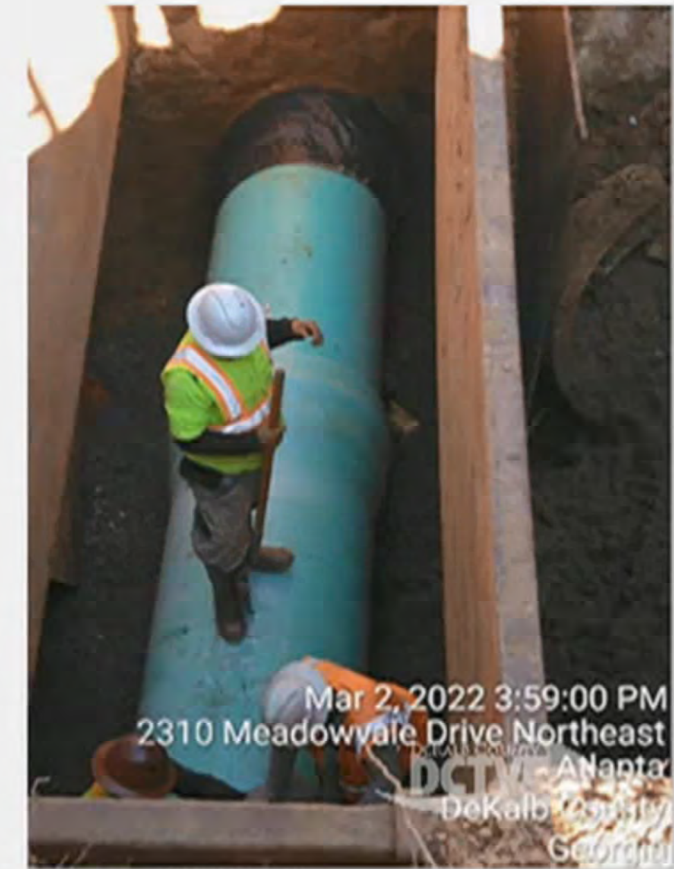
36" PVC Set in place
