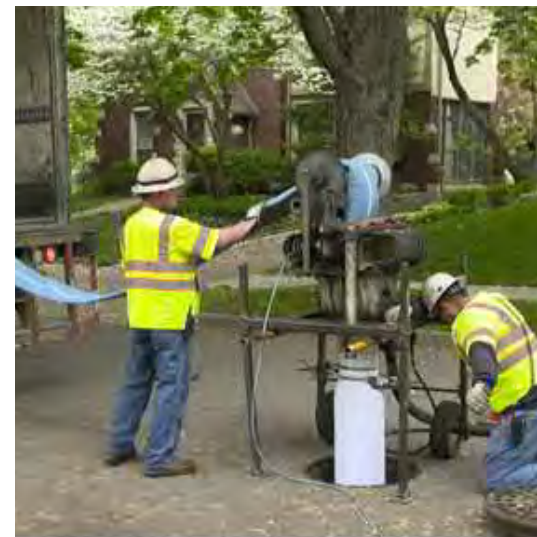
Rehab 133 miles of leaking pipes through trenchless technologies (where possible)
