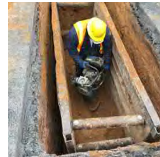
Perform 1,600 point repairs of localized pipe failures
