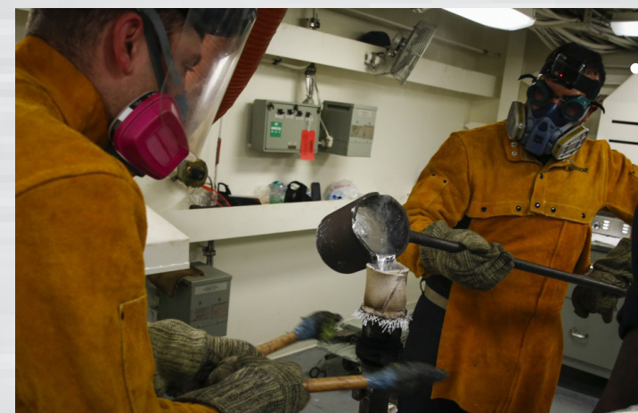
Zinc-poured socket terminal
