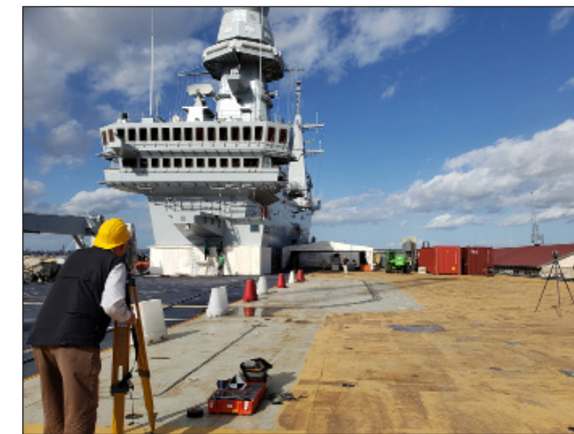
ATR surveyors use an optical transit and a laser scanner, which is on the tripod at far right. (U.S. Navy photo by Warren Kerr)
