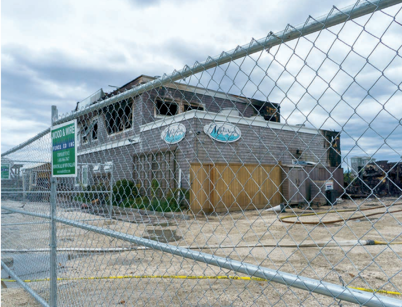
A chain link fence surrounds the fire damaged Matunuck Oyster Bar on Tuesday, May 20, 2025. Rhode Island Current photo by Laura Paton
