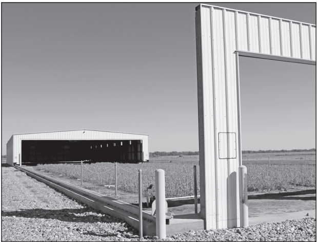
The rainout shelter at the Bayer Learning Center is a building on rails that automatically closes over crops when it senses rainfall. This ensures that plots receive only scheduled irrigation. This year's research under the shelter focuses on soybeans. (LOCAL Photo by Krystle Rhoades)
