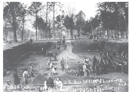
Excavation underway during the construction of the Florence, AL post office building in 1912
