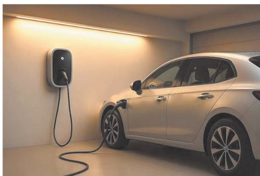
Installation of car chargers
