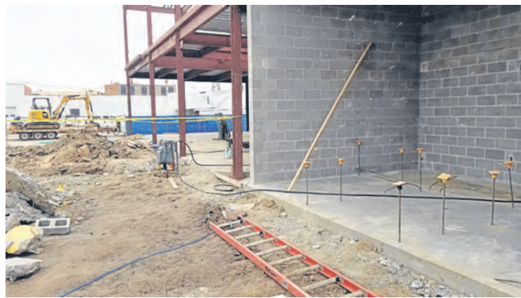
A view of where holding cells will be constructed at the site of the new Columbus Police Department. Just outside of the building, where the dirt can be seen, an exterior dog run will go in for CPD's K-9 unit.
