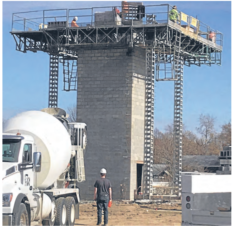
Construction workers were busy on a November 2018 afternoon with efforts on the new fire department located just north of U.S. Highway 81 between 46th and 47th avenues.
