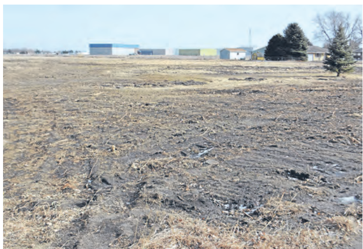
Land near Columbus Municipal Airport has been cleared so construction work can start on the Farmview Development, which calls for 24 multi-family units and 31 single-family units.
