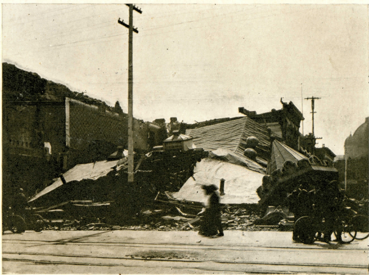
Elks' Hall, West Santa Clara St., San Jose, Cal., after the Earthquake, April 18, 1906.
