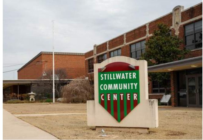
Stillwater Community Center
