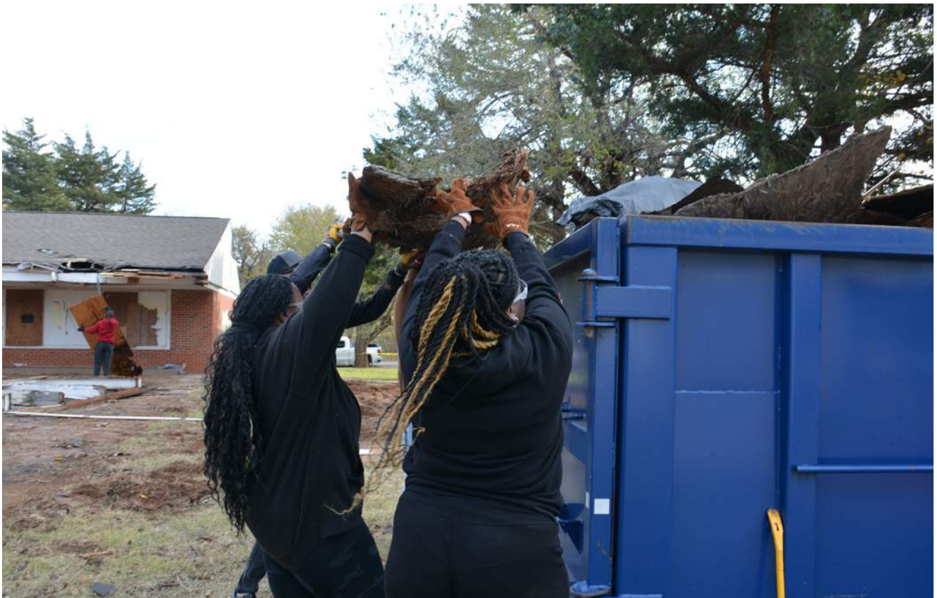
Washington school renovation, community volunteers.
