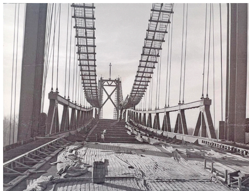
Construction sometime between 1954 and 1956.
