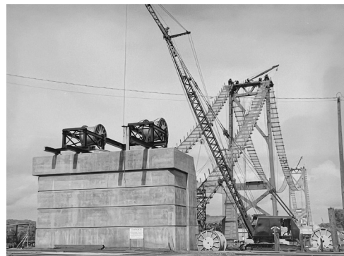
A reinforced concrete anchorage, at left, is ready for the cables that will be stretched across The Gateway Bridge's two towers in this Clinton Herald photo from between 1954 and 1956.
