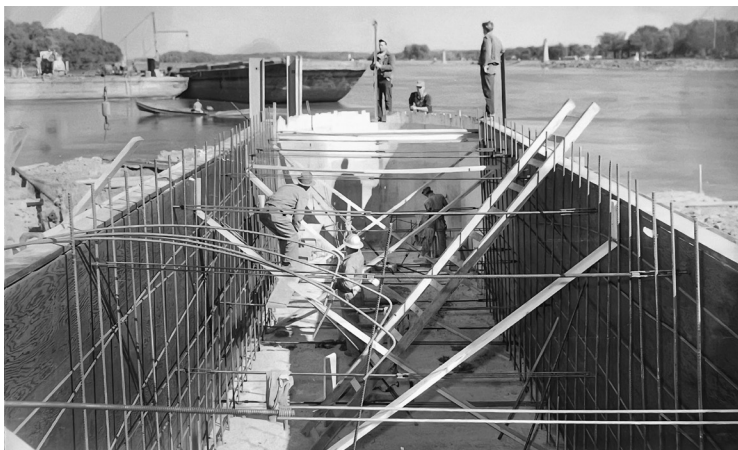
A crew constructs of a pier form for the Gateway Bridge.
