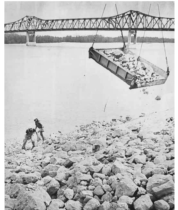
A crane drops rocks on the riverside of the new levee in 1977.
