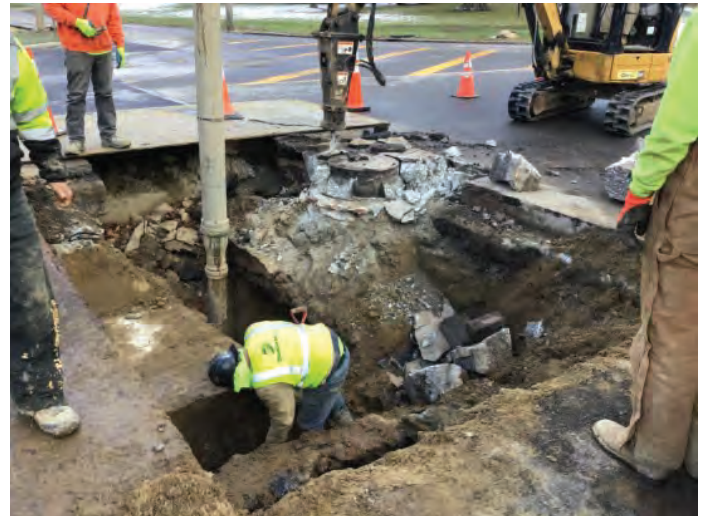
Culvert work using Hydro-Vacuum Truck and Excavated below Shaker Blvd in the roundabout
