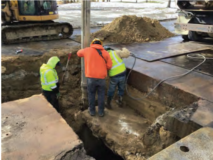
Culvert work using Hydro-Vacuum Truck for excavated
