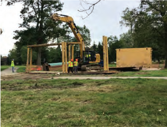
DRS putting together a trench box.
