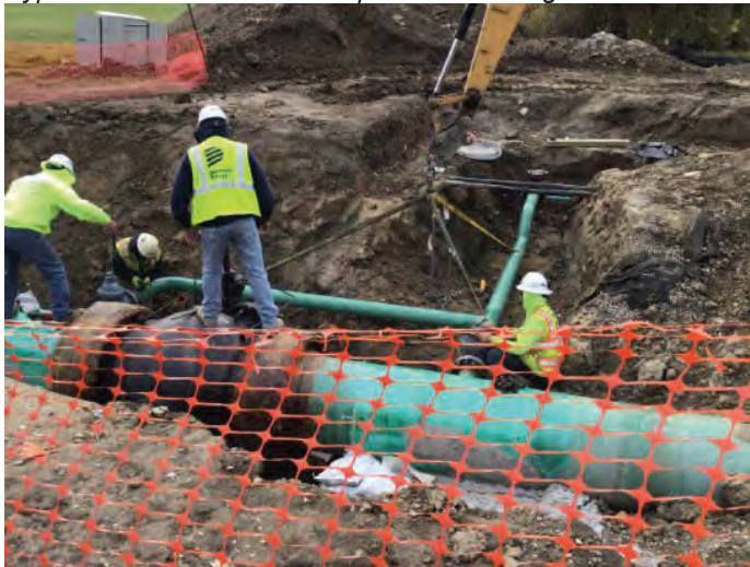
Bypass connection work last pieces for new gas service
