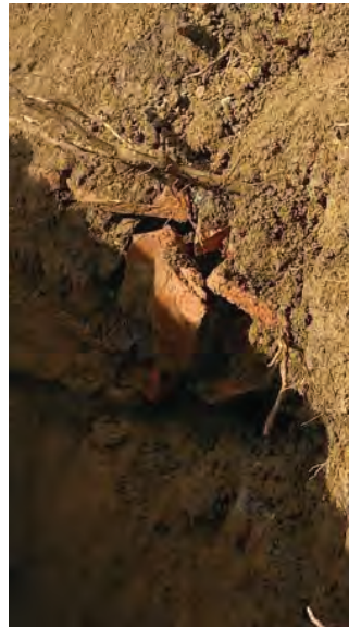
Previously broken storm drain from daylight to curb drain on Brainard.
