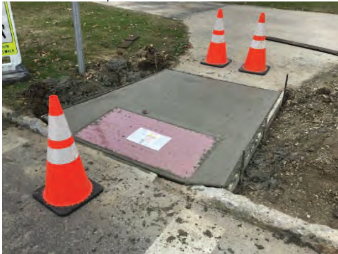
Curb Concrete ramp
