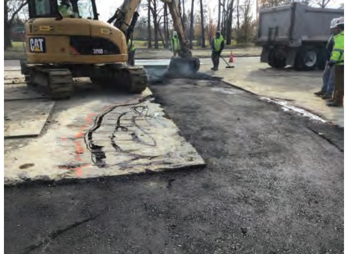
Work on the asphalt add second layer
