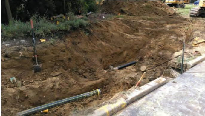
Trench that was enlarged so that crew can figure out how to tie 4 inch in.
