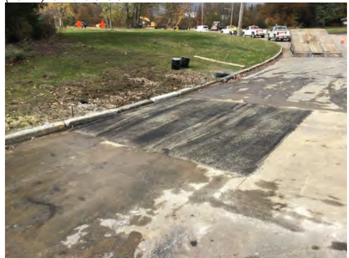
Asphalt work in front of Shaker BLVD East near the curb (10*12) ft in the circle
