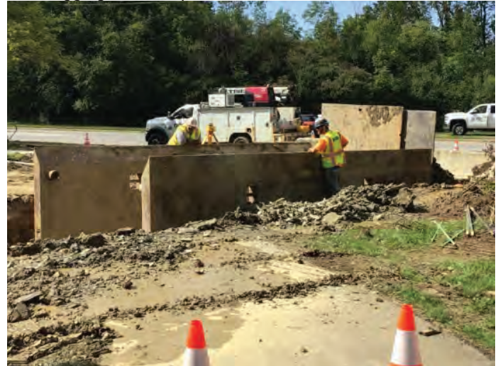
DRS digging the bore pit.
