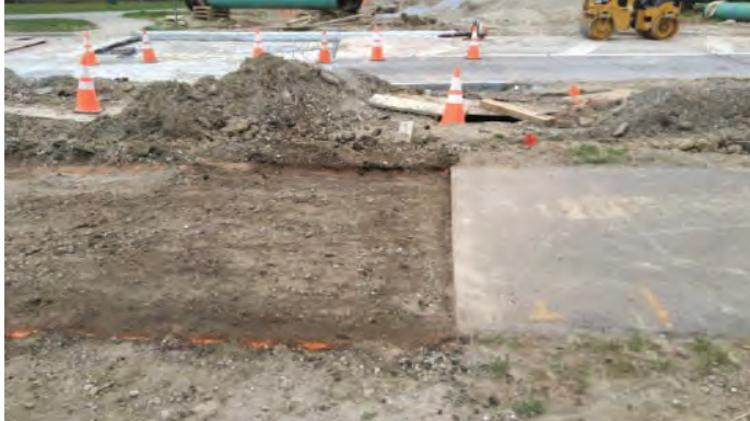
Bike path clear out ready for asphalt
