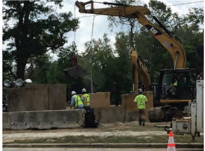
DRS removing the spoils from the bore pit.
