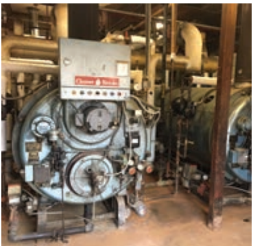
Courtesy photos from South Lane School District Facilities Director Matt Allen The two original boilers at Lincoln Middle School were designed to last 25 years and District Maintenance Staff have kept them running for 63 years.
