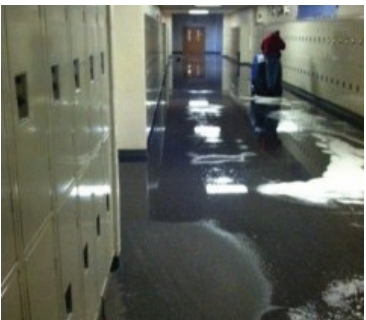
Courtesy from South Lane School District Facilities Director Matt Allen It was all hands-on deck for the district facilities team to clean flooded hallways at Cottage Grove High School after several junctions in the fire suppression system failed during multiple days of single digit temperatures in 2013.
