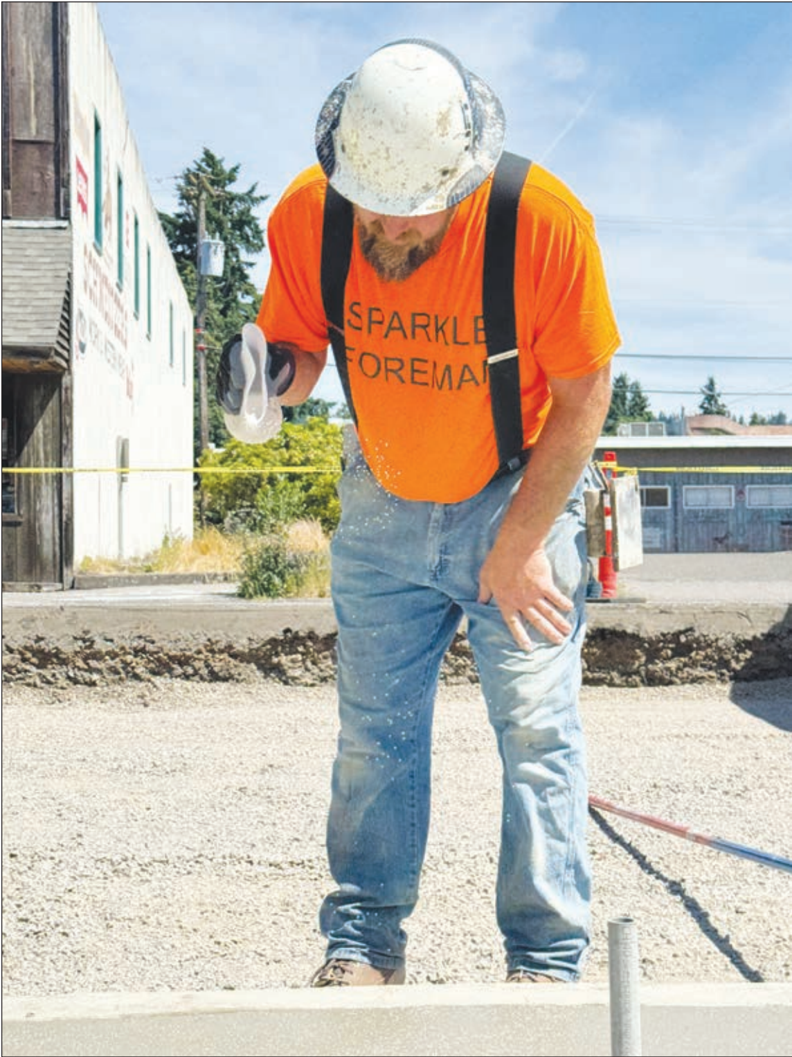
Courtesy photo from Dana Merryday The Wildish “Sparkle Sidewalk” foreman takes aim and sprinkles the sparkle material onto the walkway along Cottage Grove’s Main Street.
