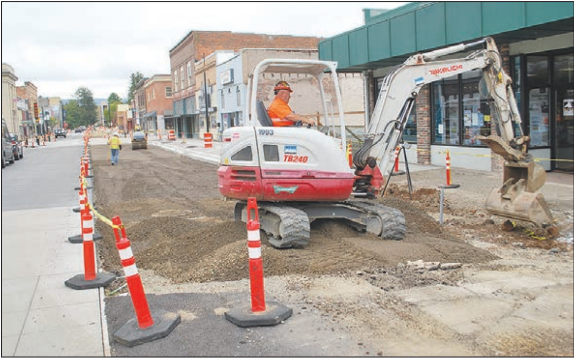
Wildish crews continue working on the Main Street Revitalization Project in Cottage Grove's Historic District.
