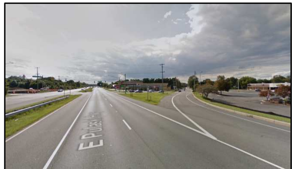
The Delaware Avenue slip lane on Route 40, facing west.
