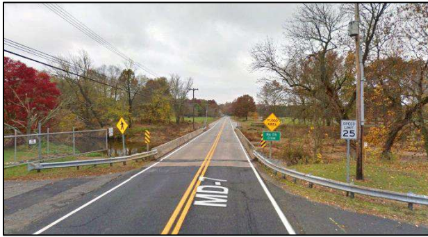
The Delaware Avenue bridge over the Big Elk Creek.
