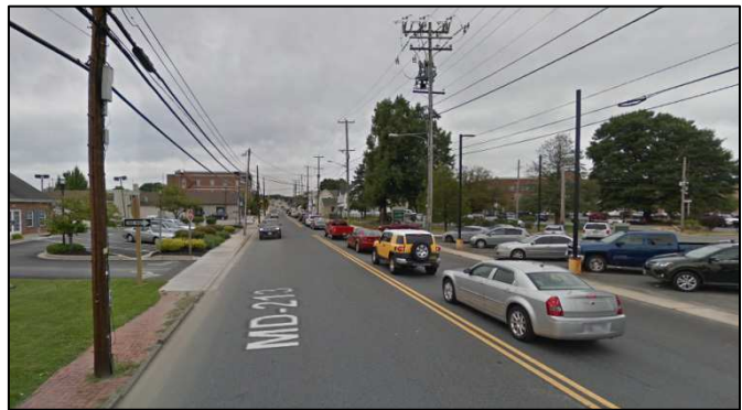
Bridge Street between Main and Cathedral Streets, looking north.
