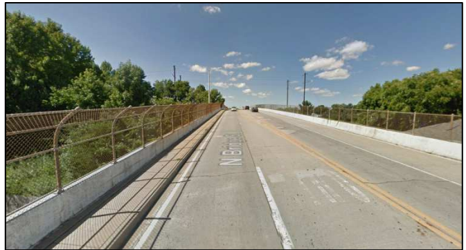
Bridge Street crossing over the railroad tracks, looking north.
