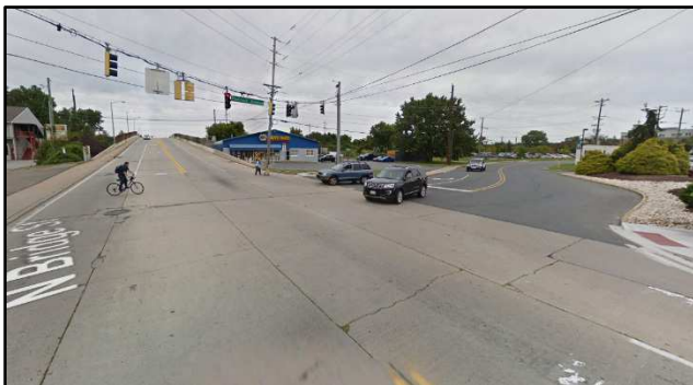
Bridge Street and Railroad Avenue, looking northeast.
