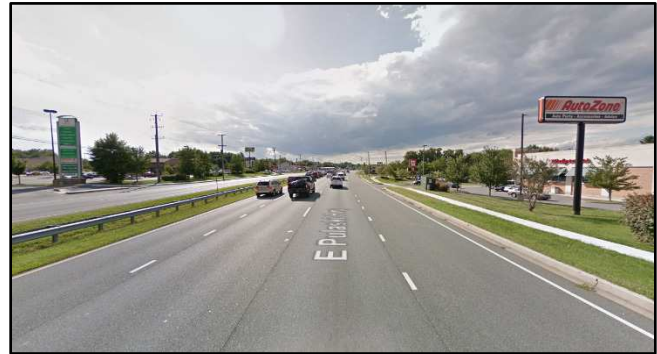
Route 40, facing west, near Whitehall Road.
