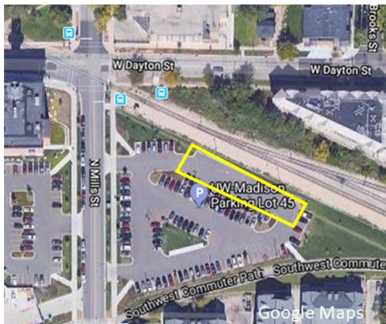
Figure 3.0-3 Charter Street Heating Plant
