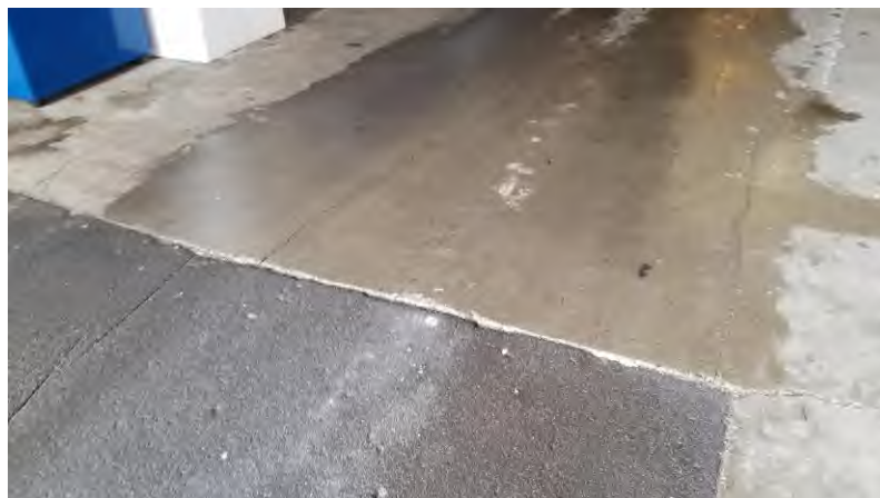
100 Level Concourse: Concourse floor surfaces present numerous cracks and uneven shifting slab edges.
