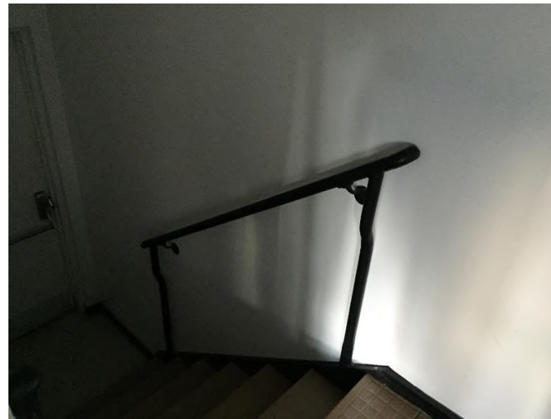
300 Level Admin – Injured Player Area: Railings to a means of egress are not code compliant. Lighting was out or off and no signage leading to the spaces was limited and or visually blocked.
