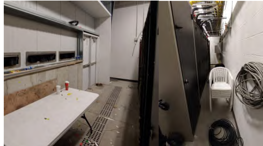
Figure 12&13- Broadcast interconnect headend racks and clearances.
