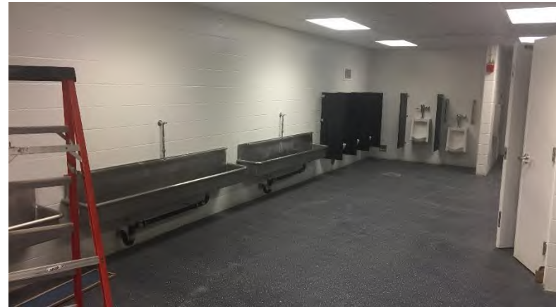
100 and 300 level Concourse Restrooms: Wide use of urinal troughs.
