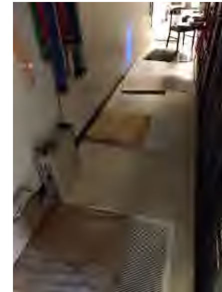
Figure 8- Production headend racks. Plywood covering diffusers to direct and/or balance airflow through racks.
