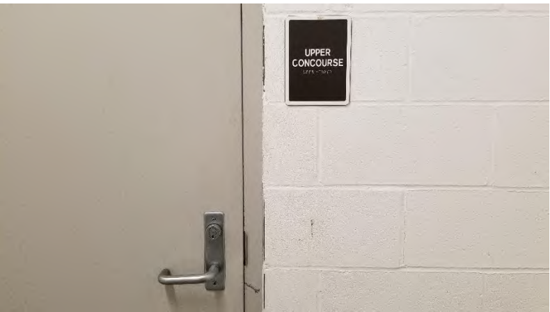
Elevator Lobby 331.05: Lockset is damaged and cannot be opened from within the Lobby.
