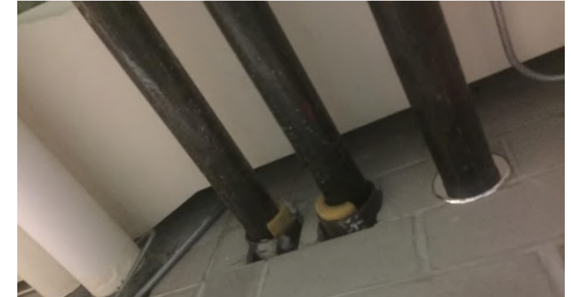
Mechanical 209.09: Many block penetrations throughout all concourses and mechanical rooms are not properly sealed.
