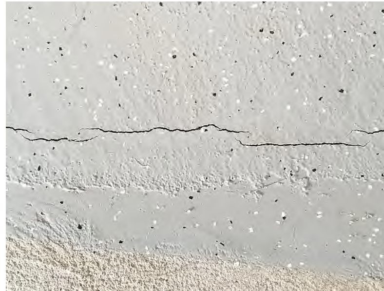
100 Level Suite Alcoves: Floor joints below traffic coatings have failed in many locations.
