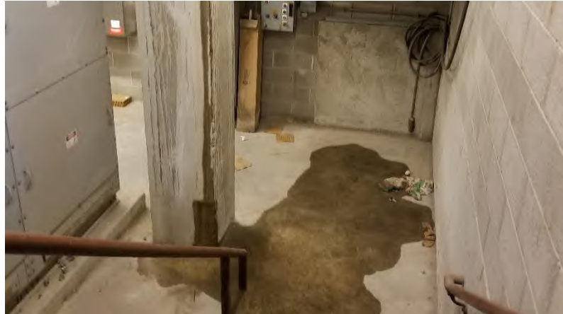
Electrical 101.03: Water leak from seating bowl above.
