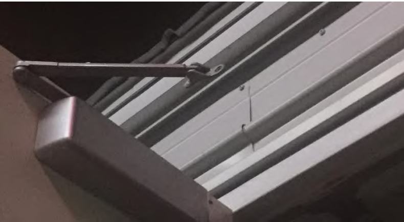
West End Camera Booths: Door closer broken.
