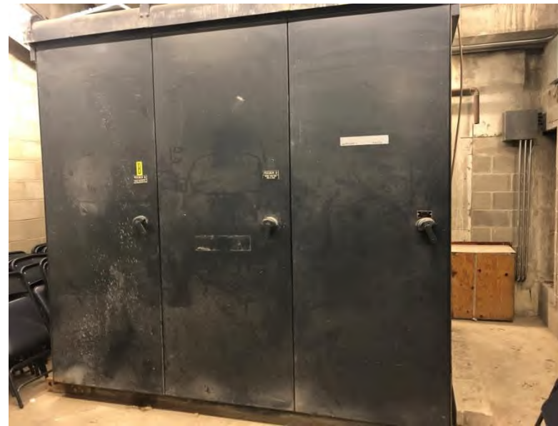
1972 15kV Main Switchgear on Feeders B & D
