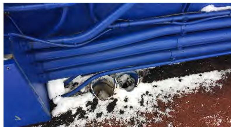
South Sideline: Number of abandoned raceways not properly capped.
