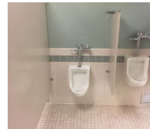
Urinals: Required grab bars are often missing at urinals.
