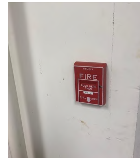
Fire Alarm Pull Station – Installed in 2014
