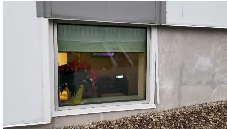
West Wall: Damaged metal siding trim around window.
