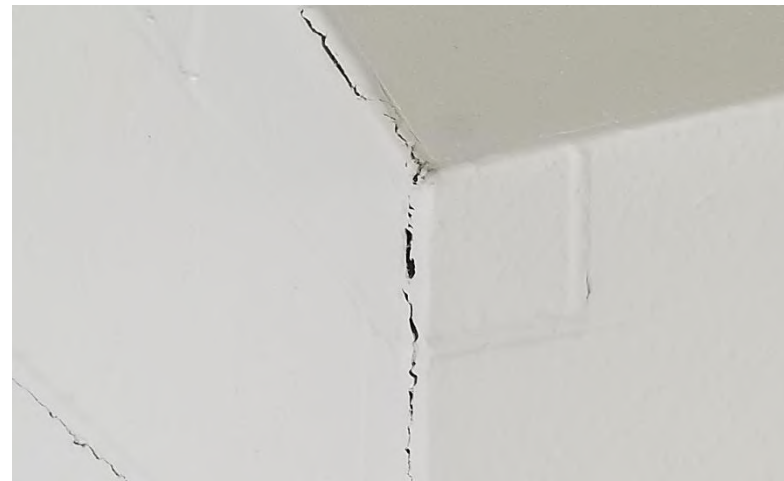
Drying Area 021.24: Movement between structure and masonry walls.
