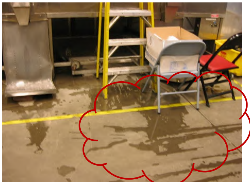
Drain water at ice plant running across floor.
