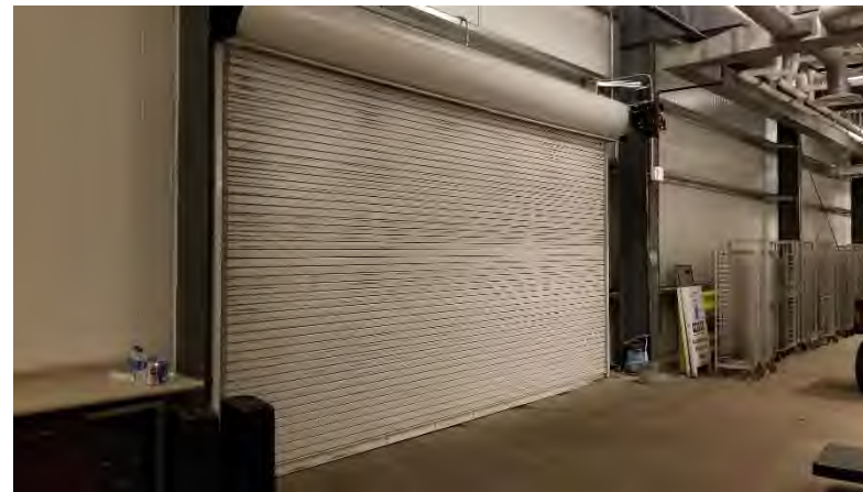
Rear Overhead Door: DNC reports that this door sags and sticks, and is difficult to operate.
