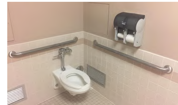
Waterclosets: Vertical grab bars are often missing at accessible stalls.
