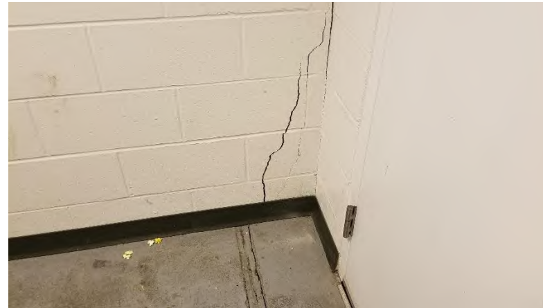
Concession 332.03: Walls were built over a building expansion joints at gridlines 19, 26, 63, and 70 resulting in failed floor joints and cracked partitions.
