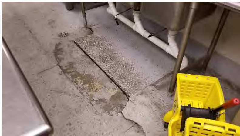
100 Level Typical Concessions / Pantries: Uneven floor surfaces hold liquids and do not slope to a drain.
