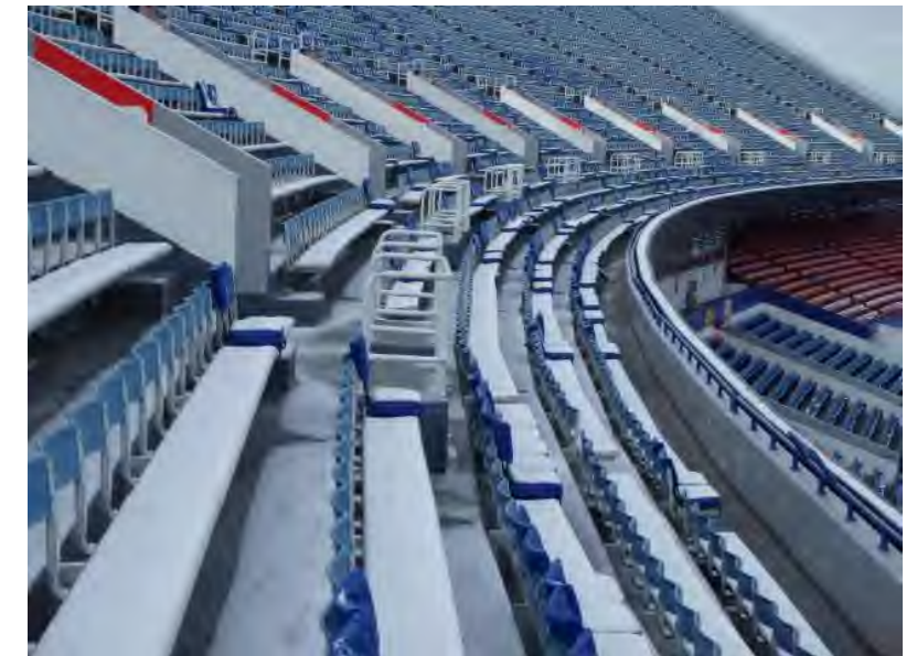
Typical Upper Level Seating Area: Lower 11 rows are waterproofed with urethane membrane in fair condition.
