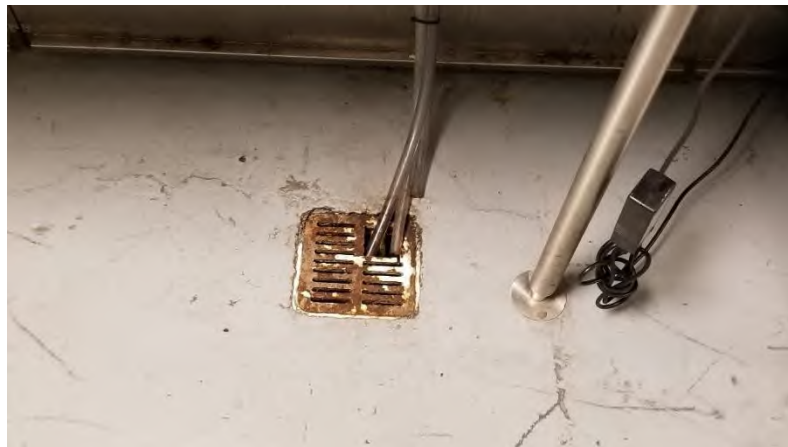
Floor sink finish corroded. Typical of many concessions.
