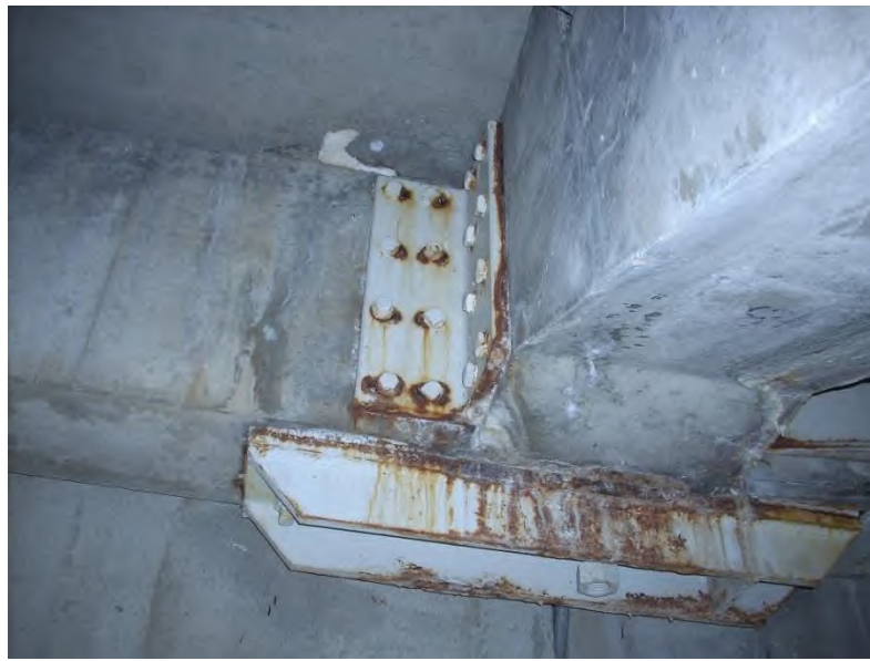
East End Zone Frame: Typical expansion joint assembly – Teflon pads require periodic maintenance.
