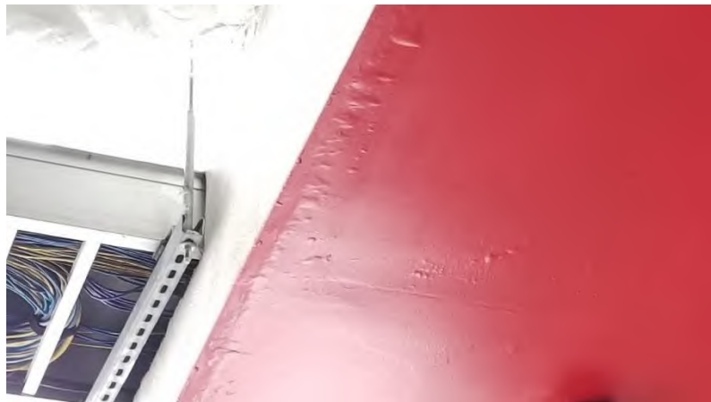
100 Level Concourse: Soffit near gridline 77 exhibits minor water intrusion from above.
