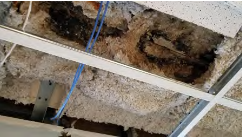
Dugout Suites: Water leaking into the Suites through the seating bowl damages spray thermal insulation and ceilings.
