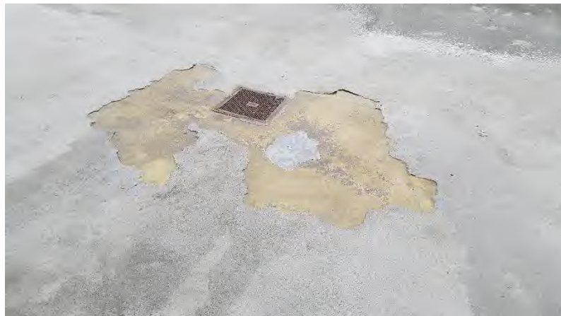
300 Level Concourse: Typical coating damage at concourse drains. Edges of drains are where coating edges are easily attacked.
