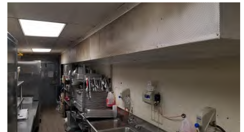
200 Level Kitchens: Ventilation screens added in 2014 collect dirt and grease.
