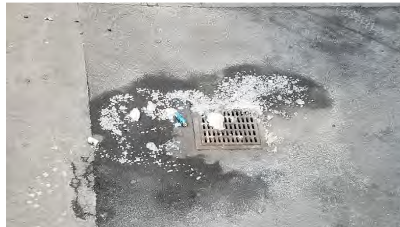
100 Level Concourse: Area drains are frequently used as ice dumps, causing icy areas (depending upon time of use).
