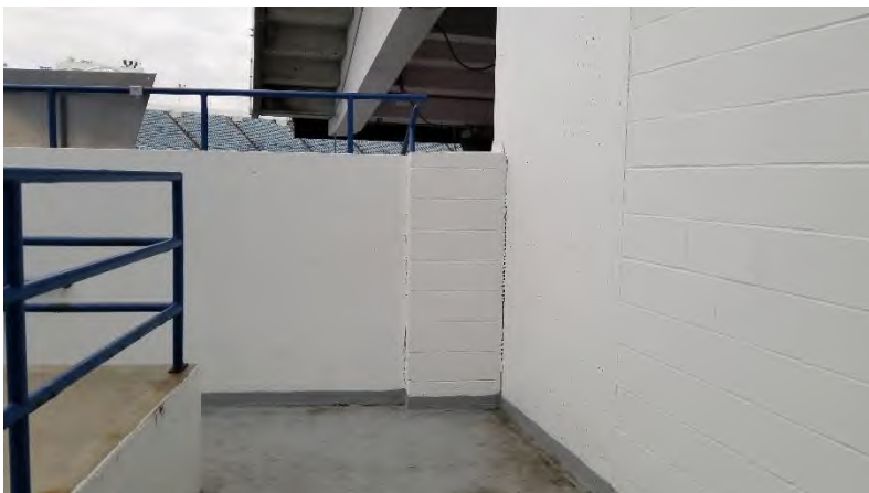
Ramp Landings: Expansion joints were not established through walls at Grids 12, 33, 56, and 77, leading to cracks in the corner shown and water intrusion in the spaces below.
