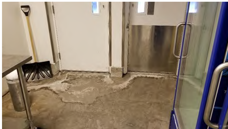
300 Level Concessions and Vendors: Water enters space at door thresholds. Slabs outside slope toward door.
