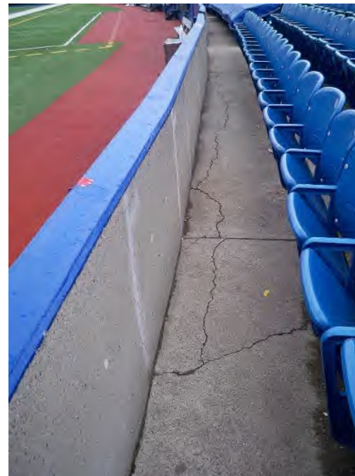
Lower Ringwall: Rotation of ringwall toward field with cracking of front row of on-grade seating slab.
