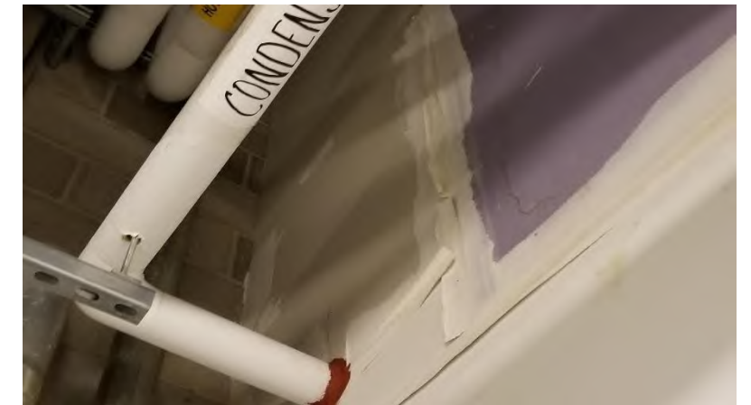
Corridor 023.19: Water damage overhead to drywall partition.
