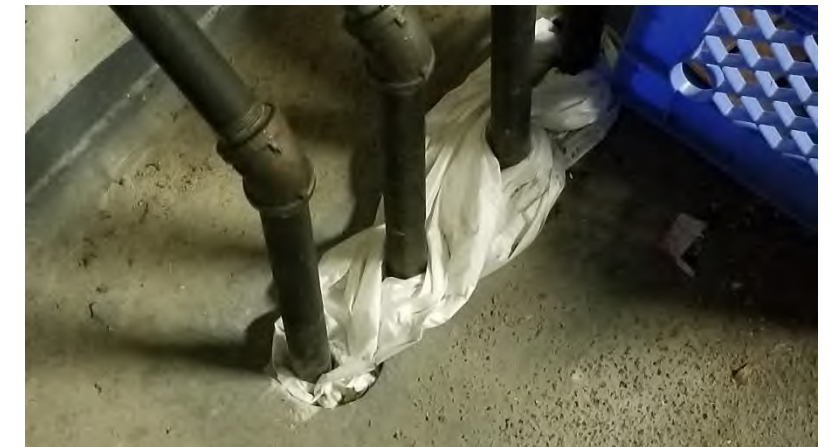
Electrical 122.04 : Floor penetrations not sealed with fire caulk. Building Code.
