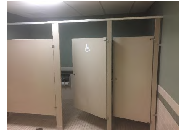
Accessible Stalls: Doors at accessible stalls often swing in the wrong direction.
