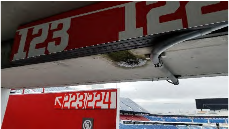
100 Level Vomitories: Ponding water above is often drained with holes drilled through front row treads. Water drips and causes ice.
