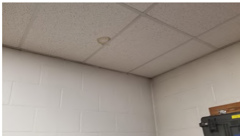
Official's Locker 023.28: Water damage at ceiling.
