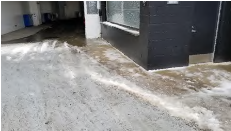
100 Level East End Concourse: Expansion joints in concourse floor frequently leak into 000 Field Level spaces below at grid lines 41 and 48.
