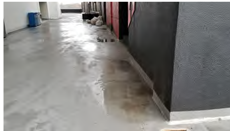
300 Level Concourses: In front of each Tower, water ponds between doorways at restrooms and elevators.
