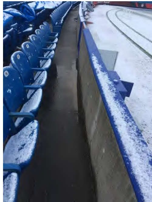
First Row: Water/ice buildup on first row. Some field wall drainage issues with proper sloping to scuppers. Substantial ponding on 2 row on North Sideline.
