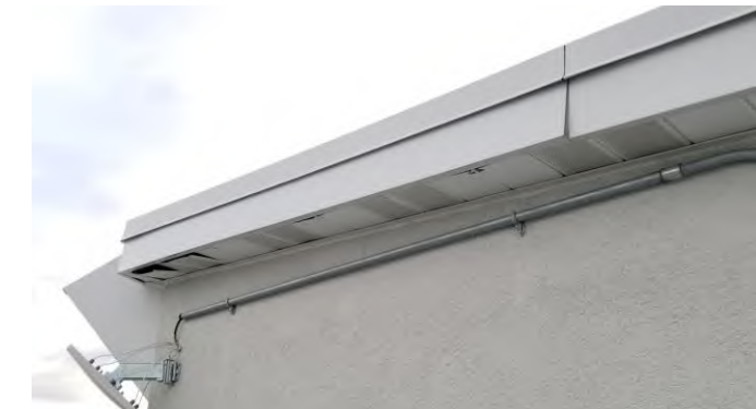
400 Level South Camera Booth: Metal soffit and fascia is damaged, perhaps from high intensity winds.
