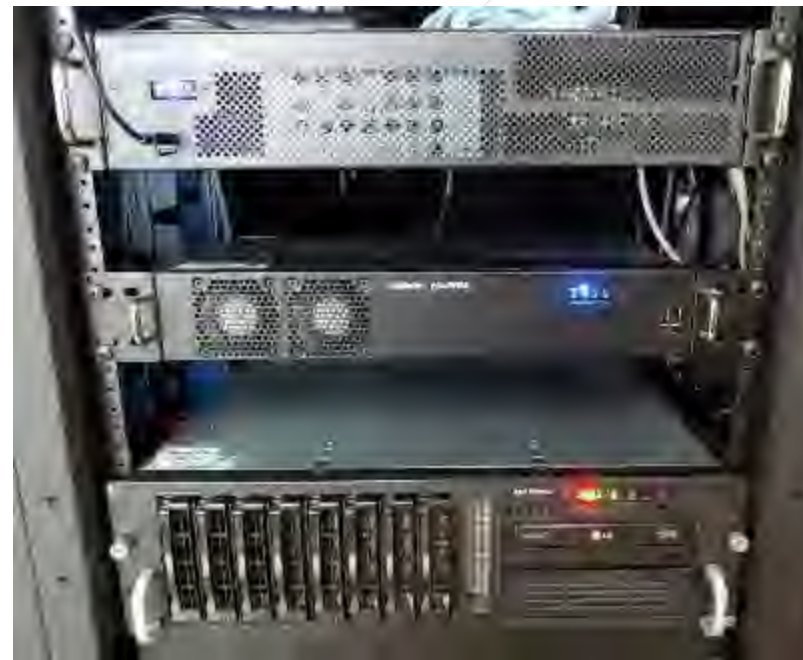
Figure 18- Harris IPTV/Signage system headend, servers and storage array.
