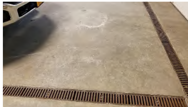
Vehicle Bay 2: Wash-down floor does not slope to drains.
