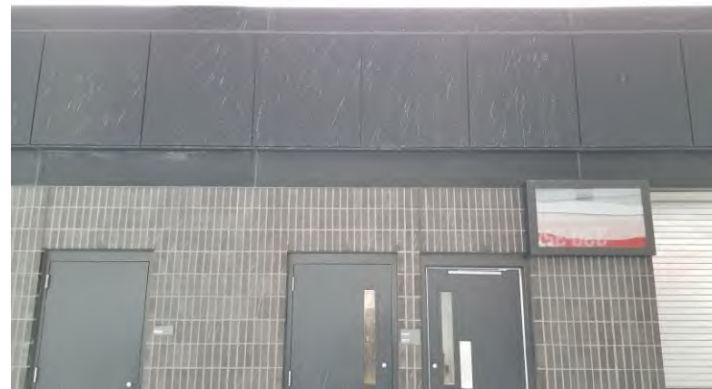
Upper Deck Exteriors: Overspray from salt brine applications often end up coating the exterior walls and roofs below.
