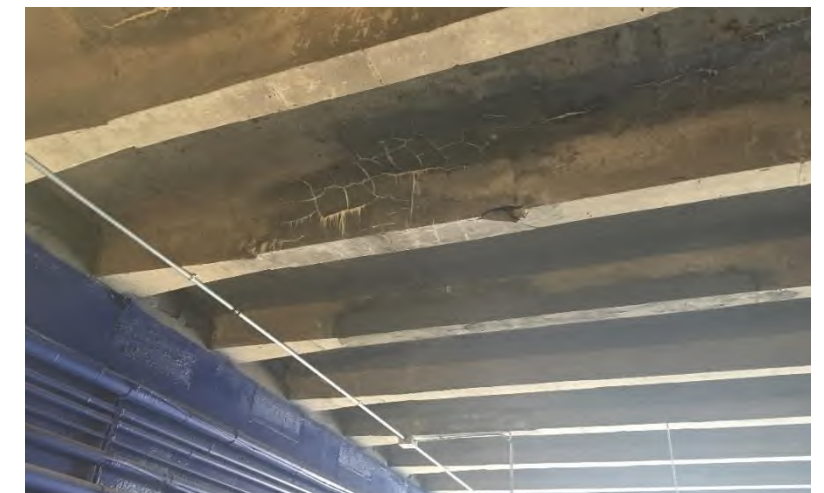
Field Access Tunnel: Extensive repairs to field tunnel access under perimeter roadway.
