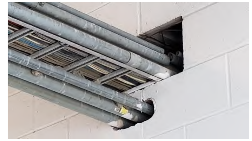
100 Level Vomitories: Many wall penetrations through vomitory walls are not closed. Raceway allows raccoons into building.
