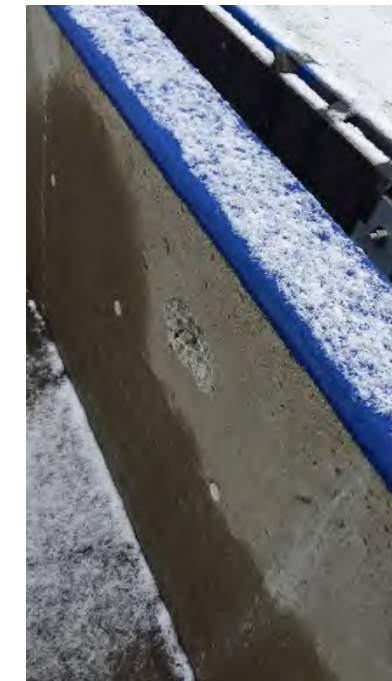
First Row – Section 102: Concrete spalling.
