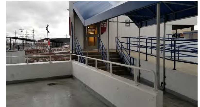
200 Level Ramp & Stair Landings: Slabs are uneven and do not slope to drains. Typical at all four corners of stadium.
