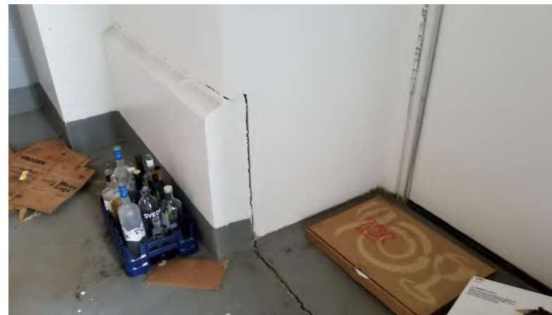
300 Level End Zone Stair: An expansion joint has not been established along gridline 56, between the Concourse structure and the End Zone Tower added in 1999. The sealant joint has failed with minor water intrusion below. The potential for similar damage to occur exists at grid line 33.
