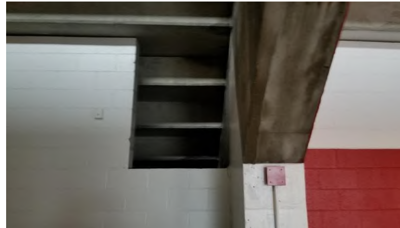
300 Level Concourse: Missing grille near Gridline 19.
