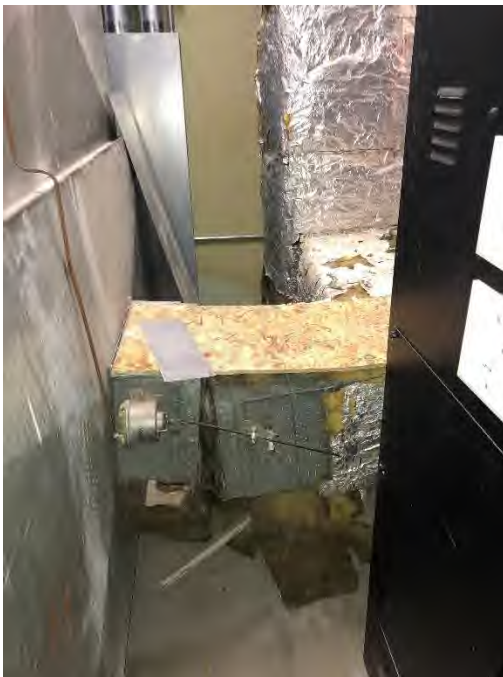
Outside air intake damper disabled and lacking economizer capability.
