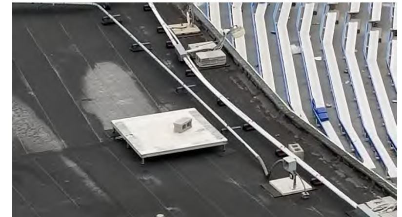
West End Camera Platforms: D-ring tie-offs are provided, but remain unused. May need protective railings. Building Code.
