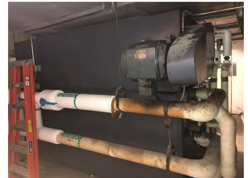
1972 AHU in need of replacement. Typical of 3.
