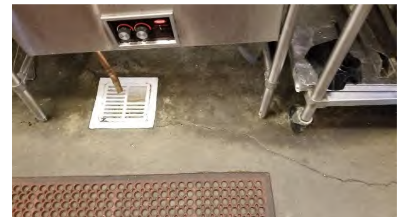
Slab-on-Grade Cracking: Shrinkage cracks have carried through food preparation areas. Joints should be sealed.
