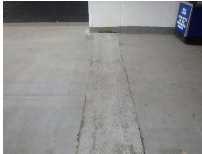
300 Level Concourse: Typical expansion joints with coated metal covers throughout the 300 Level Concourse.
