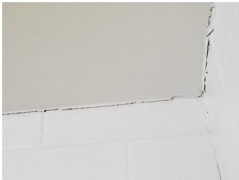
Field Level Drywall Ceilings: Joints between ceilings and walls have failed in several areas at the Field Level indicating movement in the adjacent structure.
