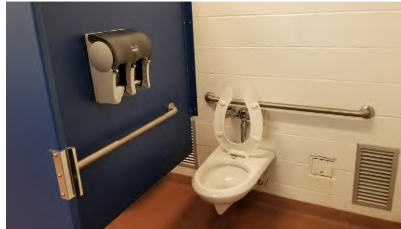
Stalls: Many of the accessible stalls in older restrooms do not have accessories configured in an accessible location.
