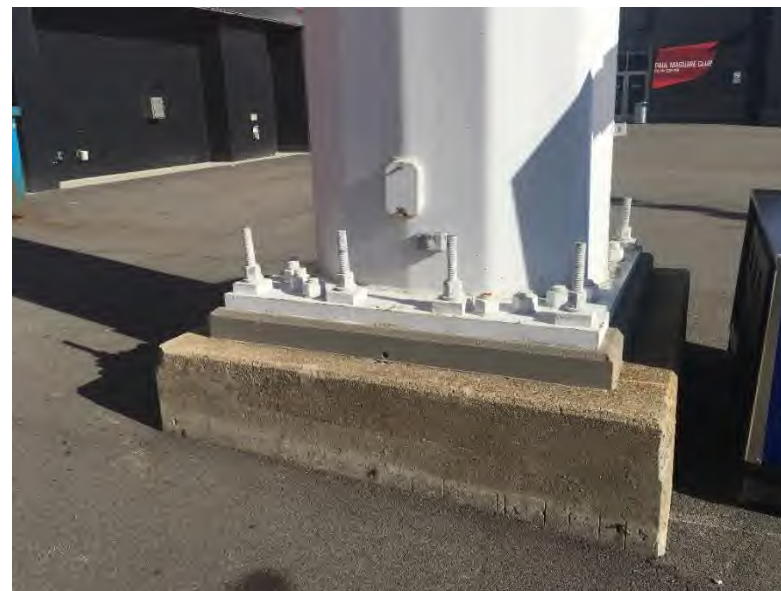
Typical Field Light Tower: Retrofit post-tensioned anchorage of light tower bases.
