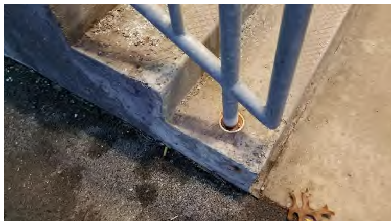
Dock Area: Concrete deterioration at base of exterior stair.
