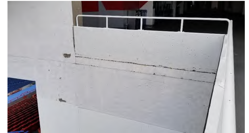
300 Level Concourse: Movement in walls adjacent to Gridline 77 is evidenced by cracks and spalling. The ramp wall in the foreground is effectively pulling on the wall exhibiting cracks because there is no expansion joint provided in the corner. The potential for similar conditions to develop exists at grid lines 12, 33, and 56.
