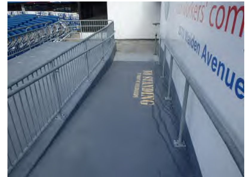
Lower Bowl Seating Area: Urethane membrane coating over accessible ramp to Lower Seating area. This area is over occupied space.
