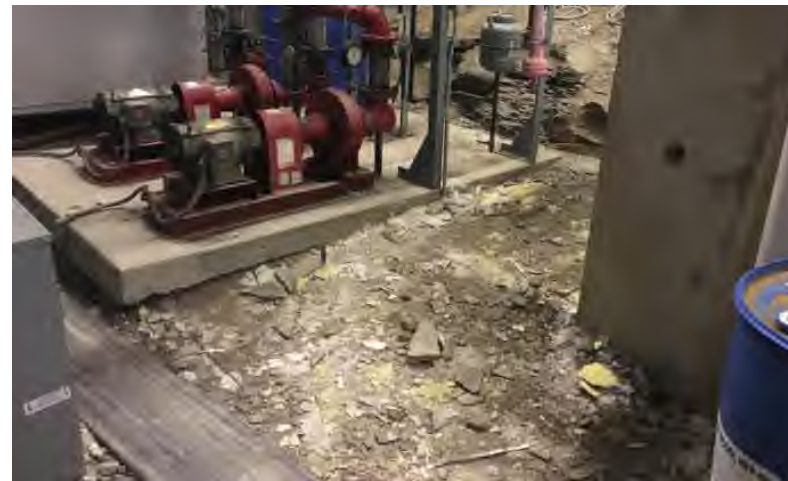
Corner MEP Spaces: Spaces still have dirt floors (exposed shale).
