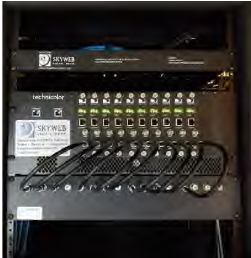
Figure 16- DTV satellite service provider interface
