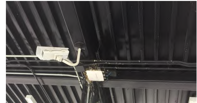
Gate 2: Birds roosting on/above newly installed camera, WAPs and pull box locations.
