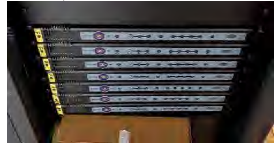
Figure 18- CATV QAM modulators
