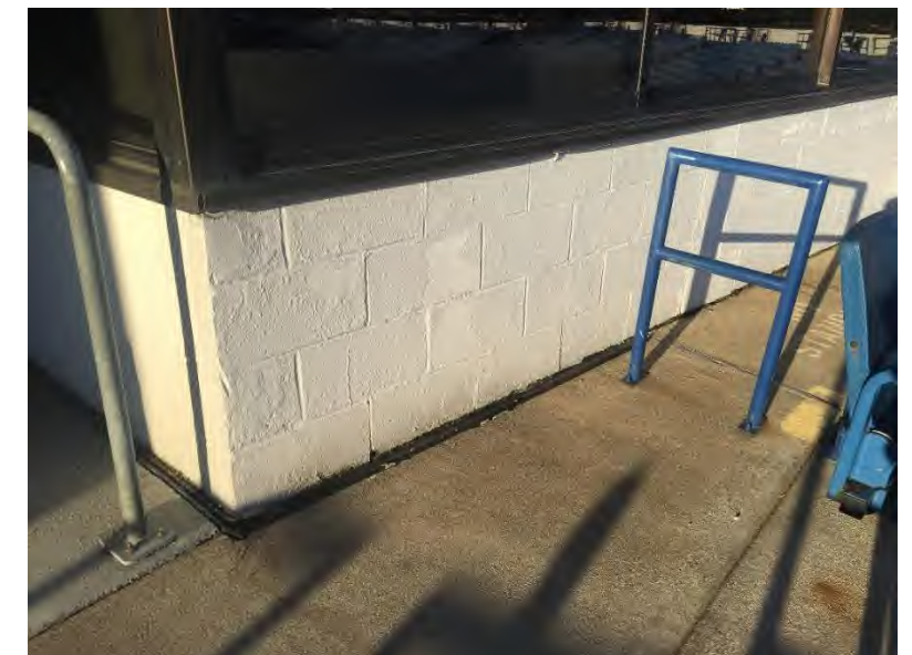
Lower Bowl – West Endzone: Endzone expansion joint along dugout suite and general condition of on-grade seating slab.
