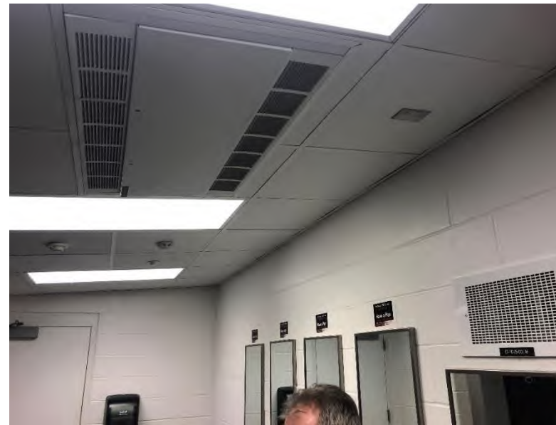
Typical restroom ceiling with cabinet heater and wall cavity fan.
