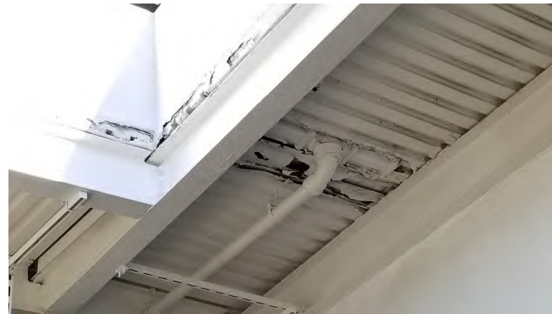
West End Ramps: Underside of ramps exhibit rusting steel and peeling paint.
