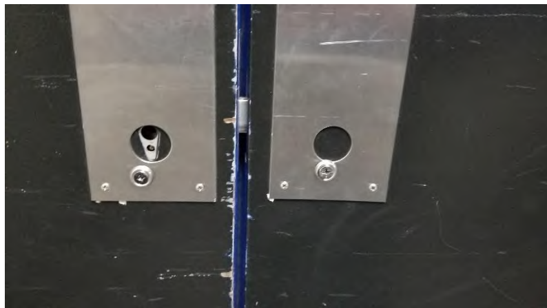
Visitor's Locker Room 023.31: Exit doors are locked from the corridor side and do not function if locked while occupied.
