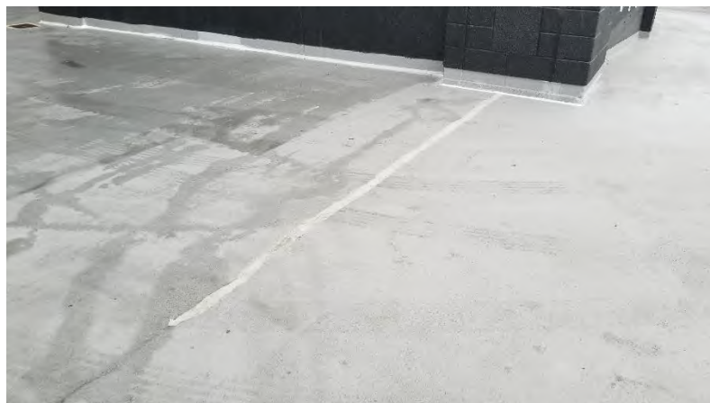
300 Level Ramp Landing: Joints in the slab have opened up and been sealed. Joints occur above enclosed space. Sealants fail.
