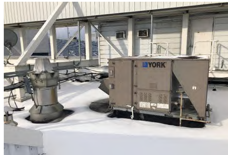
Typical of newer RTUs recently installed.
