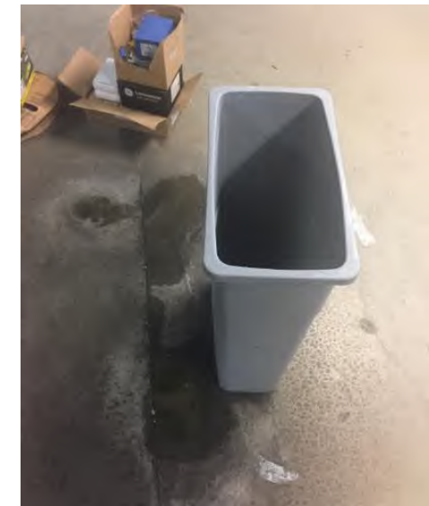
Mech 237.06: Trash can positioned to catch water from roof leak.
