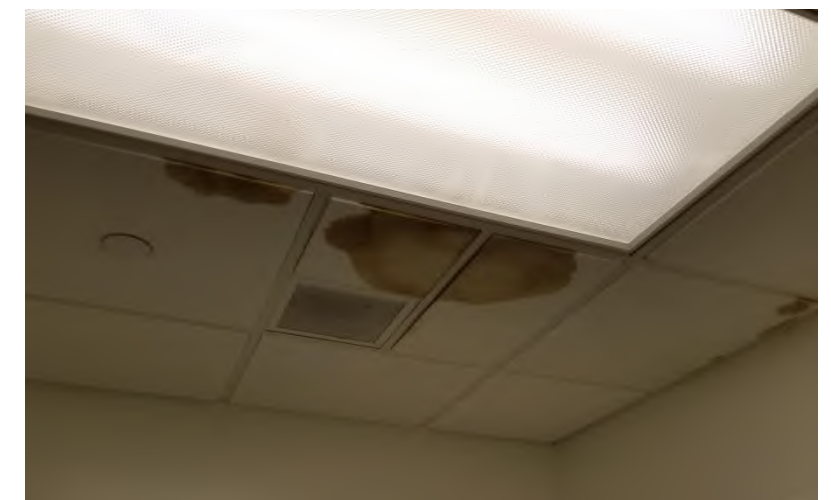
Chain Crew Toilet 023.22: Water damage at ceiling.
