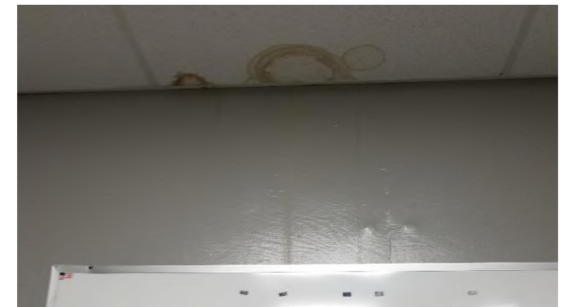
Visiting Locker 023.21: Water damage at ceiling, east wall.
