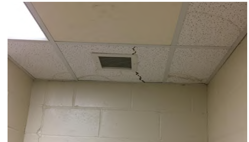
Holding 213.14: Water stains and damaged ceiling tile.
