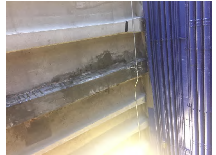
Field Tunnel: Newly repaired roof structure and roadway above tunnel continues to leak. Repairs 2018.
