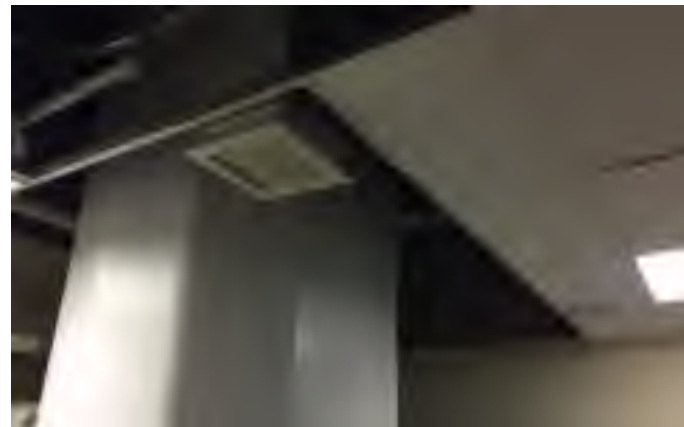
Janitor 229.05: Ceiling tiles not replaced after leak repair.
