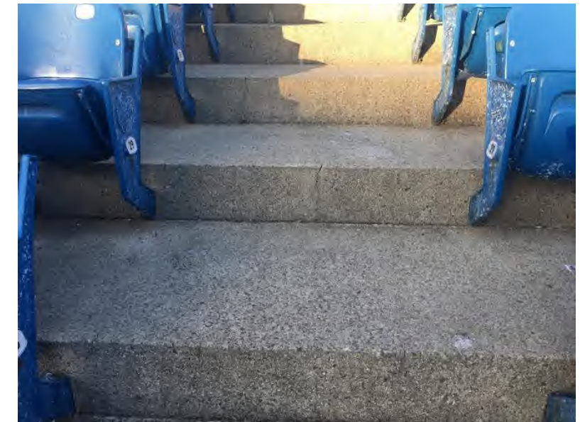
Lower Bowl Seating Slab: Typical condition of on-grade seating slab – note vertical shrinkage crack.
