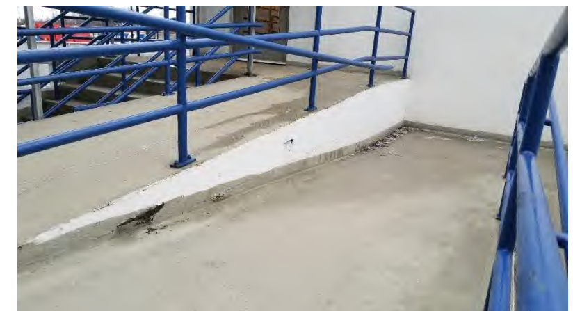
West End Ramps: Walls and slabs are deteriorating.
