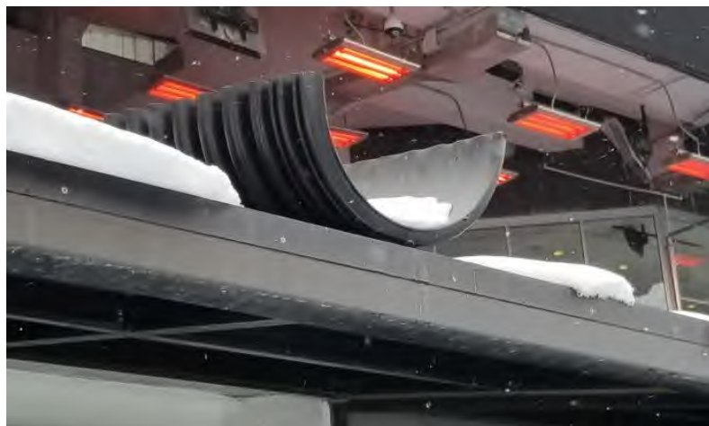
Snow removal: Plastic half-round chutes are used to pass snow down to lower levels.
