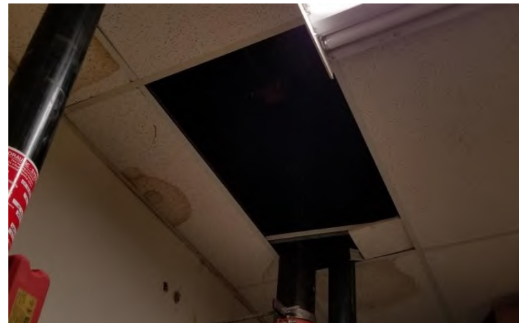
Home Team Locker Mechanical Room: Water damage at ceiling.
