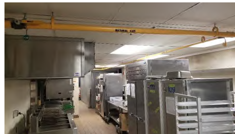
Kitchen 230.04: Suspended gas piping is present above food preparation areas, creating a dust shelf condition. Health Code.
