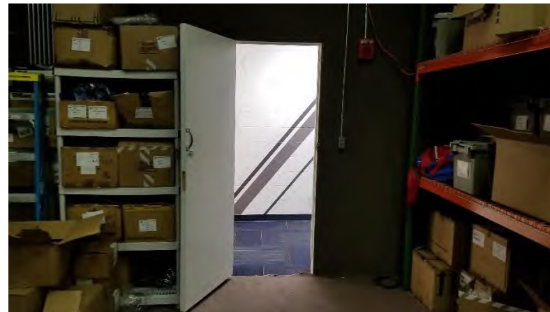
Storage 012.14: Former handball court. Door lacks code compliant hardware.
