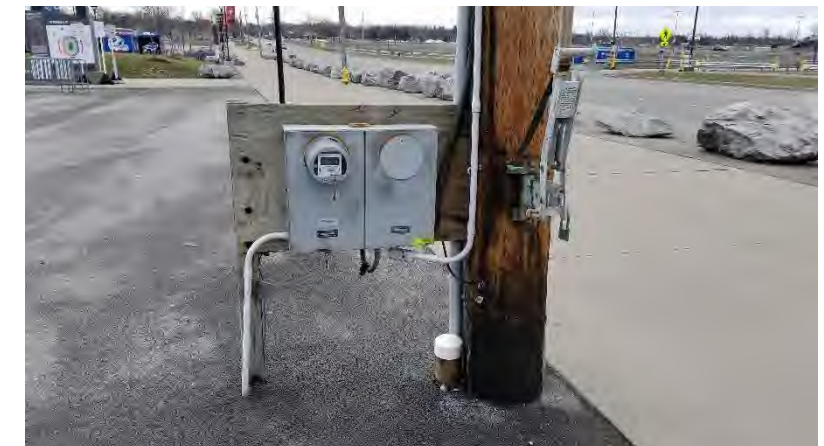
Electrical Service Entry: Two service entry meters and knife switches are unprotected and readily accessible to the public along Abbott Drive.
