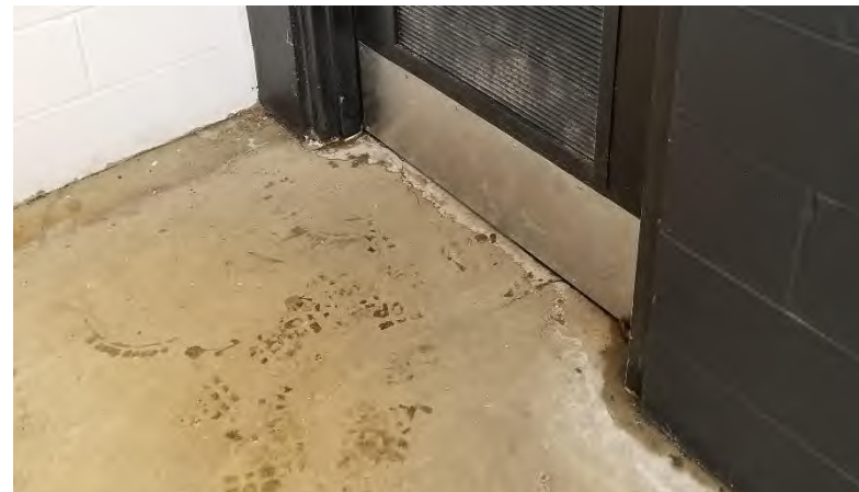
Outside Men's 121.05: Water drains into room under door.
