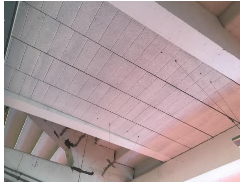
Upper Deck Vomitory Bridge: Typical "cmu-block plank" construction of concourses and suspended vomitories.
