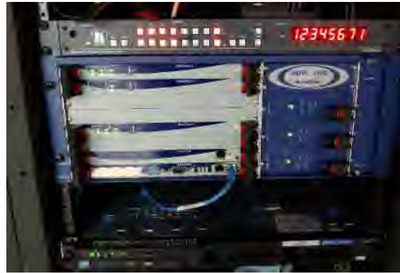
Figure 17- Vitec IPTV Headend Encoders and Server
