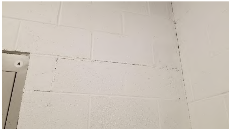
Elevator Lobby 331.05: Masonry exhibits cracking and movement in several directions.
