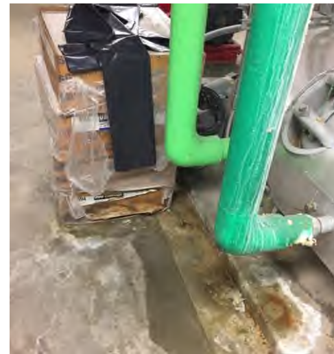
Boiler Room 023.17: Water leaks from above are corroding connectors and staining floor.
