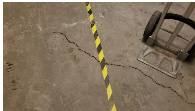
Slab-on-Grade Cracking: Old shrinkage cracks are present in many SOG areas within the building. Joints should be sealed.
