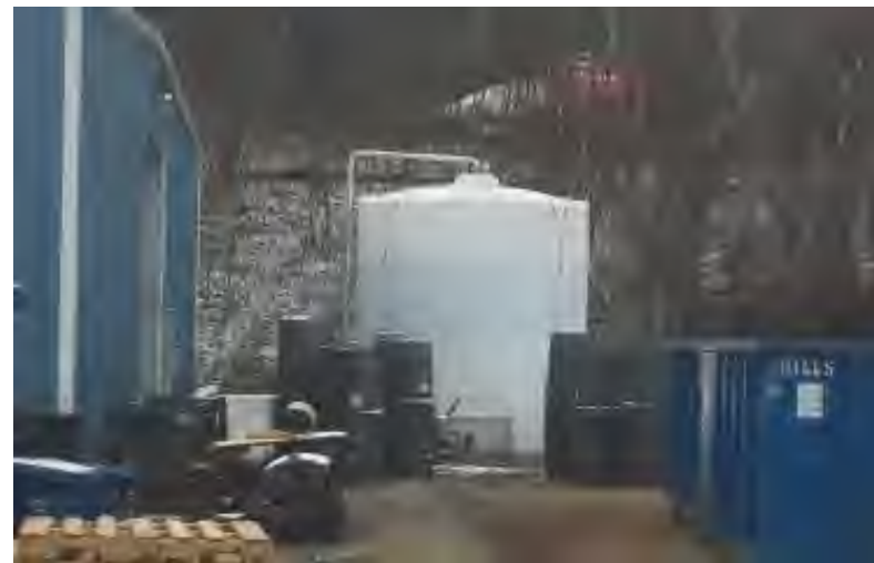
Salt Brine Tank: Salt brine is used to melt snow in seating bowl.
