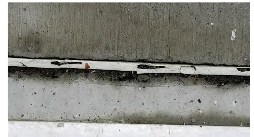
Outside Door 124.08: Zip-strip was never removed and sealed at joint in floor adjacent to grid line 48.
