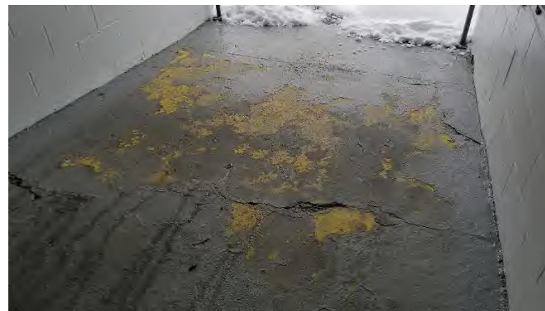
Vomitory 131.01: Traffic coating damaged by snow removal operations.
