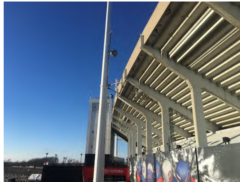
Typical Field Light Tower: Viscous dampers bracing light tower at top of upper deck – one of two dampers have failed in most locations.
