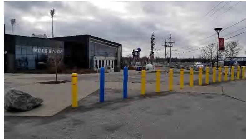
Hardening Line: Areas near the Team Store and Entry Gates are protected with bollards.
