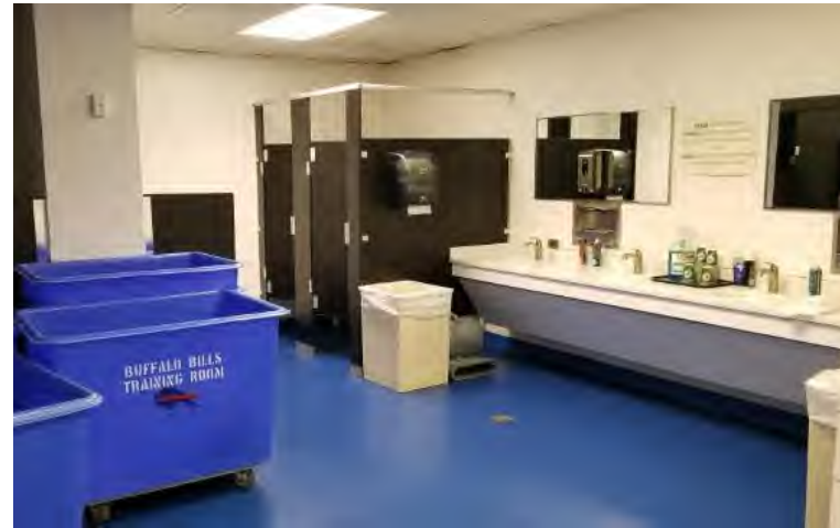
Game-Day Lockers: Stalls are not accessible. Lavatories do not provide knee clearances. Mirrors and accessories are not mounted at accessible heights.
