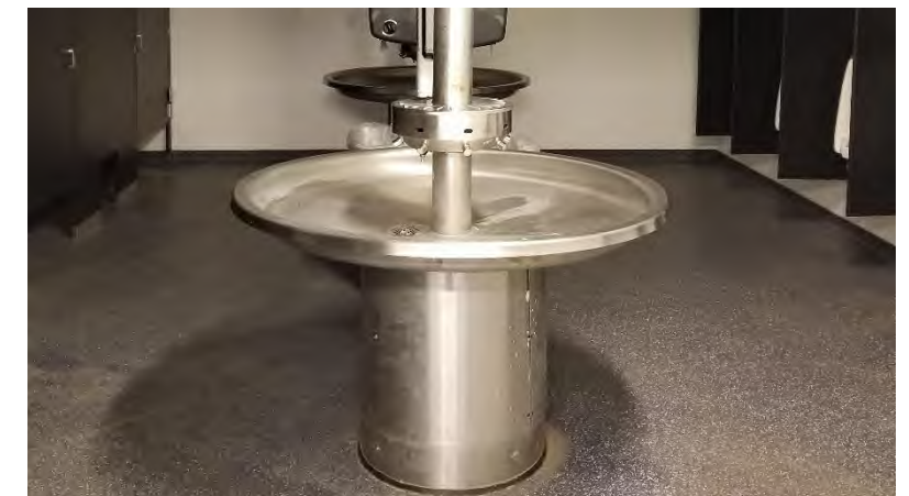
Gang Lavatories: Gang lavatories of several types still remain in many public restrooms. These lavatories do not provide accessible clearances or controls within allowable reach ranges.
