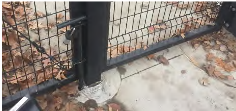
Gate 3: Column foundations re-poured to prevent racking.
