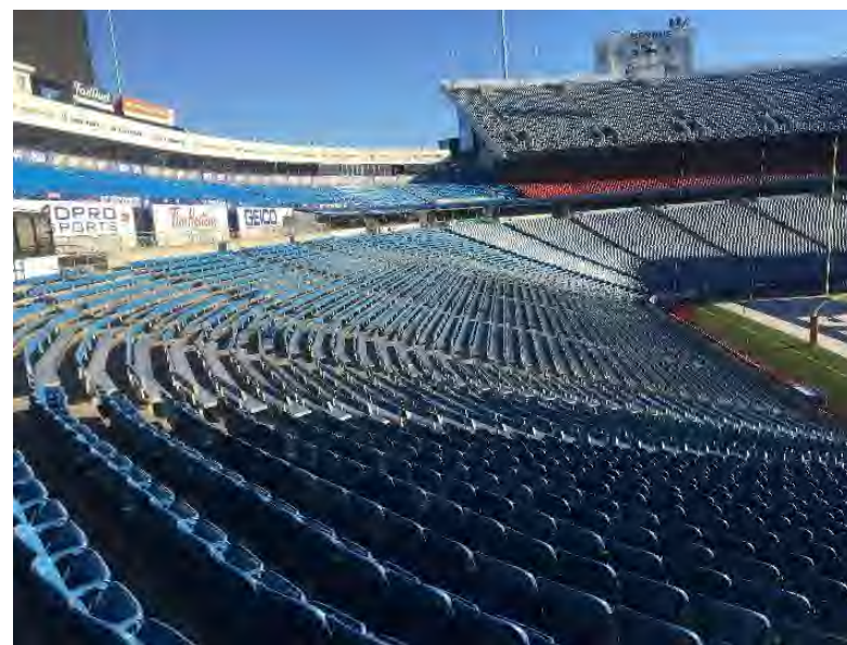
Lower Bowl: Typical configuration of on-grade seating
