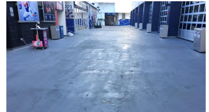
Field Access Tunnel: Bonded Overlay and Traffic-Coated area of tunnel and rooms between Admin Building and Stadium.
