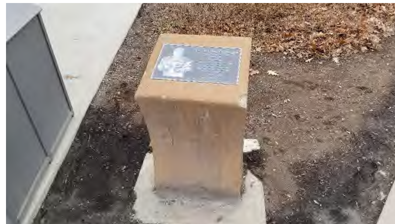
Monument: The Tim Russert monument exhibits cracking and spalling of the concrete base.
