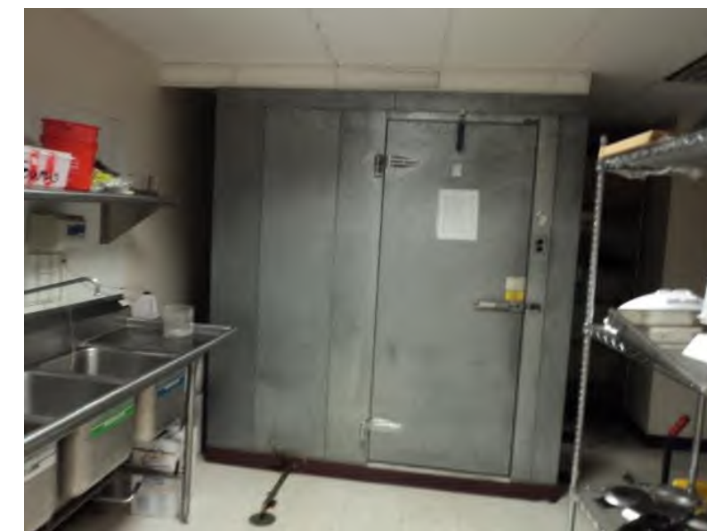
Pantry walk-in very old and undersized. Does not include a ramp; a tripping hazard to staff.
