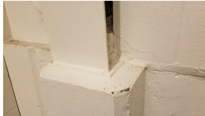
Retail Warehouse 3039: Masonry cracked at structure.
