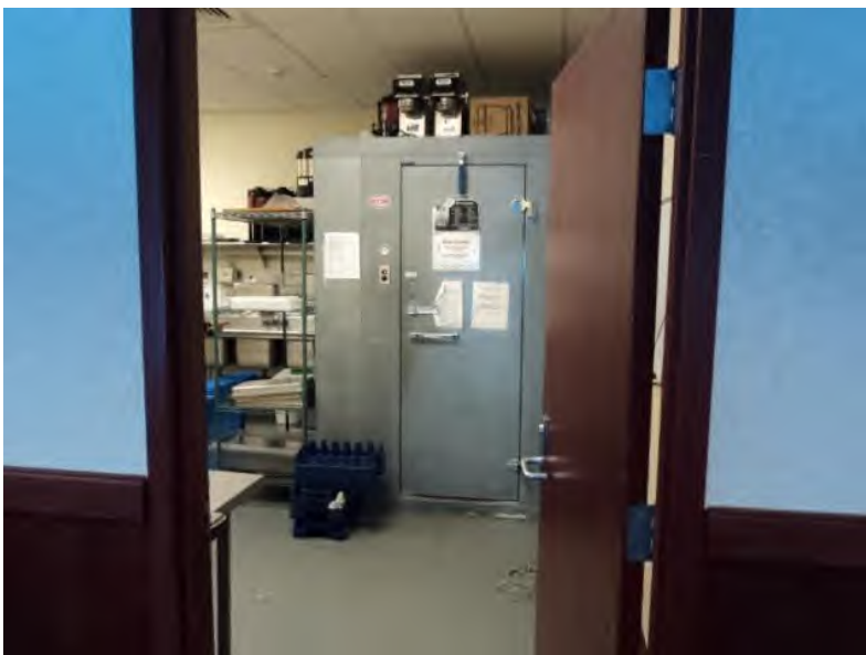
Pantry walk-in very old and does not include a ramp; a tripping hazard to staff.
