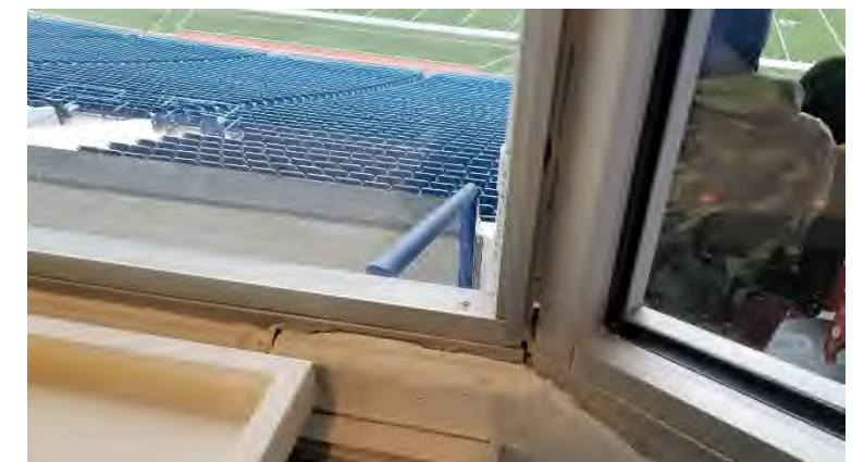
Super Suites: Expansion joints were not established through window system at Grids 63 and 70, leading to water intrusion and air infiltration.
