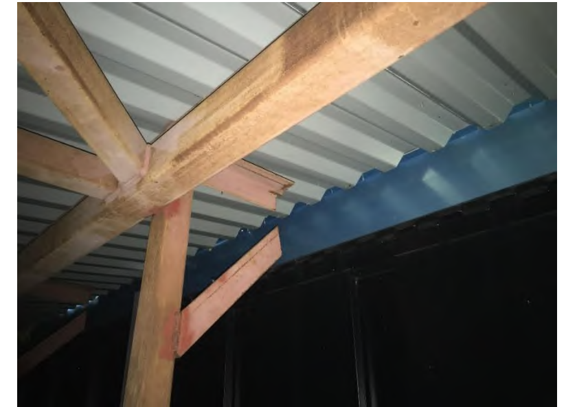
Main Scoreboard: Missing perimeter angle at top of main scoreboard.
