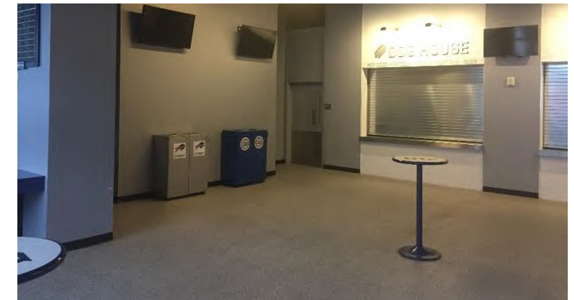
East End Bar: New MMA Floors installed in 2017 within bar and restrooms.
