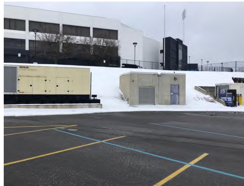
Existing Diesel Generators
