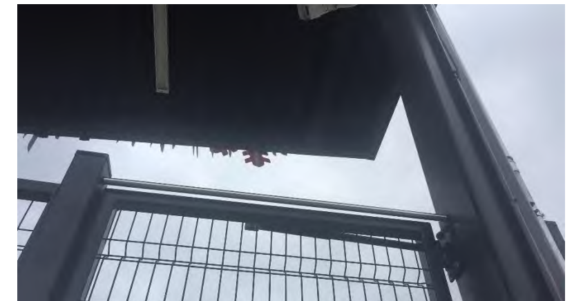
Gate 3 Egress Door: Gates are racking preventing the egress doors to properly close. Bars added to prevent racking.
