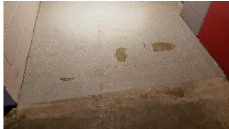
100 Level Suite Entry Alcoves: Alcove floor coating is failing to various degrees in most alcoves.
