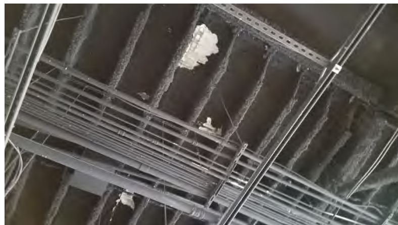
100 Level Concourse: Birds peck at exposed underslab insulation.
