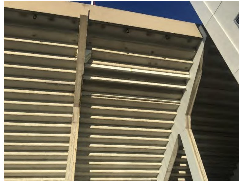
Upper Deck Seating Panels: Typical configuration of upper deck precast concrete seating panels.
