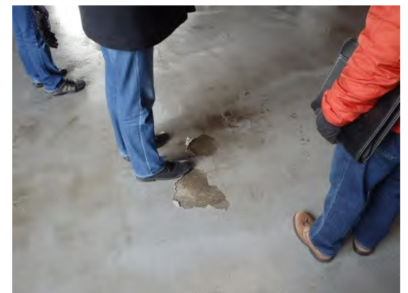
300 Level Concourse: Typical deterioration of the protective urethane membrane on the 300 Level Concourse slab.
