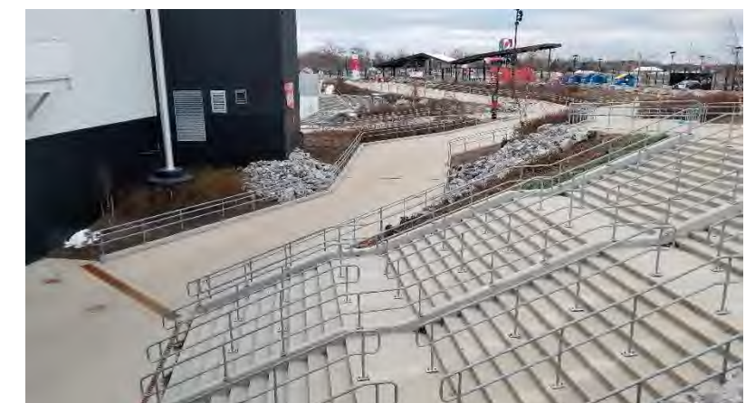
West Ramps & Stairs: Bills report that snow removal is difficult due to tight turns at landings. Snow pushed uphill to be removed.
