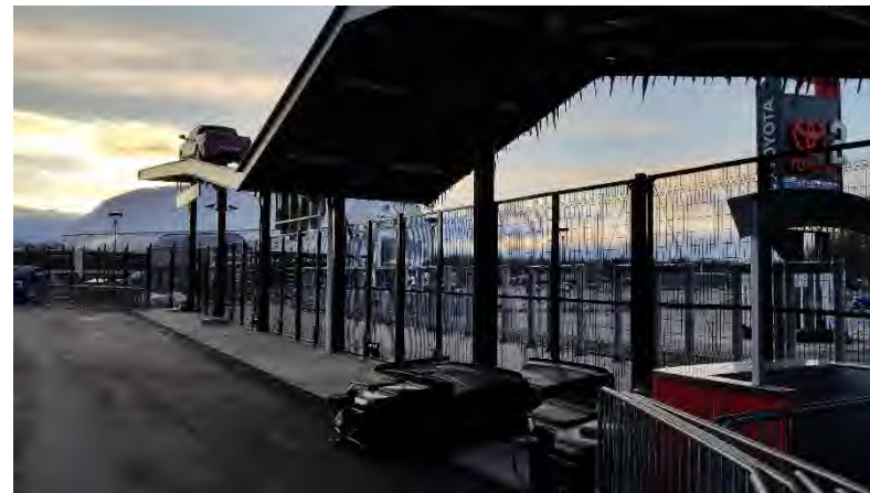
Entry Gate 2: Slab-on-grade slopes to create valley where it meets asphalt. Condition repeats at Gates 2, 3, and 4.
