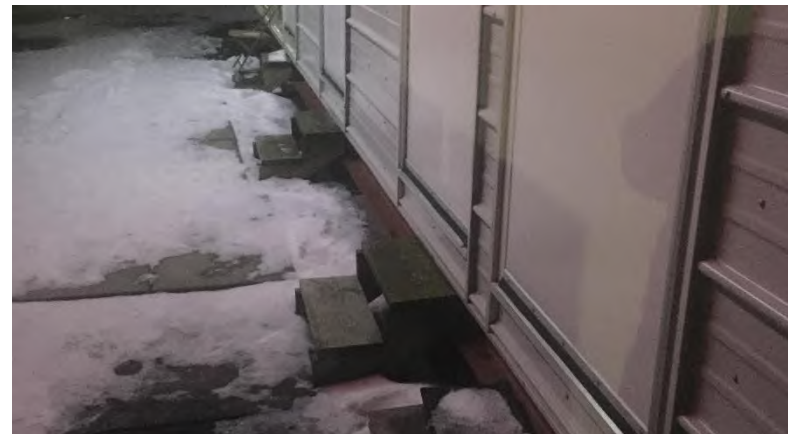
West End Camera Booths: Stairs not securely fastened and lack compliant railing. Ice buildup from above.
