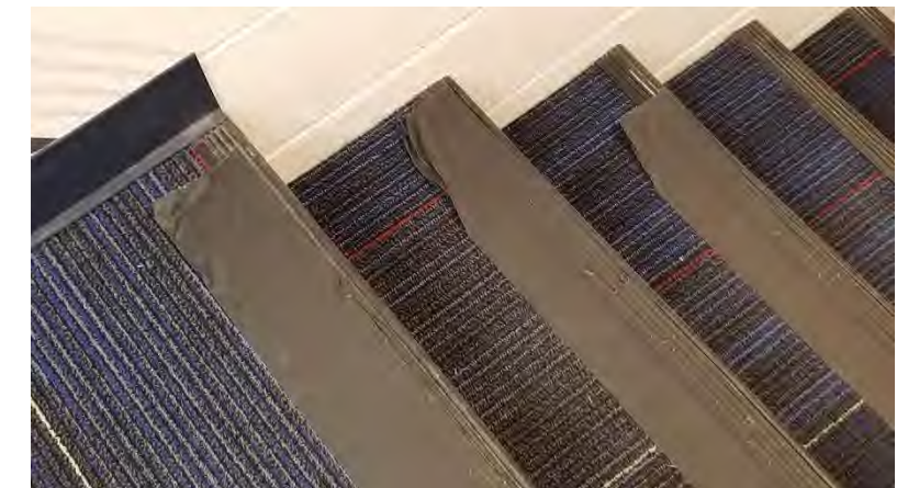
Corridor 021.13: Damaged tread nosings on stair.
