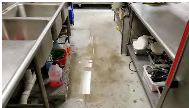
Concession 107.05: Uneven floor surfaces trap water against a grease interceptor.
