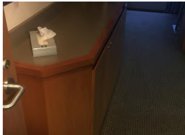
West End Suites: 75% of unrenovated suites had millwork installed at entries that prevent proper door clearances.
