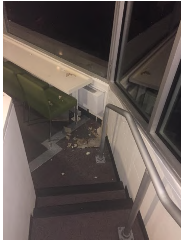
200 Level Sideline Super Suites: Water damage along expansion joints above. Both Suites experience substantial water damage to finishes.
