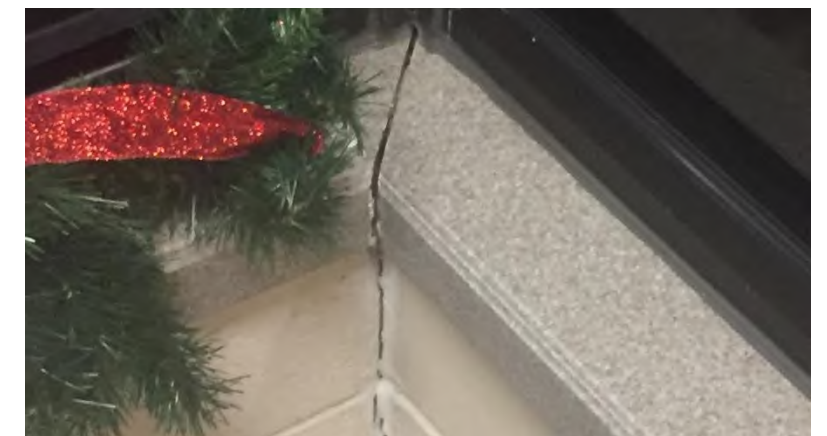
Suite 240A: Block cracking and separating at corner.
