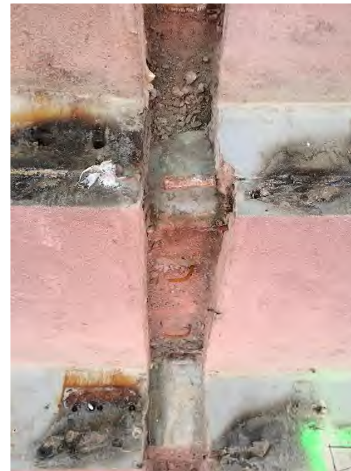
200 Level Seating Panels: General joint configuration and deterioration of extended PT strands observed during joint reconstruction.
