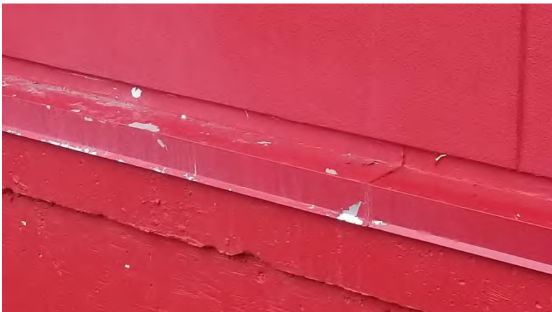
South 50-Yard Line Plaza: Paint on flashing is peeling above monumental stair.
