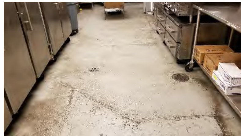
Typical Concession: Worn and damaged floor coating. Floors do not slope toward drains.
