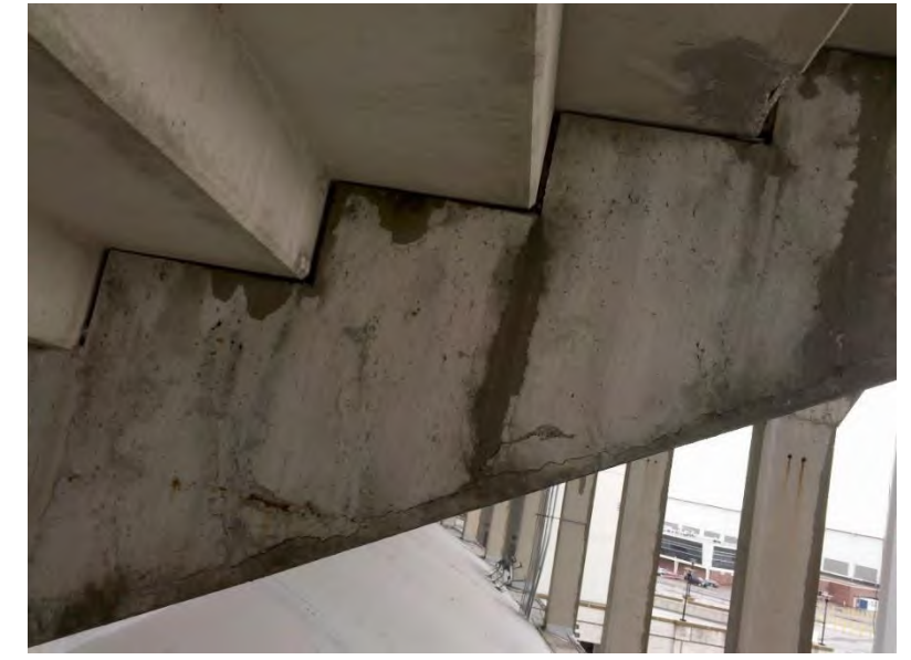
Typical Area of Upper Deck Frames: Typical leakage through deck joints (Pre-2014) – leakage currently occurring primarily at expansion joints since 2014 repairs/improvements.
