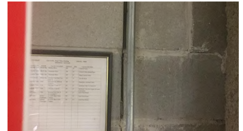
Mechanical 209.09: Control joints not proper sealed in many of the MEP spaces below the ramps. Daylight visible in some locations.
