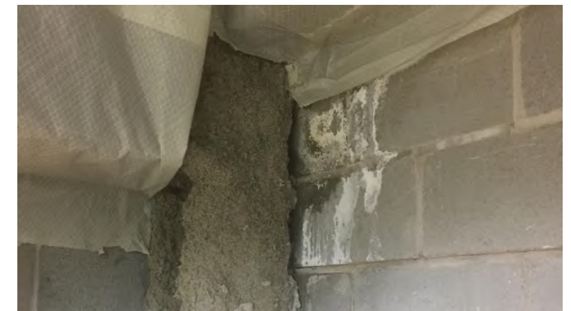
Mech 209.09: Water leaking from ramp above.
