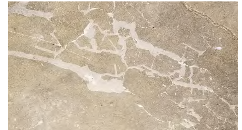
Team Store Retail Area: Clear sealer on floor is peeling in areas. DNC reports this started after a vendor worked in the space.
