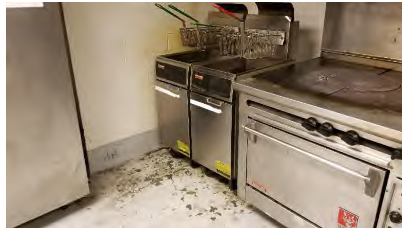
100 Level Pantries: Floor coating has been damaged by stray hot grease.
