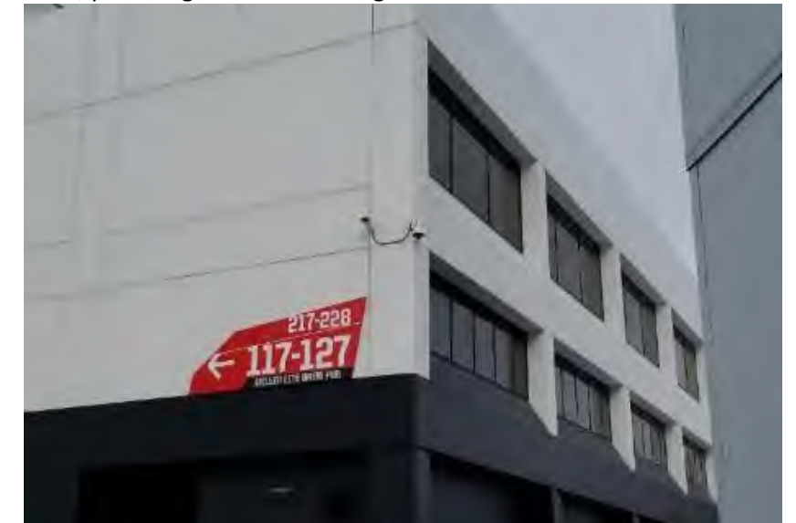
Figure 3 Exterior PTZ camera for site coverage
