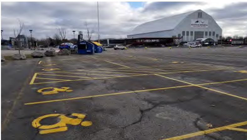
Lot 2 Overflow Accessible Parking: Accessible stalls and access aisles are not provided with identification signage.
