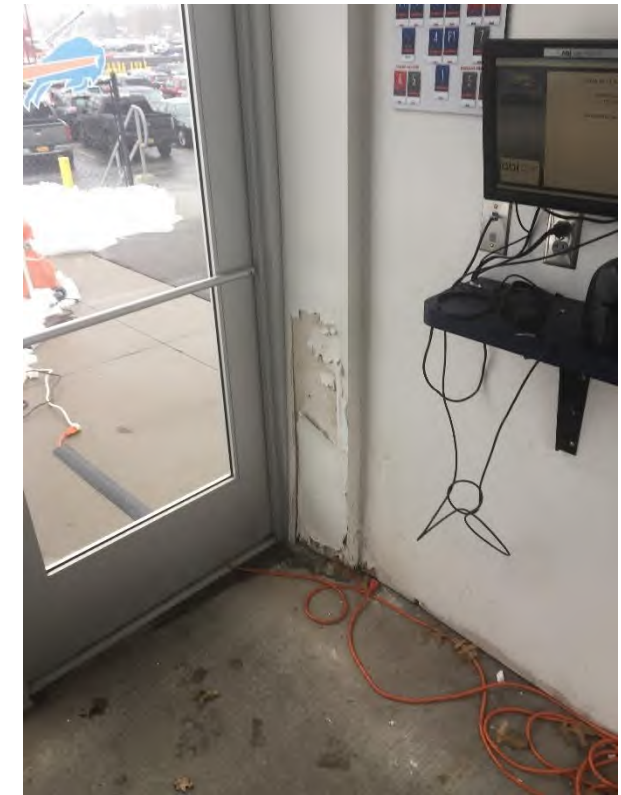
Gate 1 Booth: Pavement has been regraded and trench drains added in front of booth entrances, but substantial water damage has already occurred.
