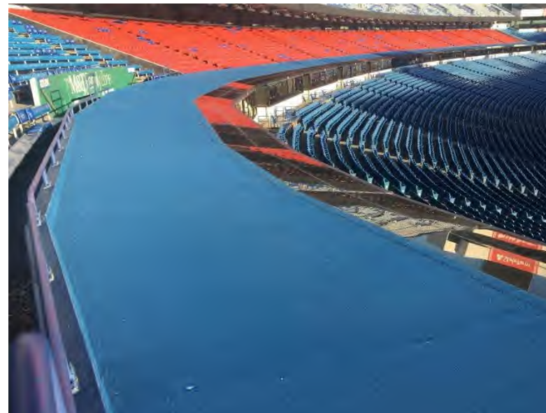
Dugout Suites: Interface of suite roof with upper ringwall – site of continuing localized leakage issues.
