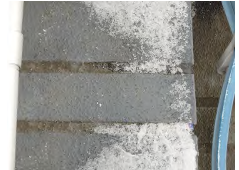
Typical Upper Level Seating Area: Expansion joints above rakers are either waterproofed coated with reinforcement scrim or older applications do not have reinforcement over the sealant joint.
