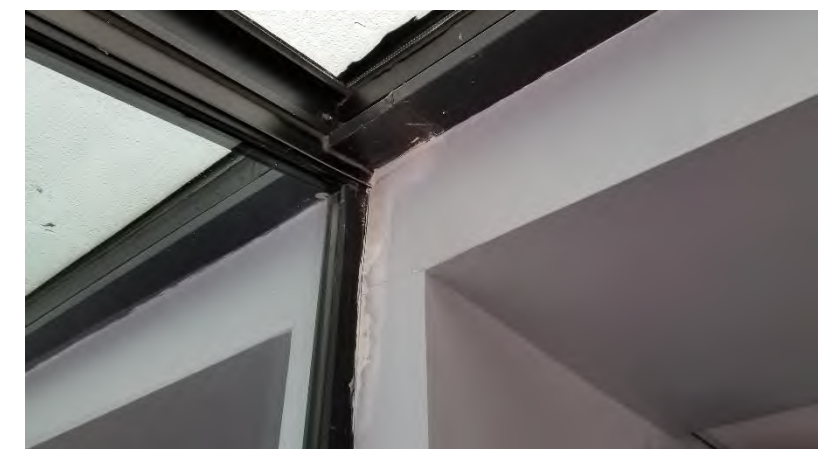
Dugout Suites: Joint between skylight framing and concrete bowl structure allows water into some suites below.
