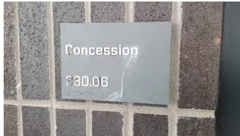
Exterior Room ID's: Several door signs on the 300 Level Concourse exhibit corrosion on the text of signage.
