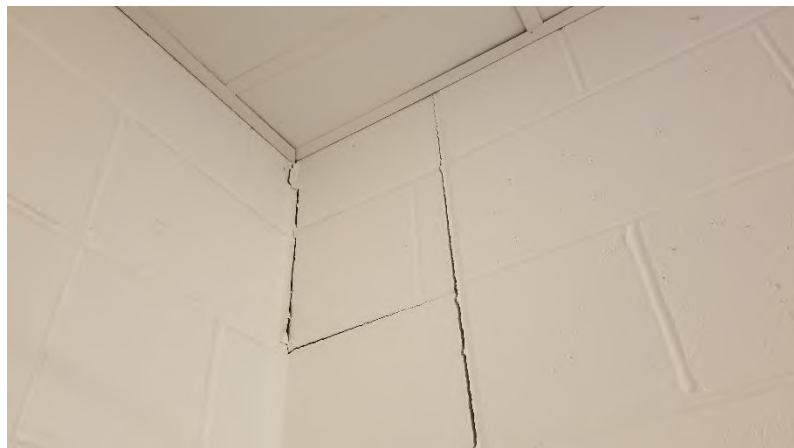
Concession 334.04: Movement between structure and masonry walls.
