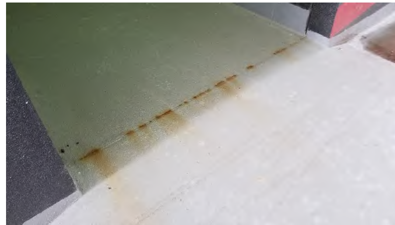
Outside Women's 331.04: Traffic coating has worn off of slab edge angle leading to rusting of the angle.
