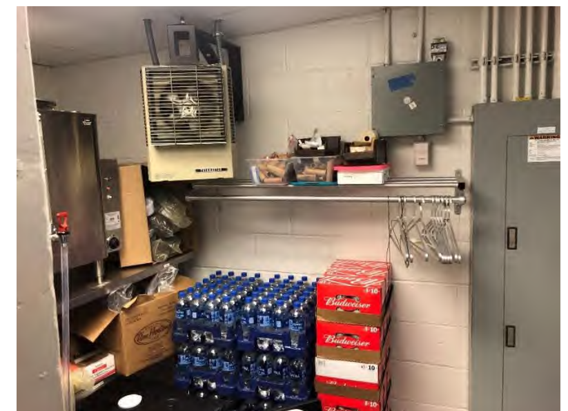
Unit heaters are hung low within spaces. Single heater locations leads to uneven heating and freeze problems.
