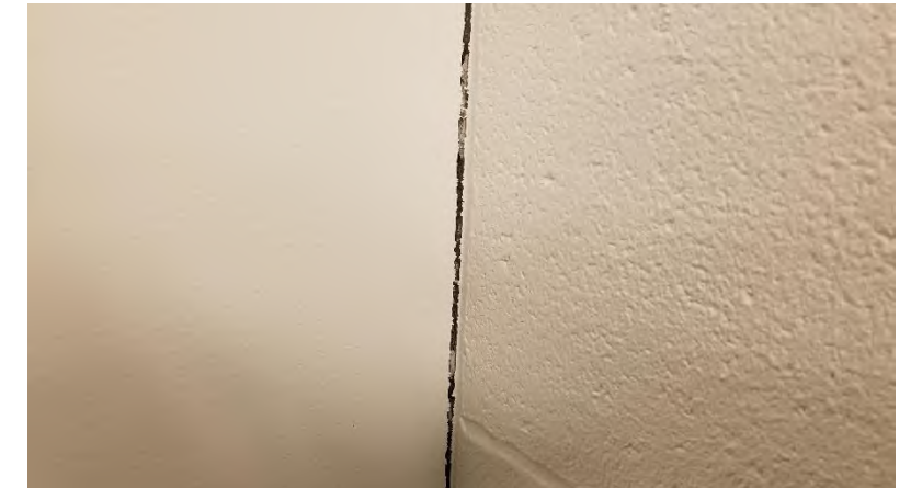
Commissary: Sealant joints between interior drywall partitions and exterior masonry partitions were never sealed.
