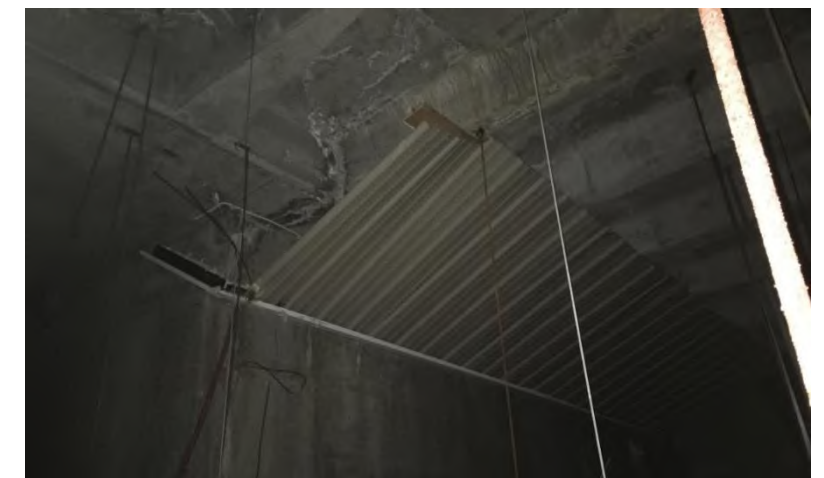
Room Adjacent to Tunnel: Leakage containment at north end of tunnel over team medical offices.
