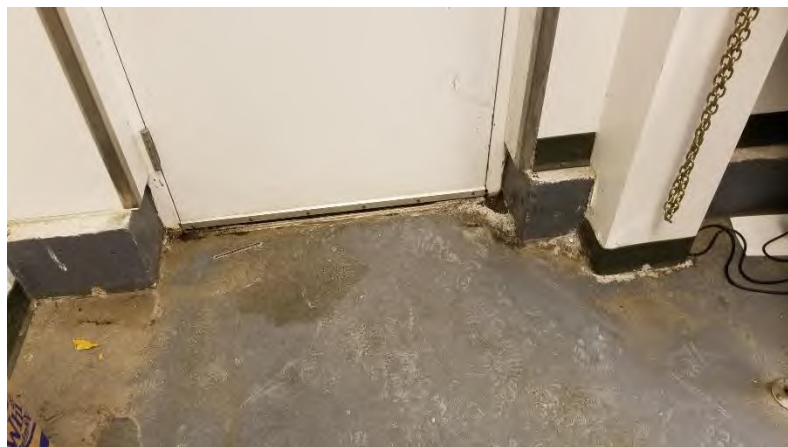
Concession 330.06: Slabs outside this door slope water toward the door bringing salt and debris inside.
