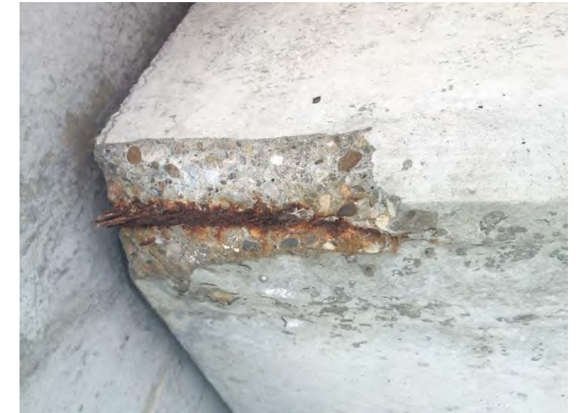
Underside of Elevated Seating Panel: Typical spalled seating panel at nosing exposing corroded PT strand.
