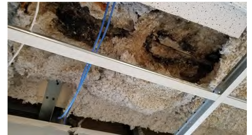
Dugout Suites: +/- 25% of all Dugout Suites exhibit some degree of water damage from leaks in the seating bowl above.
