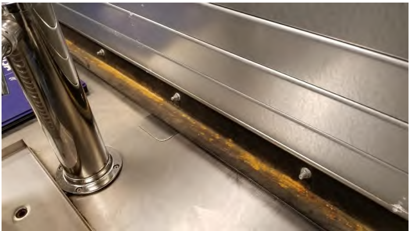
Concession 139.06: Bottom bar on overhead door is rusting
