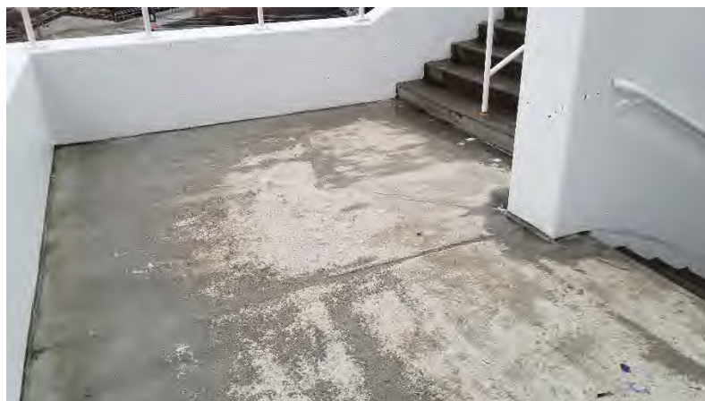
Corner Stair Landings: Traffic coatings protecting Retail spaces below are old and worn.
