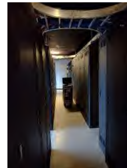
Figure 9- Production headend racks. Hot aisle lacking dedicated exhaust diffusers.
