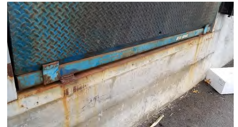
Dock Area: Dock levelers exhibit rust, especially at exposed connections.
