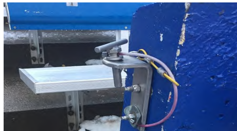
Field Wall Gates: Paint damage consistent at all gate locations. Gates newly replaced and are in decent condition.
