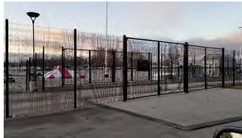
Perimeter Security Fence: The size of openings in the existing fence does not meet recent NFL standards.
