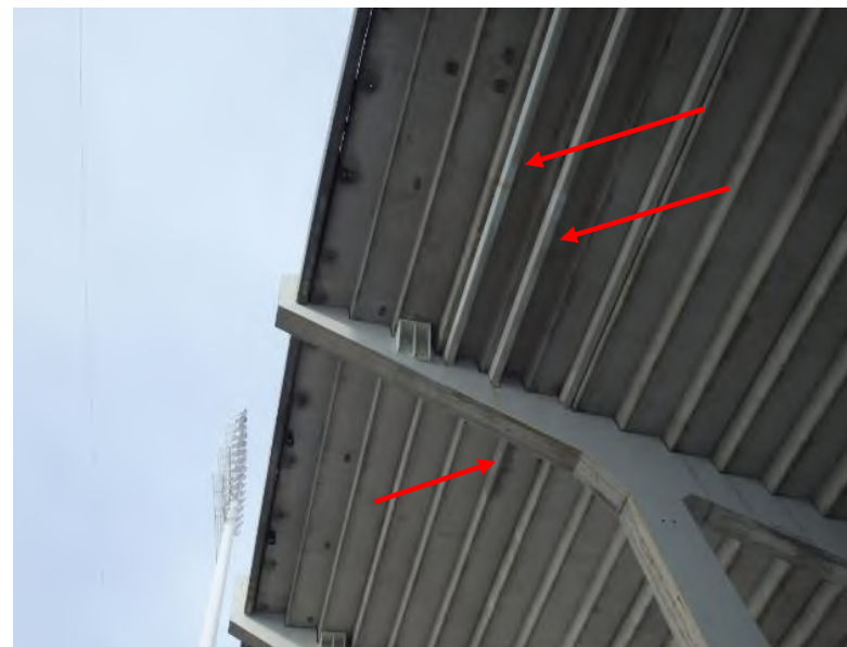
Elevated Seating Panel: Arrow indicates concrete repair on precast beam and supplemental box tubing installed on underside of precast beam.
