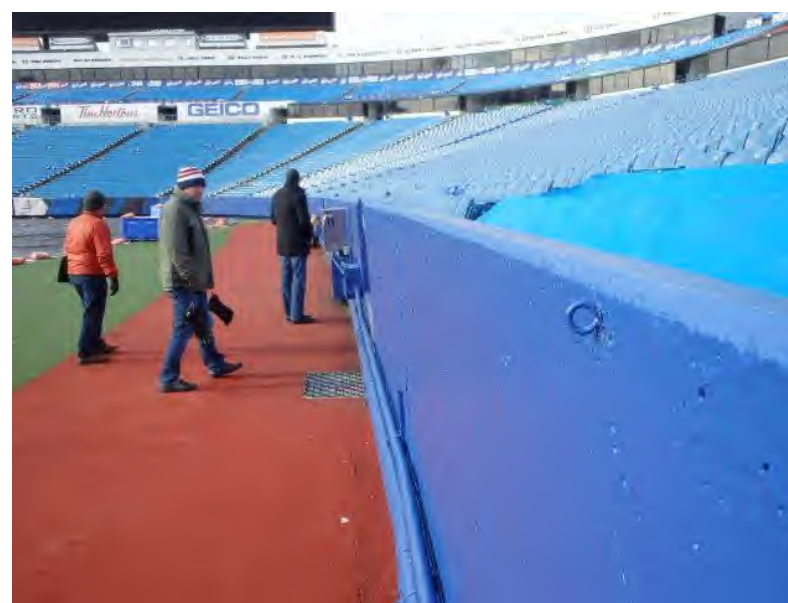
Lower Ring Wall: View of leaning, out-of-plumb Lower Ring Wall.
