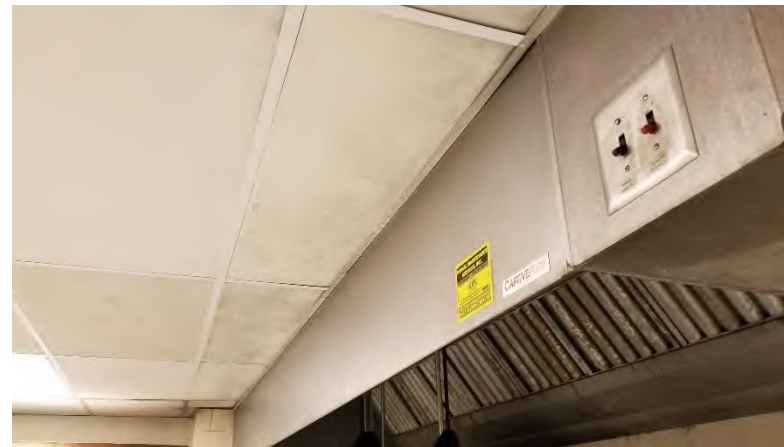
100 Level Pantries: Ceiling tiles have been stained by grease.
