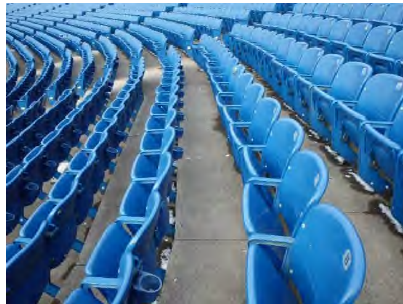
On-Grade Lower Bowl Seating Area: Treads for Lower Bowl seating. Sawcut joints are visible in the treads, with sealant in fair to poor condition.
