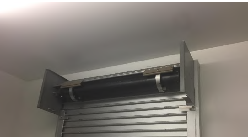
West End Camera Booths: Overhead coil shroud missing.
