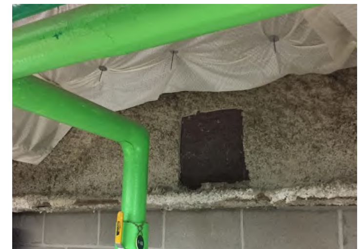
Mech 214.06: Plastic placed to catch falling insulation created by water damage from ramp above.
