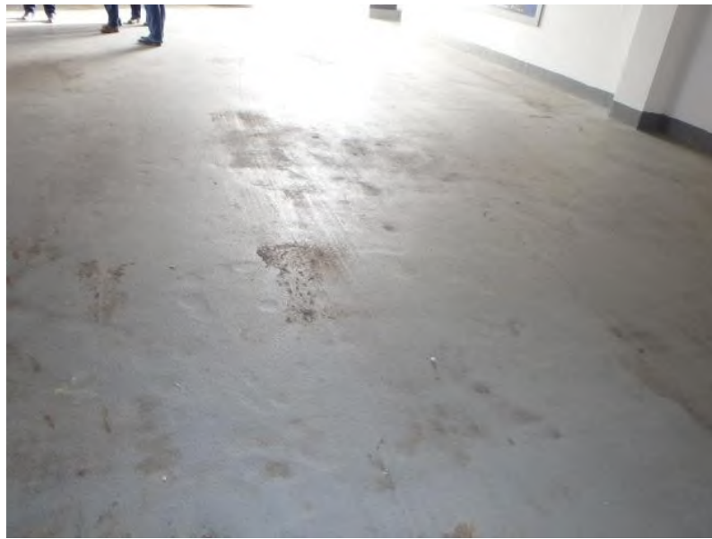
300 Level Concourse: Typical view of 300 Level Concourse with protective urethane coating over non-uniform finished concrete slab.
