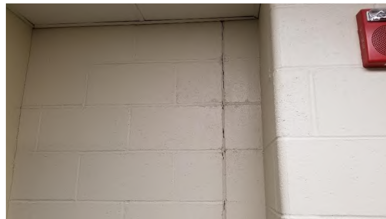
100 Level Concessions and Restrooms: Sealant joints in walls at locations where newer partitions meet older partitions have failed in several locations.
