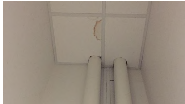
Closet 321.05: Water damage at ceiling.
