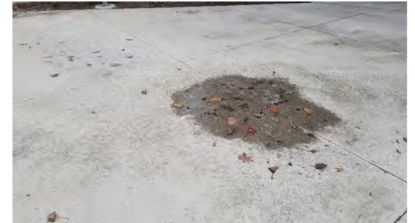
Team Store Plaza: Low spot creates need for intense use of salt, which leads to spalling concrete surface.
