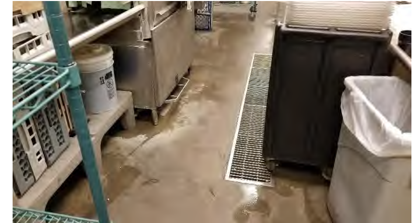
Commissary Kitchen: Floors do not slope to trench drains.
