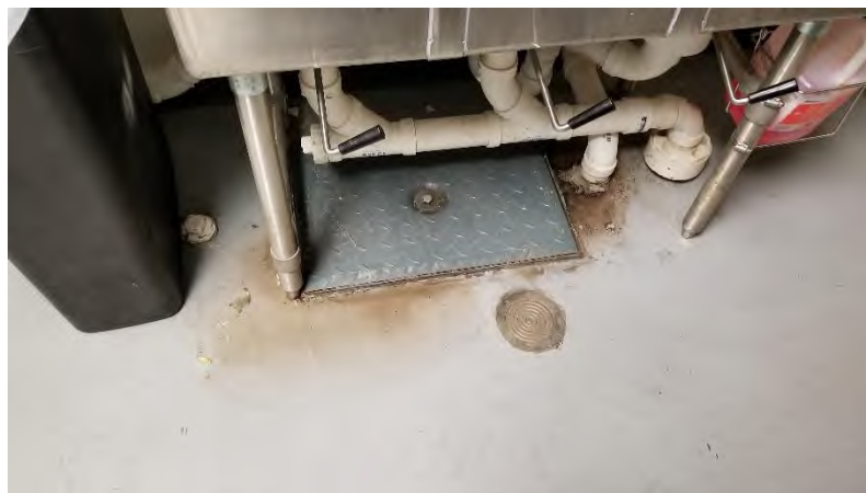
Concession 136.05: Uneven floor surfaces trap water against a grease interceptor.
