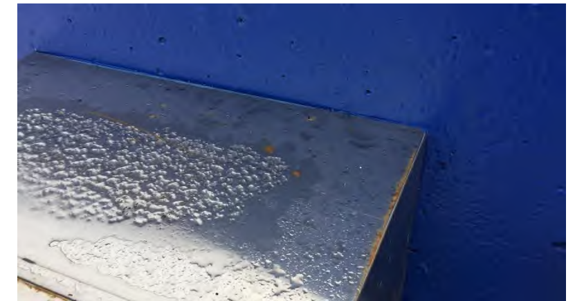
Communication boxes: Rusting and damage noticed a 15-20% of connection boxes.
