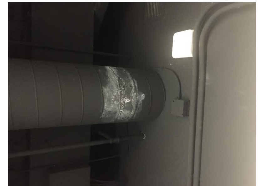
200 Level NFL Broadcast Booth: Water damage from leaks at 300 level above.
