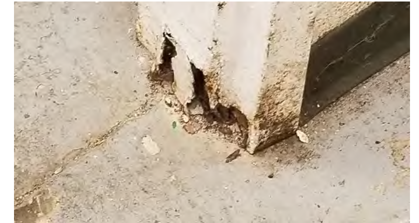
Many Locations: Older door frames exhibit severe rusting at floor
