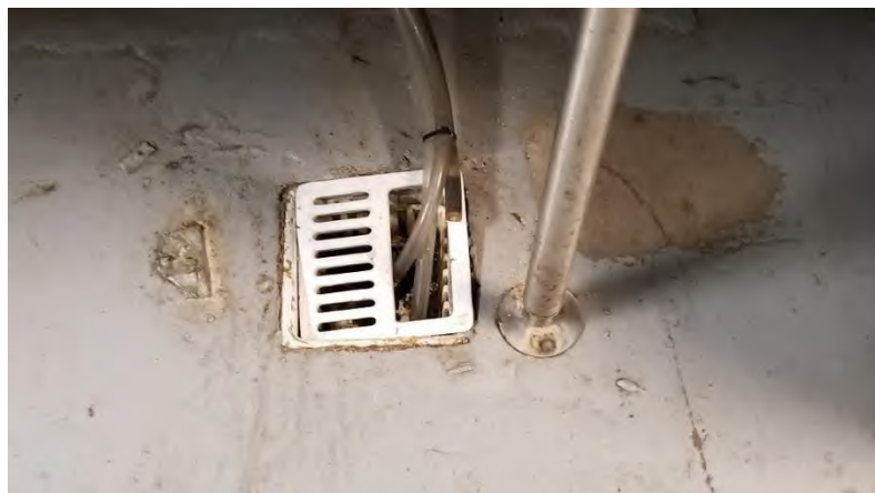
Floor sink grate replaced in some areas.
