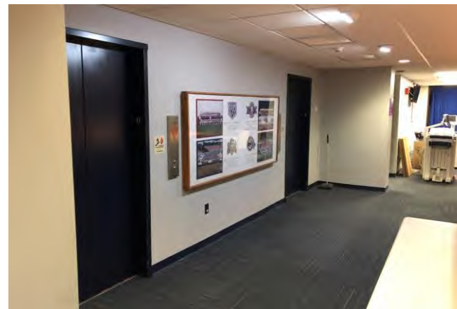
Admin Elevators: Hoistway openings at the 2 nd Floor of the Admin Building sit within an unprotected egress corridor.
