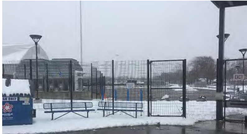
Exit Gates: General Assistance/ADA waiting area directly adjacent to dumpsters. Gates are racking preventing the egress doors from properly closing. Bars added to prevent racking.
