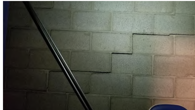
Telephone 021.41: Movement between structure and masonry walls.
