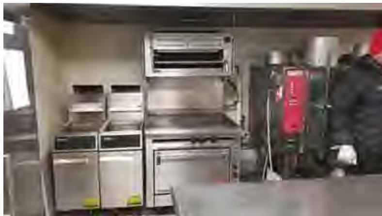
Cooking equipment left on to provide space heat.
