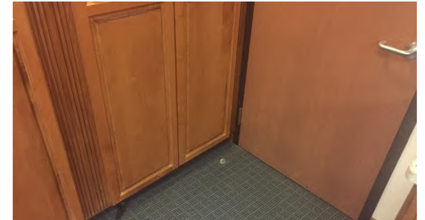
West End Suites: 20% of un-renovated suites have millwork installed behind doors which prevent the door from opening 90 degrees.
