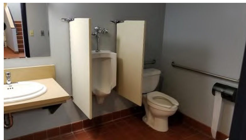
Dugout Suite Restroom 129 AB: Addition of urinal leaves the restroom with inaccessible approaches to any fixture.
