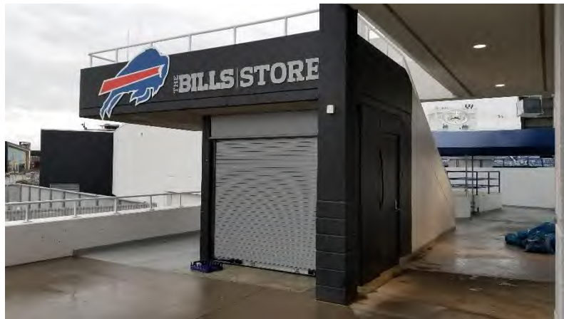
200 Level Corner Retail Stands: Water enters space at floor line and cracks in masonry walls. Typical at four corners of stadium.
