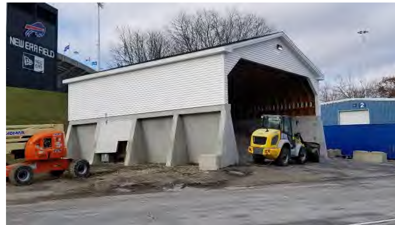
Salt Building: Building was constructed in 2017 and has an asphalt shingle roof.
