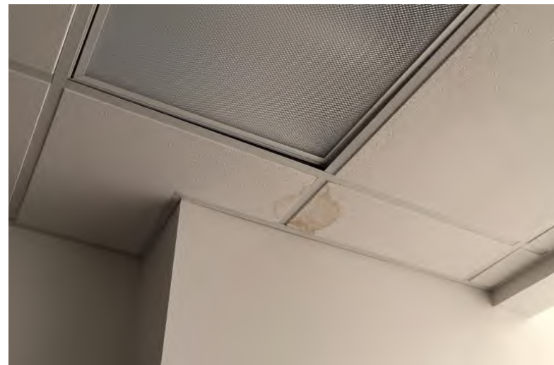
Office 321.07: Water damage at ceiling.
