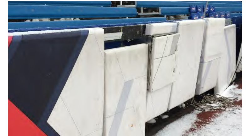
South Sideline Pads: Several pads were loose and or not mounted to the wall. Vinyl last replaced in 2014. Netting guide wires replaced prior to 2018 season.
