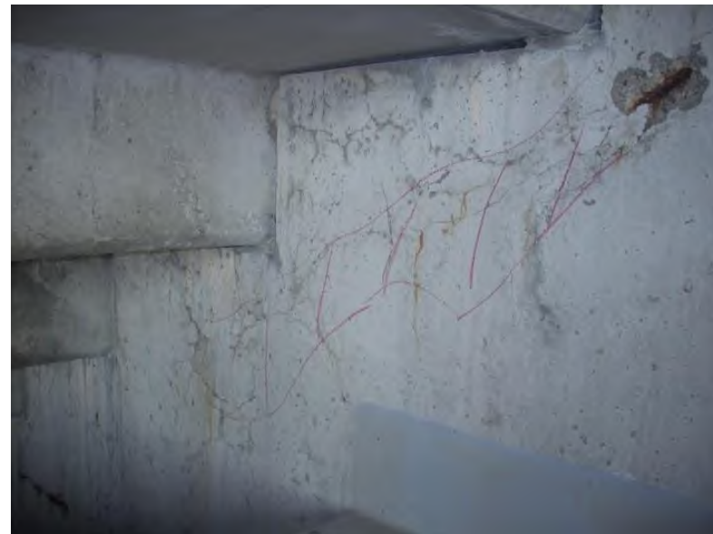
Typical Upper Deck Frames (pre-2014): Typical re-entrant corner cracking, longitudinal cracking along primary reinforcing and localized spall.
