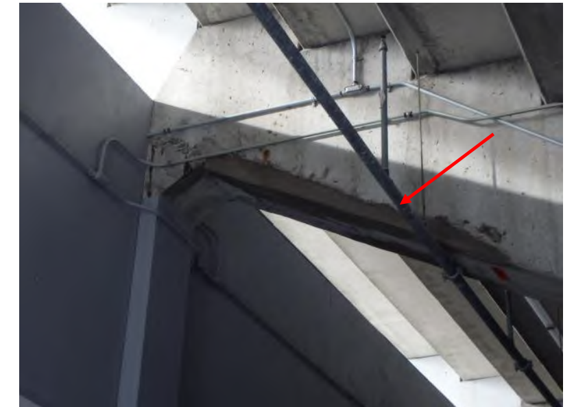
Cast-in-Place Concrete Frame: Arrow indicates previous overhead concrete repairs.
