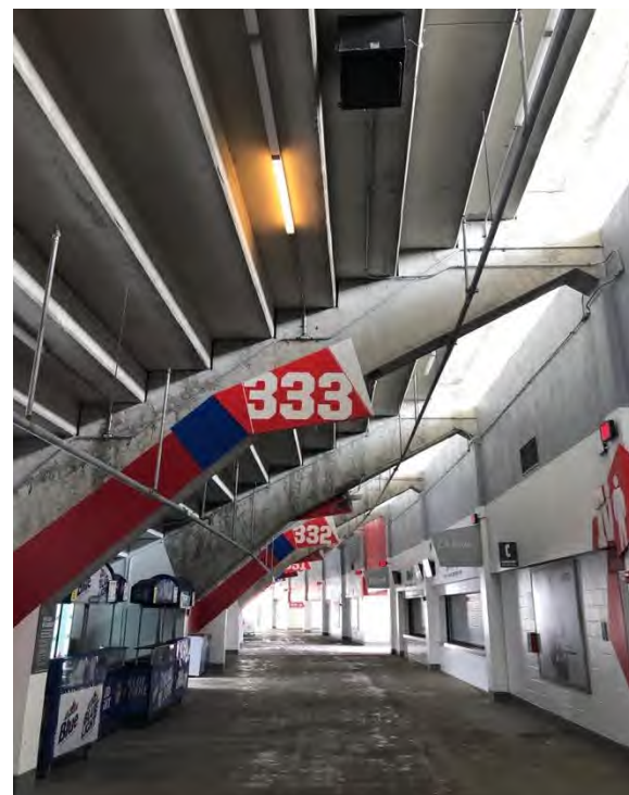
Upper Concourse Fluorescent Linear Lighting – installed in 2014
