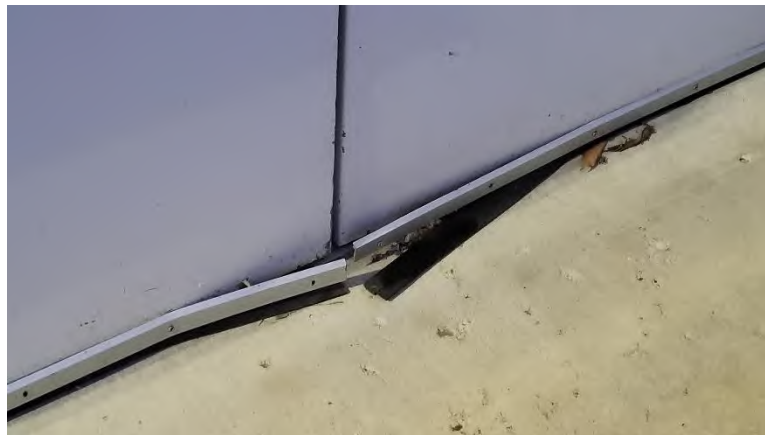
Mechanical Room 3041: Damaged exterior weather stripping on doors.
