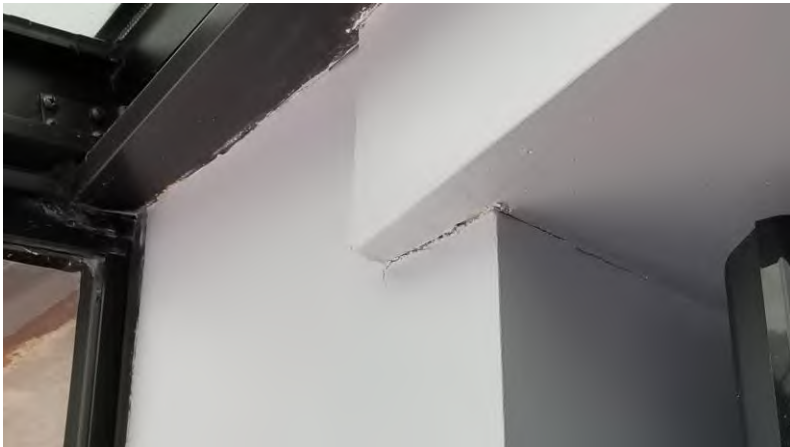
Dugout Suites: Movement between skylight framing and drywall construction is apparent in many suites. Few leaks observed.
