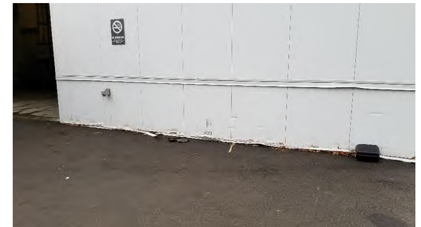
Rear Dock Area: Walls have been damaged by forklifts and snow plows.
