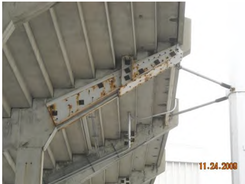
Rear Cantilever of Upper Deck Frames - South: Previous steel repair, typical map cracking, viscous damper anchorage.
