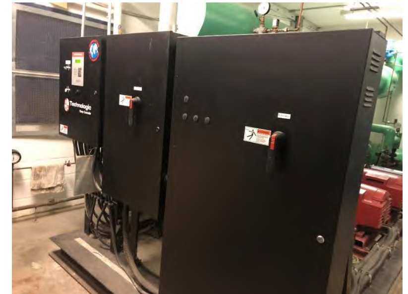
Booster pump control panel.
