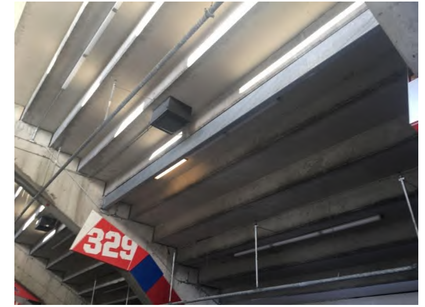
Upper Deck Seating Panels: Typical spall repairs to lower corners and supplemental steel supports where excessive debonding of PT strands exist.
