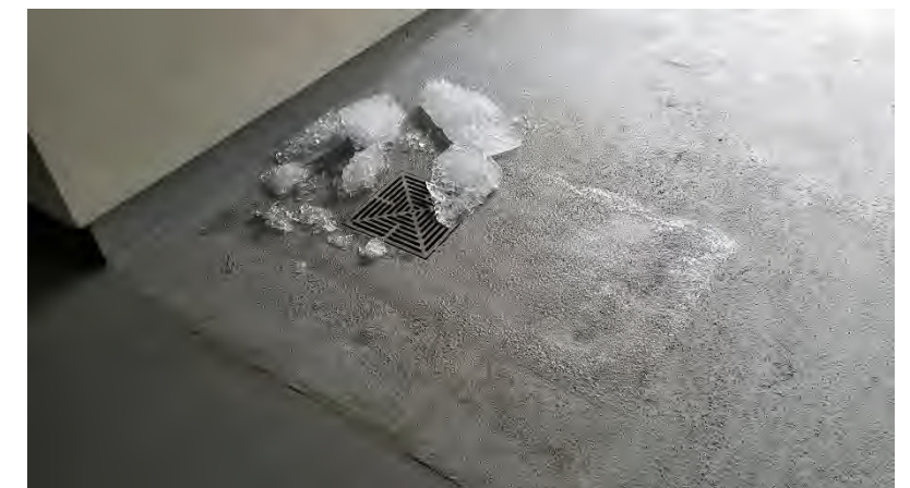
300 Level Concourse: Area drains are frequently used as ice dumps, contributing to traffic coating damage.
