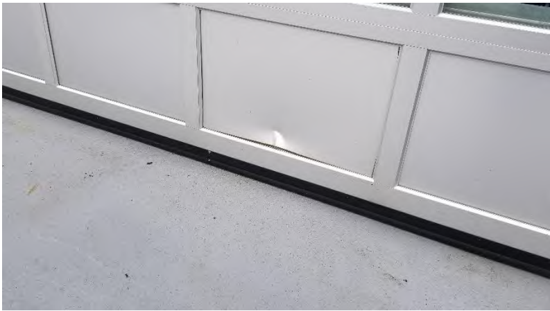
East End Bar: Sectional door bottom panels damaged from impacts.
