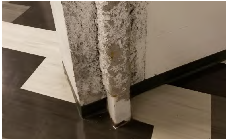
Corridor 023.01: Damaged fireproofing adjacent to Band Locker Room entrance.
