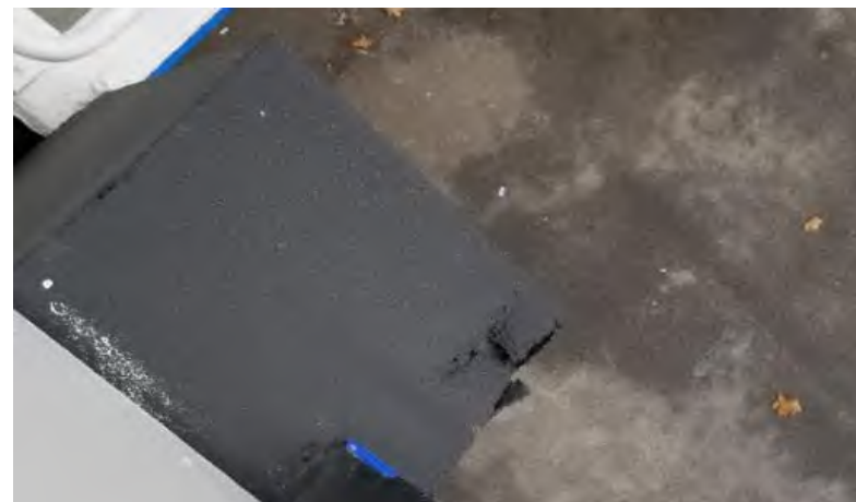
Damaged EIFS: Damage to pilaster outside of east entrance to Dunn Tire Club. View is from above.
