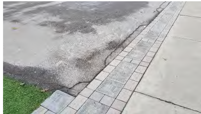
Team Store Plaza: Asphalt is failing along the edges on adjacent donor bricks and artificial turf.
