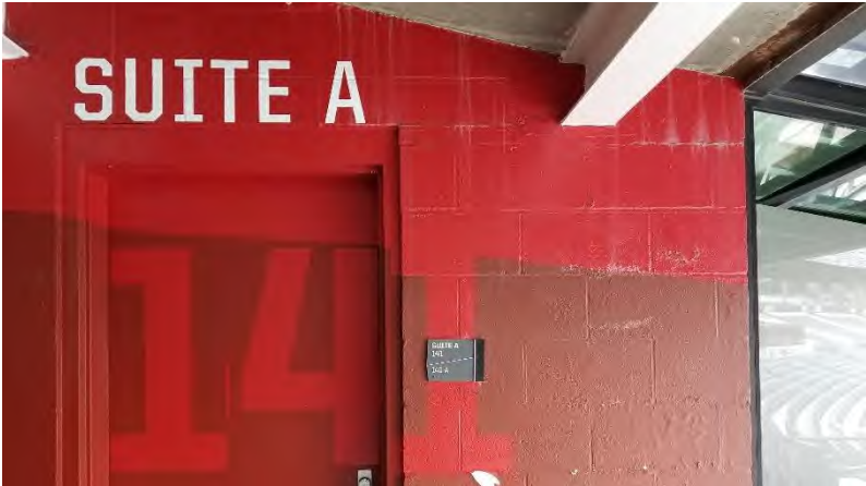
Outside Dugout Suite 141A: Water leaks from the seating bowl above have stained wall and are causing paint finish to peel.
