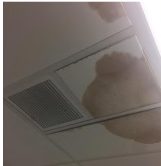
Corridor 021.07: Water damage at ceiling.
