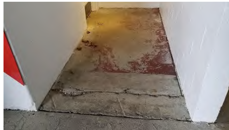
100 Level Restroom Alcoves: Floor surfaces are typically uneven and damaged, with work traffic coatings.
