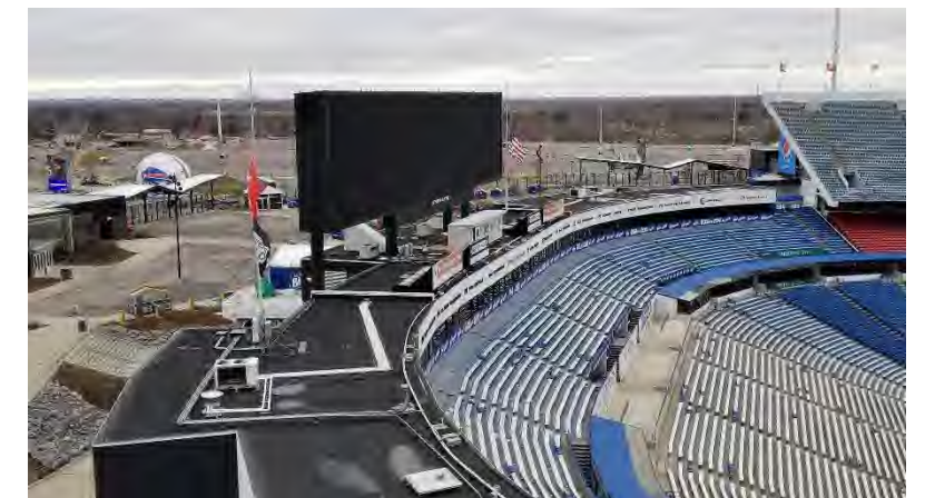
West End Roof: Roofing was replaced in 2018 at north and south ends.
