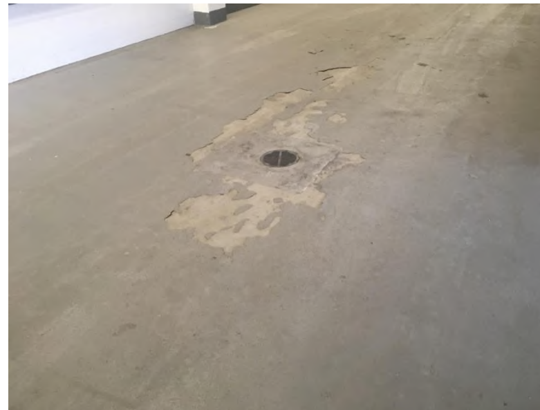
300 Level Concourse: Typical plow damage to traffic coating.
