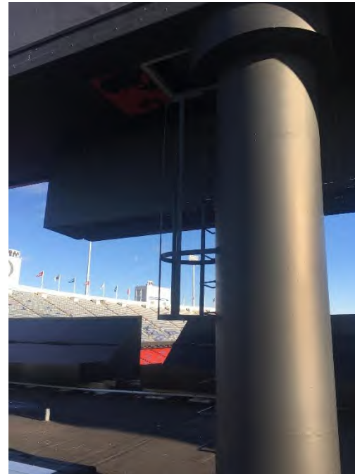
Main Scoreboard: Non-code compliant access ladder to main scoreboard.
