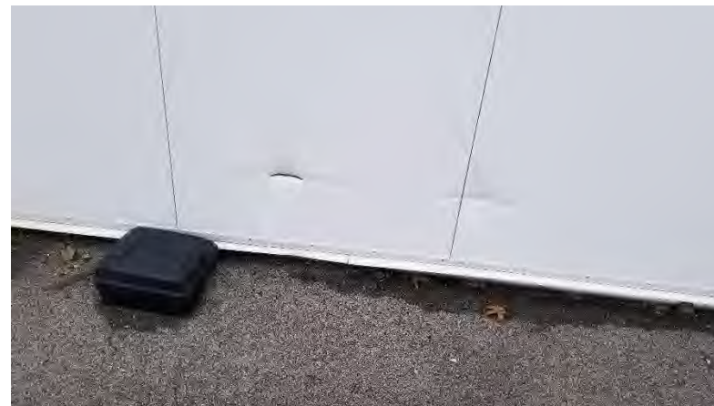
Exterior West Side: Forklift damage to exterior wall panels.
