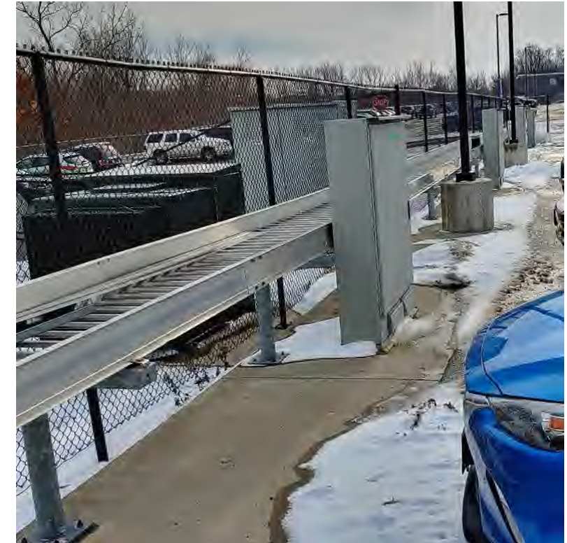
Figure 15- Broadcast truck pad, dedicated power connection interface.
