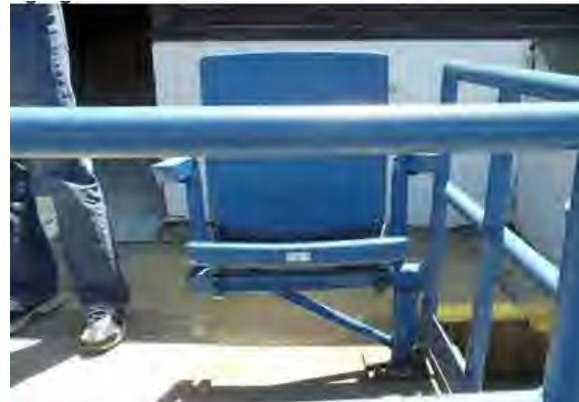
Lower Bowl Swing Seats: Seats that fold away for wheelchairs were added at the bottom of Lower Bowl aisles in 1999.
