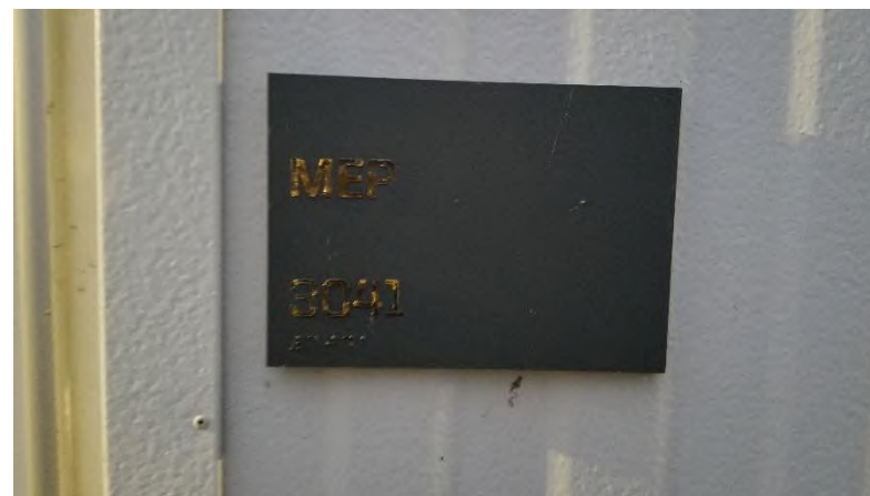
Exterior Room ID's: Several door signs on the east face of the Commissary Building exhibit corrosion on the text of signage.
