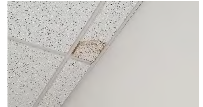
Conference Room: Evidence of water leaks in SE corner of room.
