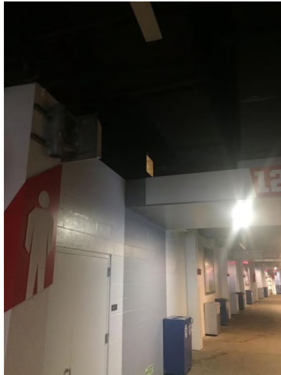
100 Level Electrical Rooms: Unrated penetrations through rated assemblies.
