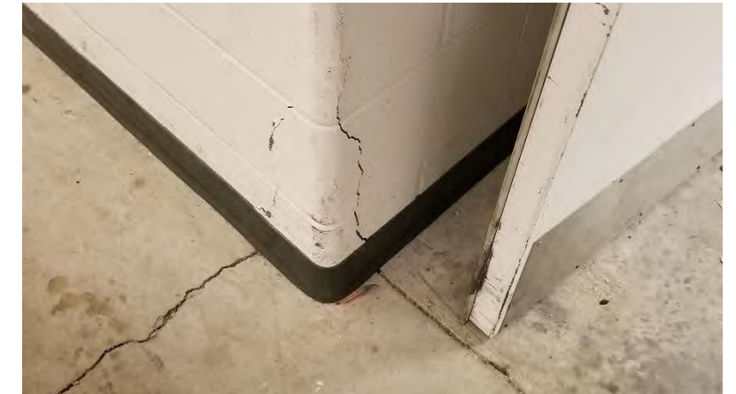
Slab-on-Grade Cracking: Shrinkage cracks have damaged masonry partition above. Joints should be sealed.
