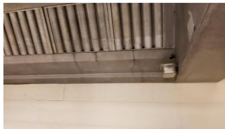
100 Level Pantries: Exhaust hoods exhibit a history of water intrusion
