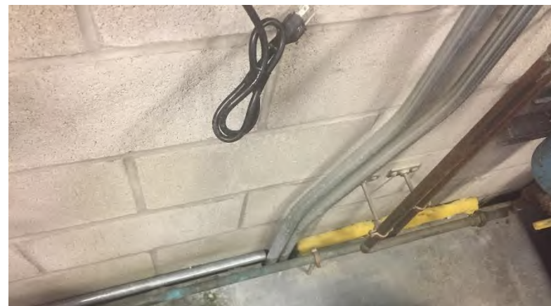
Storage 244.01: 1" Gap between floor without sealant or firestopping.
