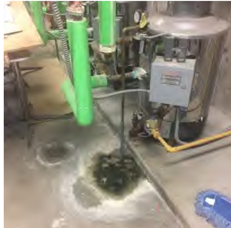
Mech 237.06: Water on floor from water heater overflow.
