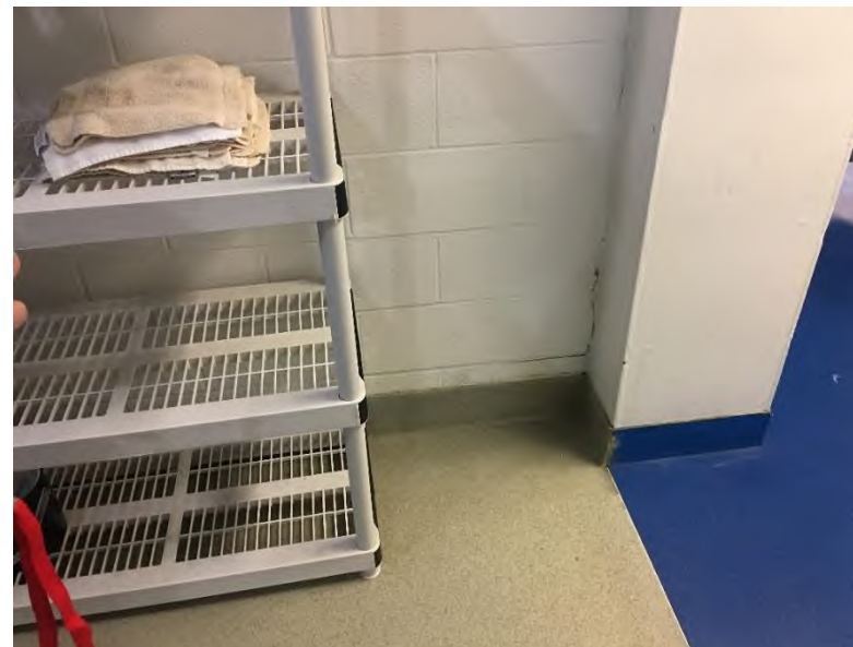
Bills Game Day Locker Room: Differential settlement of floor slab – note separation of joint along column.
