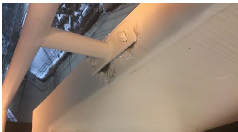
West End Suite Ramps: Deterioration of walls and connection to rails.
