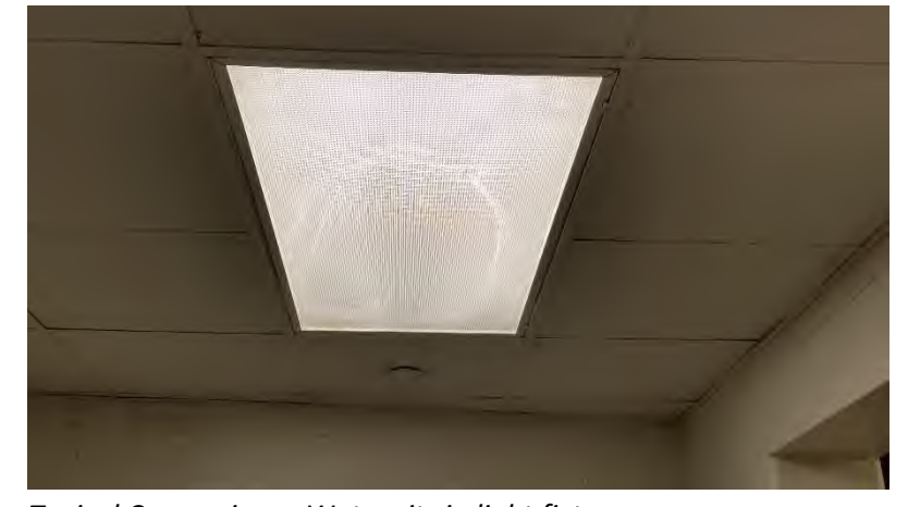
Typical Concessions: Water sits in light fixtures.
