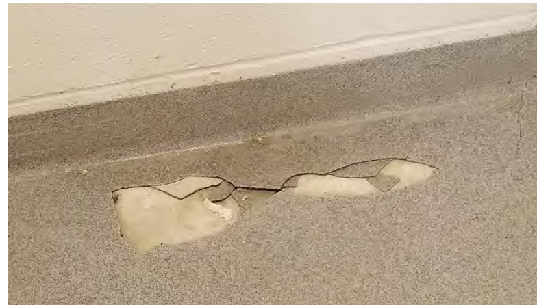
Men 430.01: Flooring substrate unsound. Flooring finish is cracked.
