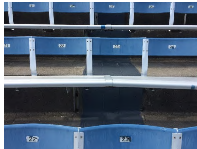
Upper Deck Seating Panels: Typical fixed construction joint in elevated seating panels.
