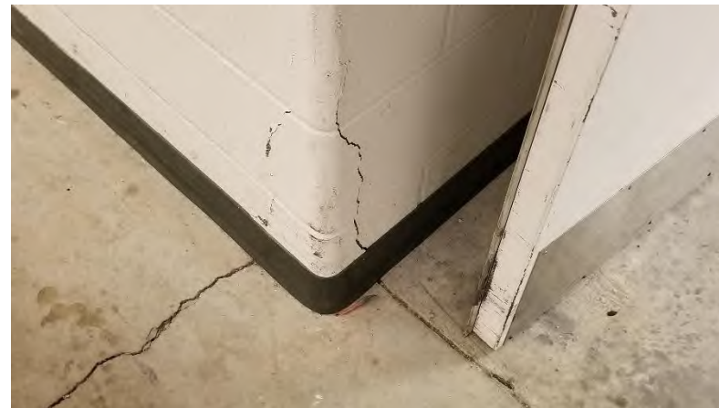
Commissary Main Corridor: Shrinkage cracks in the floor slab have propagated up into the masonry.
