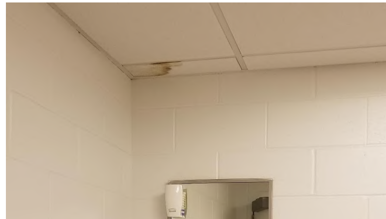
Toilet 023.07: Water damage at ceiling in NW corner of room.
