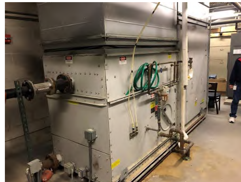
Ducted cooling tower for heat pump loop.
