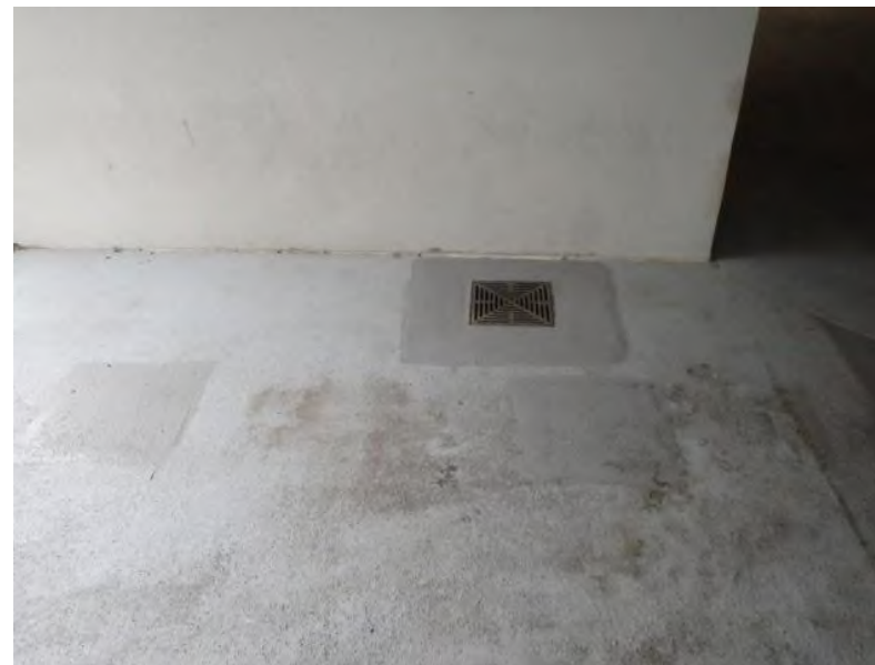
300 Level Concourse: Typical isolated repairs to coatings and around drain penetrations through the 300 Level Concourse slab.
