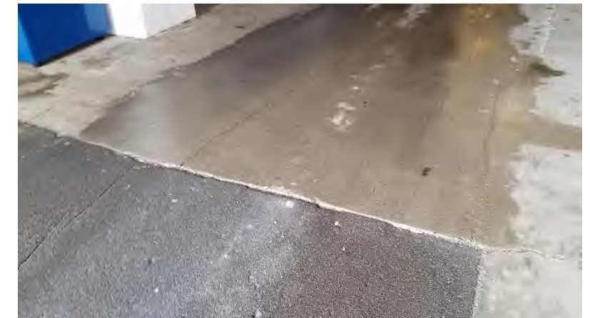
100 Level Concourse: Many differing pavement surfaces leave uneven joints and poor water drainage throughout the concourse.
