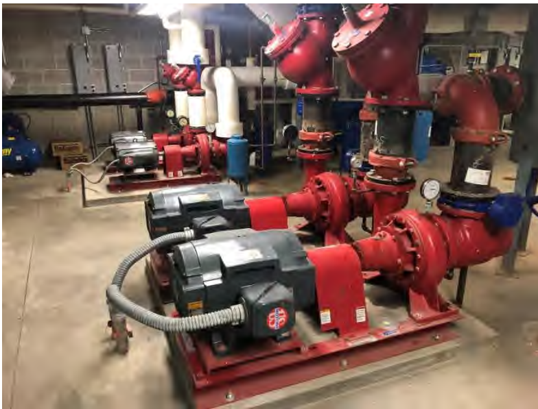
Heat pump condenser water circulation pumps.
