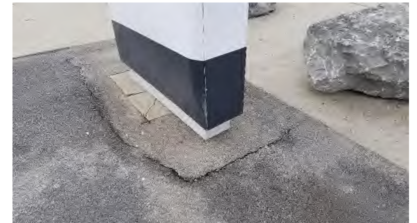
Pylon Signs: Several pylon signs exhibit impact damage.
