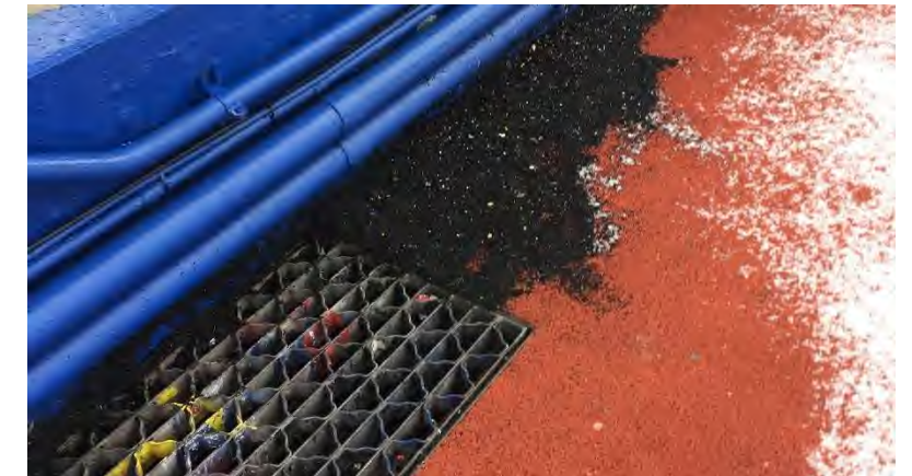
Field Drainage: Substantial buildup of turf granules at and within drainage areas. Noticeably used for paint disposal in past.
