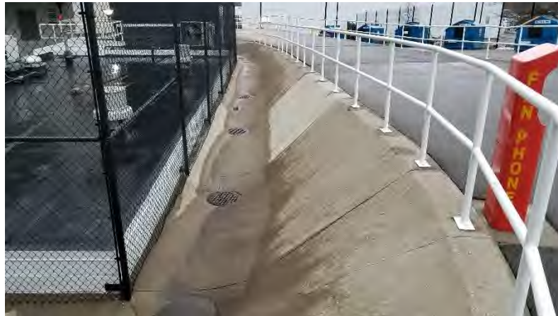
200 Level Concourse: At NE & SE corners, concrete surface drainage troughs are unsightly and not well protected.
