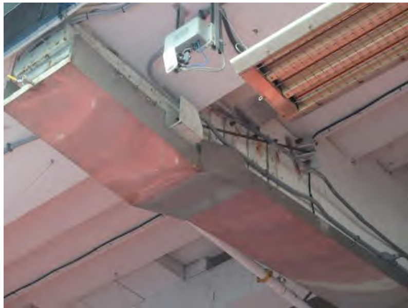
Typical Upper Level Seating Area: Underside of rakers have received metal gutters for leakage and drainage control over seating areas.
