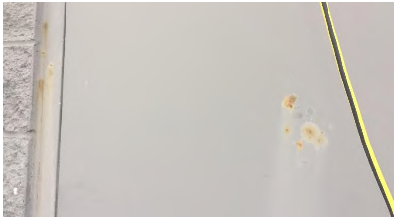
Pump House: Doors show signs of internal rusting.
