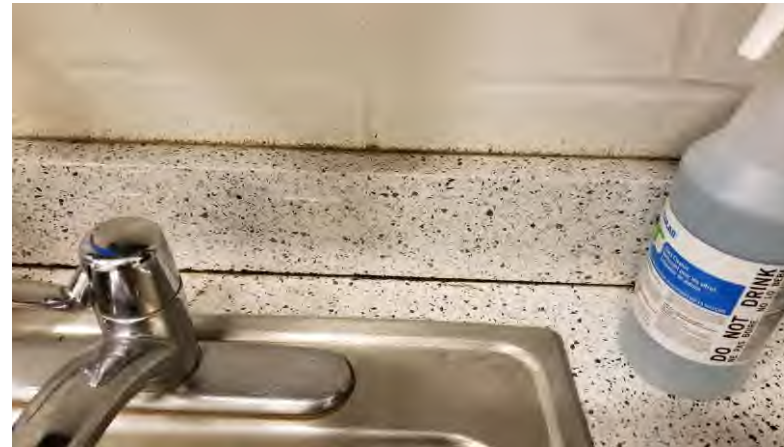
Break Room: Clear acrylic sealant at countertops is stained in nearly all locations within the Commissary. Since this condition happens nowhere else in the stadium, the culprit may be the cleaning methods used.
