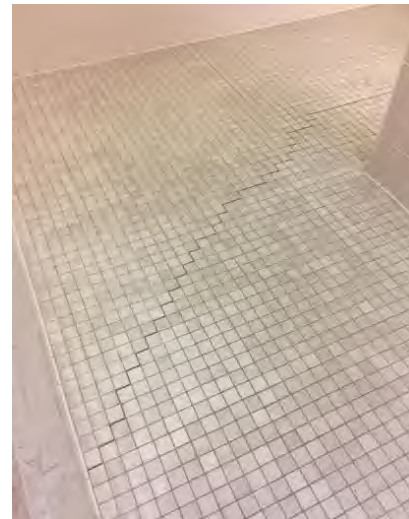
Women's Restroom 213.04: Tile flooring is cracked; appears to indicate movement in floor structure below.
