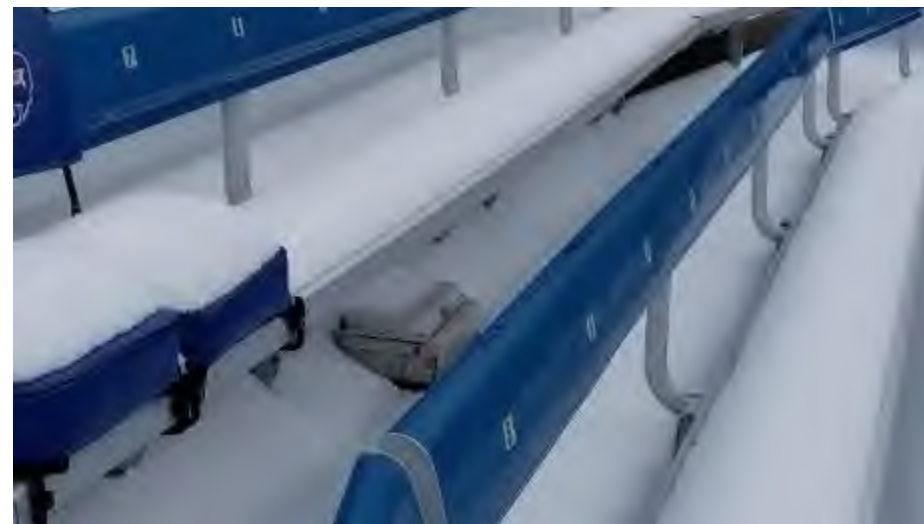
Figure 2- Under seat wireless enclosure
