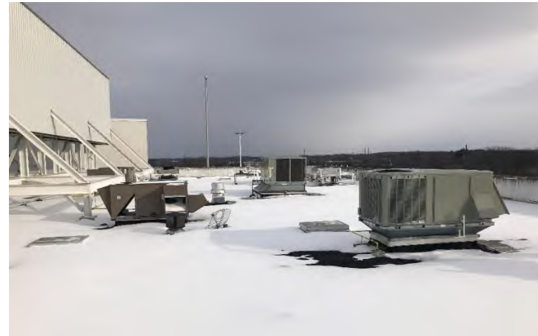
Older RTU on left in need of replacement.
