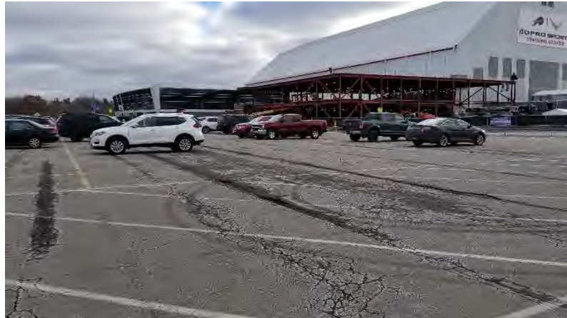
Parking Lot #2: Old trenches through asphalt are deteriorating.
