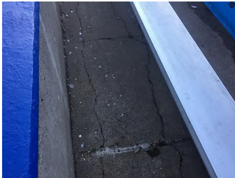
Lower Bowl Seating: Typical cracking of front row of on-grade seating slabs related to rotation of lower ringwall.
