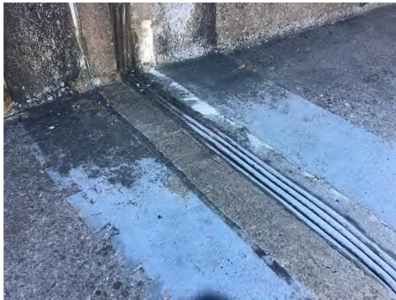
Upper Deck Seating Panel: Typical elevated seating panel expansion joint.
