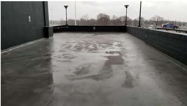
300 Level Ramp Landings: Traffic coatings become damaged from snow removal processes at all four upper ramp landings.
