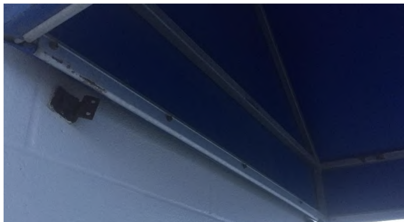
West end suite entrance awnings: Structural supports and mounts damaged, rusted or completely dislodged.
