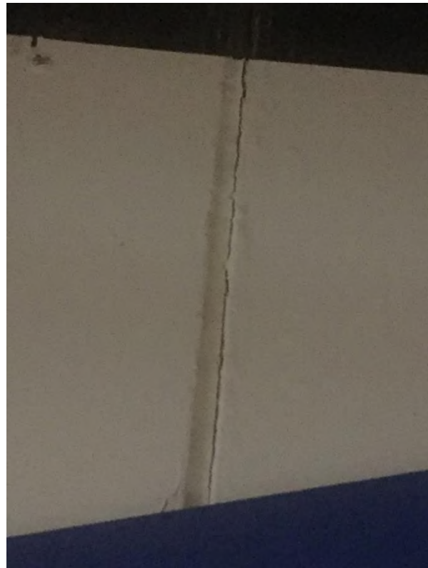
100 Level Concourse: Expansion joints between paired concrete columns were recently repaired, but show signs of sealant failures.
