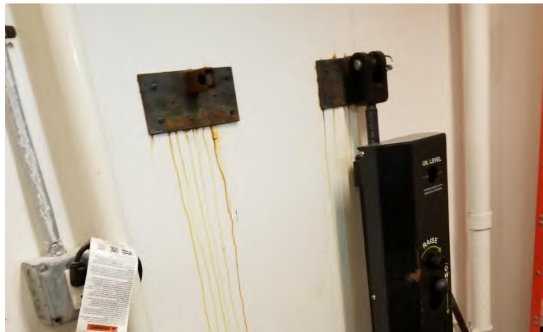
Storage 021.02: Water damage at connections penetrating foundation wall.
