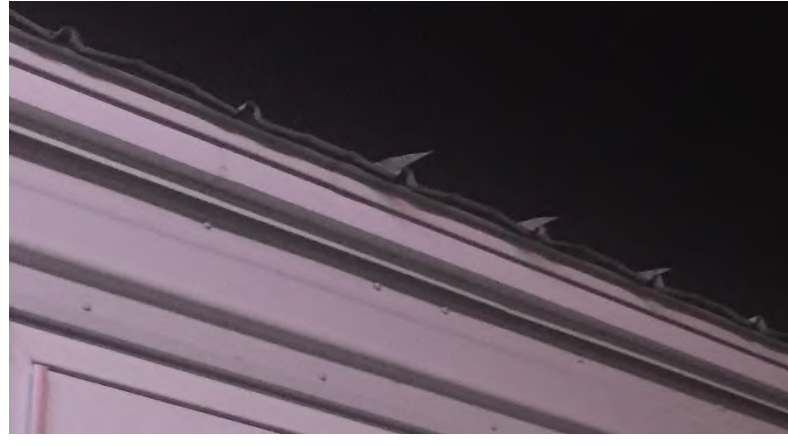
West End Camera Booths: No snow clips or ice prevention. Exposed, uncapped fascia at standing seam roofs.
