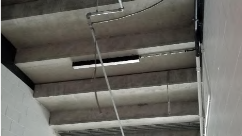
100 Level Vomitories: Dislodged backer rods from joints in bowl structure overhead.
