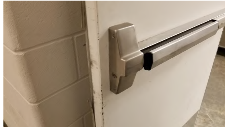
Commissary Kitchen: Pair of doors leading to the main kitchen are dinged up, smoke seals are damaged.
