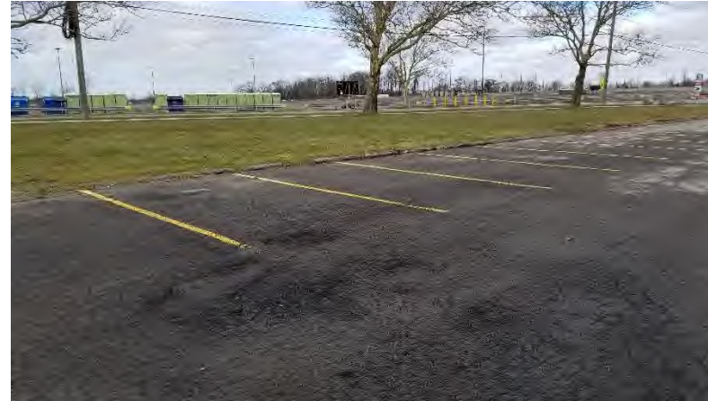
General Parking Lot Item: Many asphalt lots are deteriorating. Bills replace/repair on a rotating basis with County funds.
