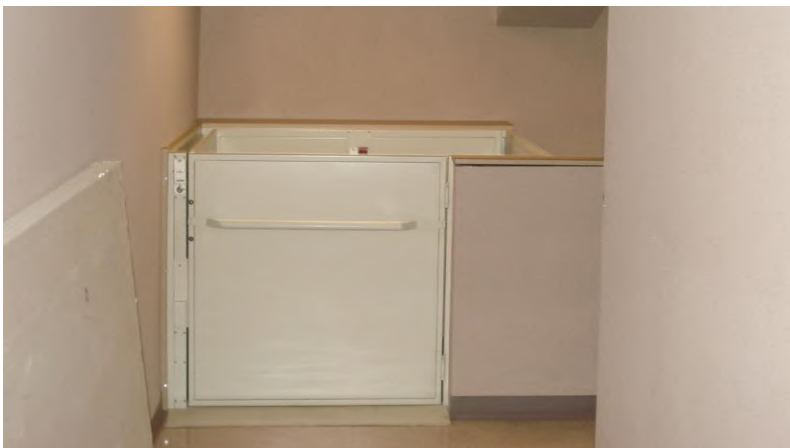
Dugout Suites: All Dugout Suites are provided with chair lifts – most not having proper approach clearances.
