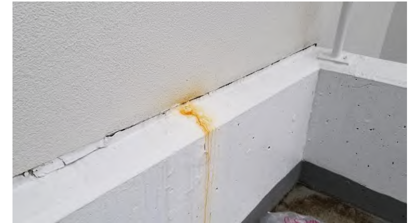
300 Level Stair Landings: Open joints at base of EIFS walls.
