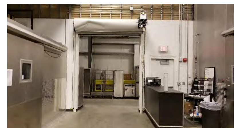
High-Bay Area: Impact damage to overhead door hood.
