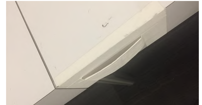
National Broadcast booth: Solid surface flip tops removed and replaced with laminate flip tops. Flip tops show significant damage and modifications from original design and likely need to be replaced.
