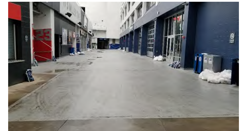
100 Level East Concourse: Traffic coatings are damaged by snow removal, and allow water to leak into spaces below. The topping slab and traffic coating were replaced most recently in 2018.
