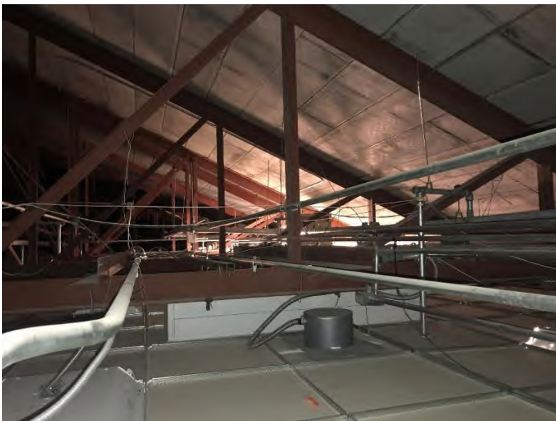
Cold cavity above Level 300 restrooms where heater and insulation might be added.
