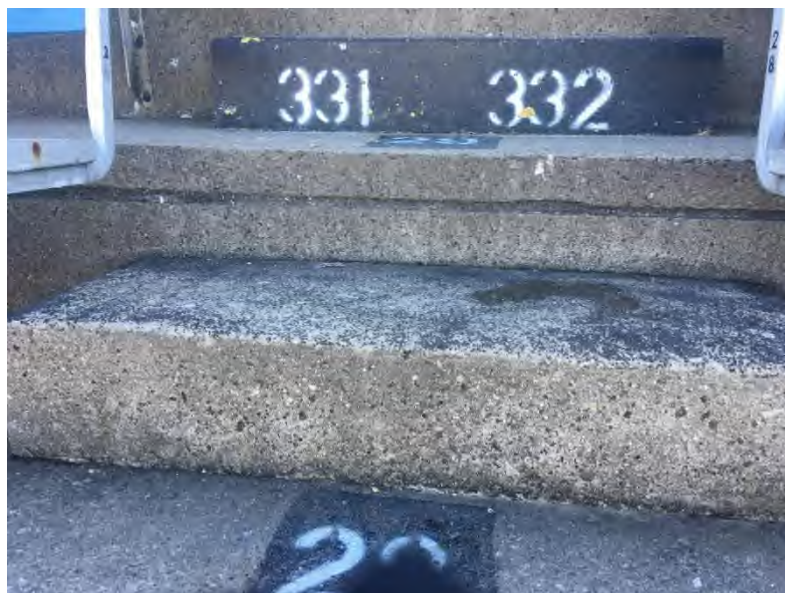
Upper Deck Seating Panels: Typical cast-in-place concrete tread.
