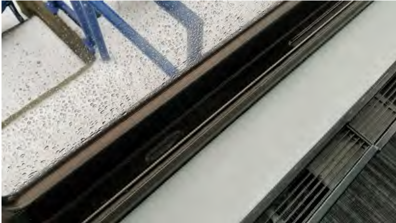
Dugout Suites: Suite windows reportedly leak in many locations. Observed leaks pond water in window tracks.
