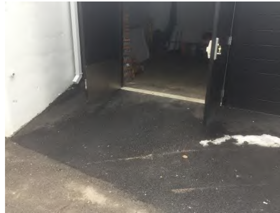
New storage adjacent to 117.09 Women: Ramp outside of door not accessible. Railing along accessible route removed.
