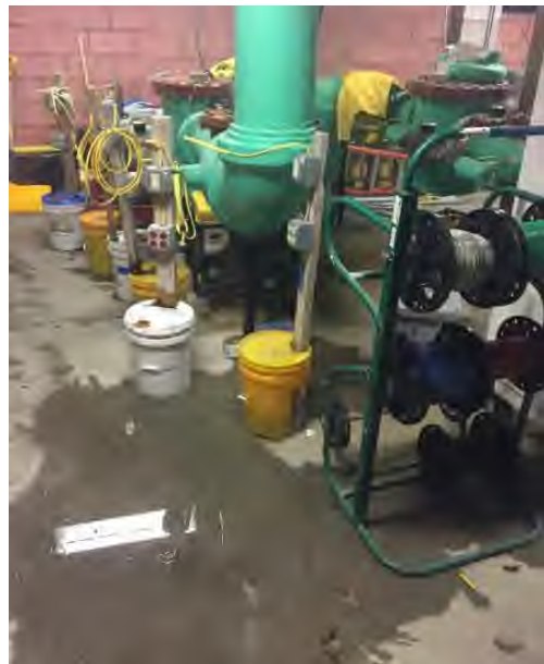
Pump Building: Roof leak overhead.
