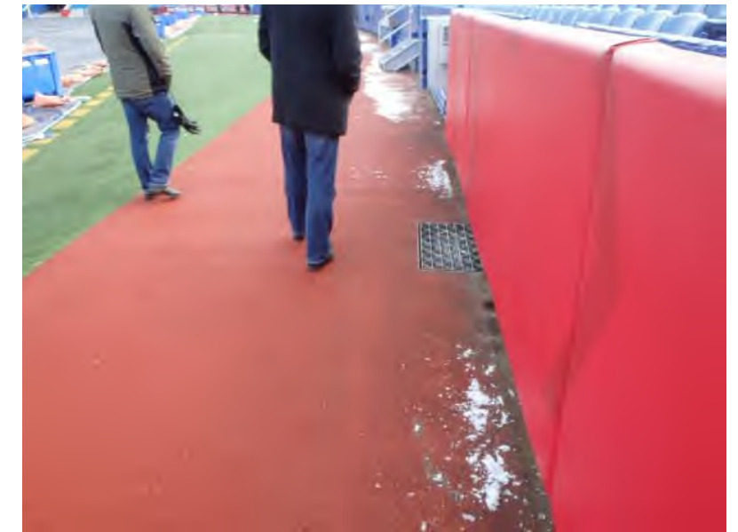
Lower Ring Wall: View of leaning, out-of-plumb Lower Ring Wall. This view indicates the Field Drainage System that is located below-grade along the perimeter of the Lower Ring Wall.
