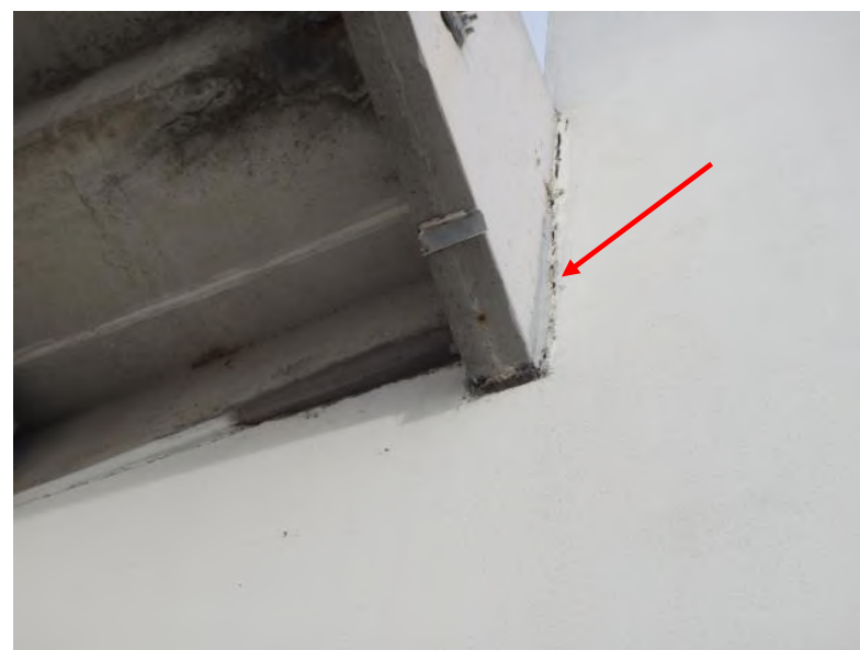
Cast-in-Place Concrete Frame: Arrow indicates failing protective vertical sealants.
