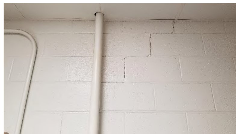
Concession 136.05: Movement between structure and masonry walls.
