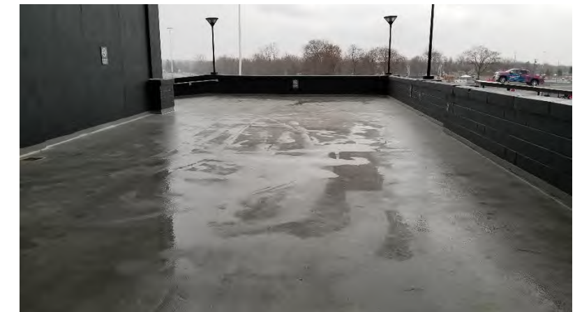
300 Level Ramp Landings: Traffic coatings become damaged from snow removal processes at all four upper ramp landings.
