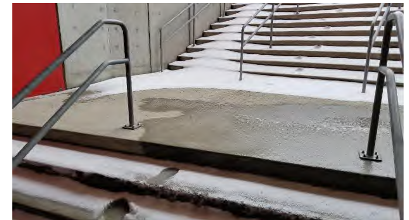
Monumental Stairs: Stair landings exhibit significant spalling due to application of salt.
