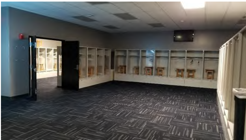
Visitor's Locker Room 023.31 : No compliant exits provided from room (door configurations, damaged hardware). Building Code.
