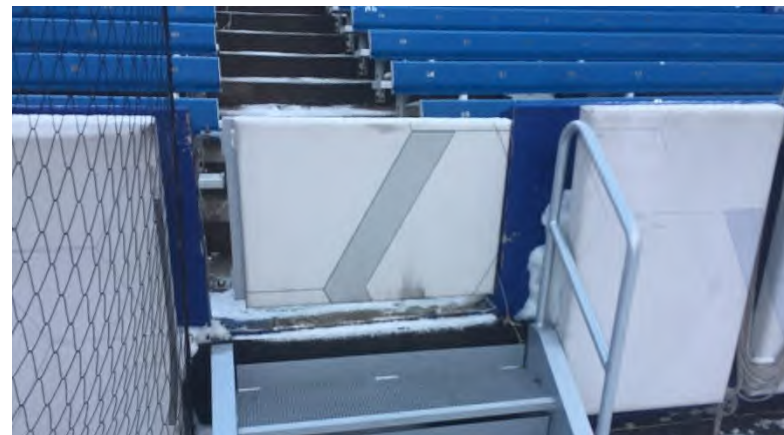
Field Access/Egress: Temporary wood stair units were recently replaced with metal units. Railings are not provided on both sides and do not have extensions.
