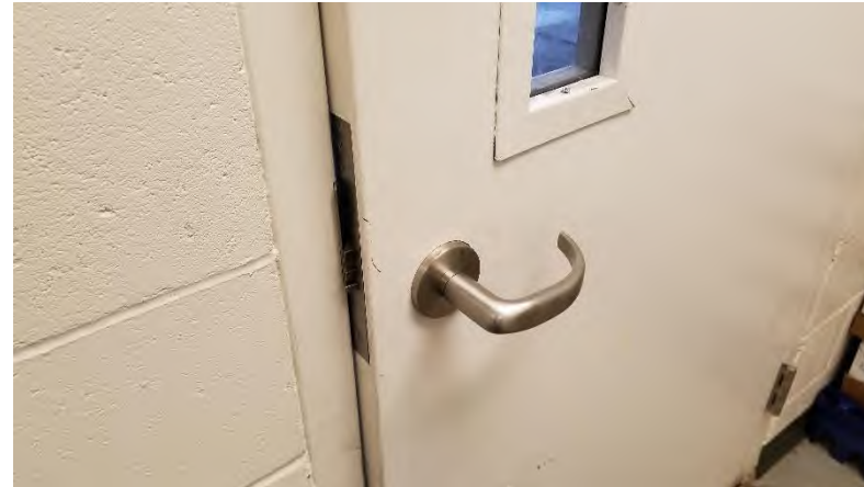
100 Level Concessions: High-use doors often do not close and latch, exhibiting a need for closer adjustments or latch adjustments.
