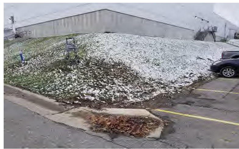
Tunnel Lot: Steep slopes around this area are disturbed by vehicles and are eroding in many places.
