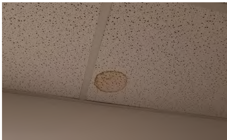
Office 023.27: Water damage at ceiling.
