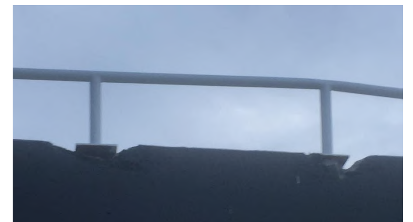
Corner stairs to 300 level: Deterioration of walls and connection to rails.
