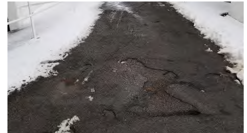
East End Zone Ramps: Asphalt ramps are frequently damaged where water collects and where vehicles make turns.
