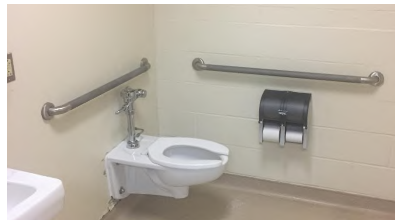
Sideline Medical and Security Restrooms: Missing vertical grab bars.
