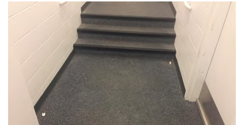
Corridor 021.01: Rubber Flooring shows substantial wear from cleats and traffic.
