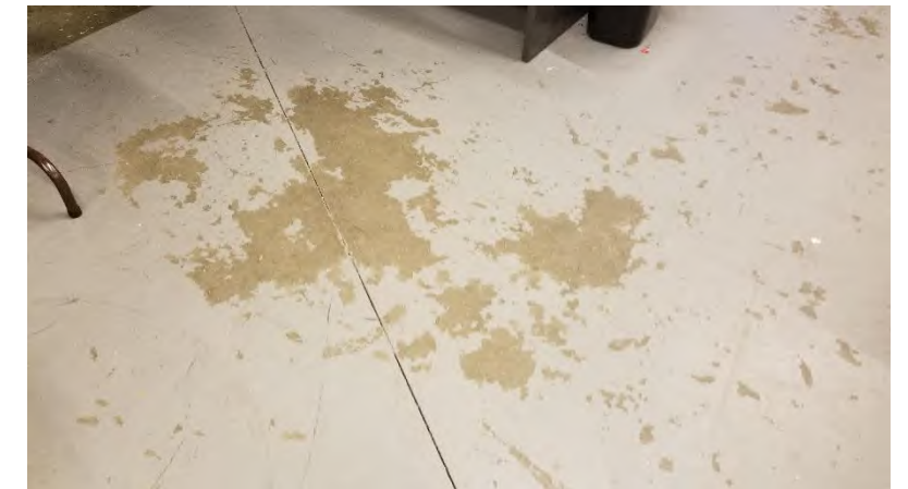
Warehouse Flooring: The tinted sealer coating is damaged in several areas.
