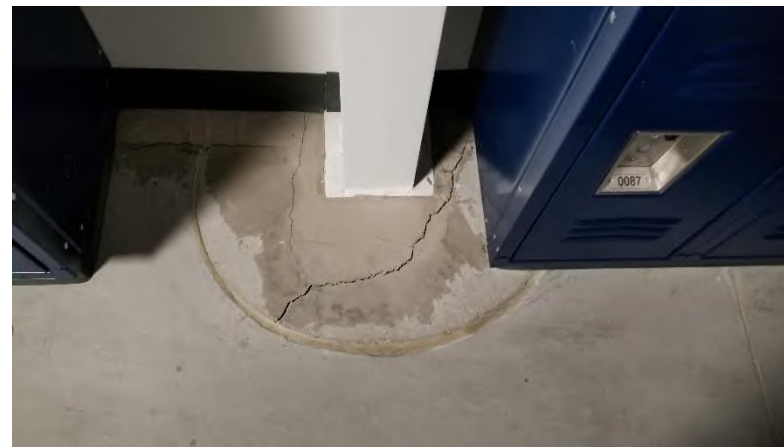
Men's Locker 3009: Slab movement at base of Column V1.
