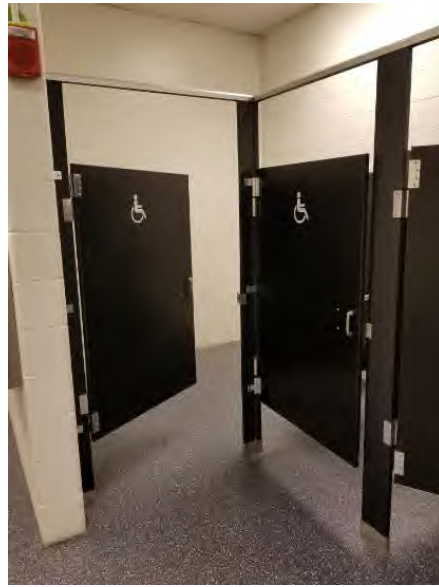
“Accessible” Stalls: Older toilet stalls labeled as accessible typically are not dimensionally compliant, do not have doors swinging in the correct direction, do not provide required types of stalls, or do not have required accessories.
