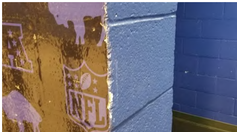
Game-Day Locker Room Entrance: Impacts have damaged corners of masonry walls.
