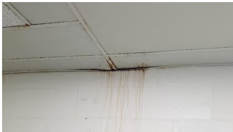
Toilet 021.21: Water damage at ceiling.
