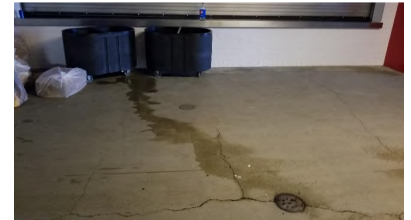
Concourses: Trash leaks onto slab, often seeping into floor cracks.
