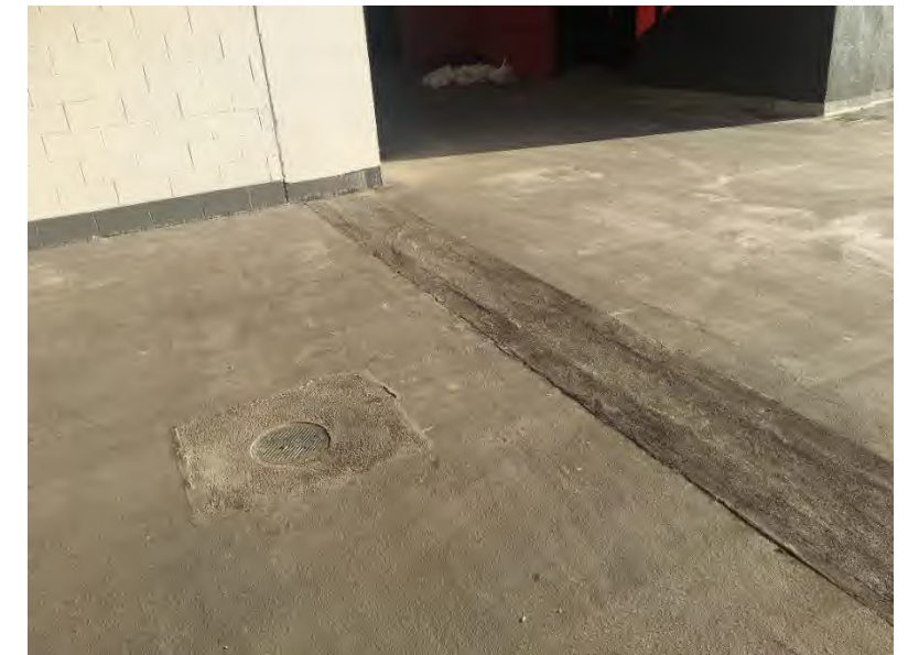
300 Level Concourse: Typical expansion joint and floor drain – note roofing material over joint.
