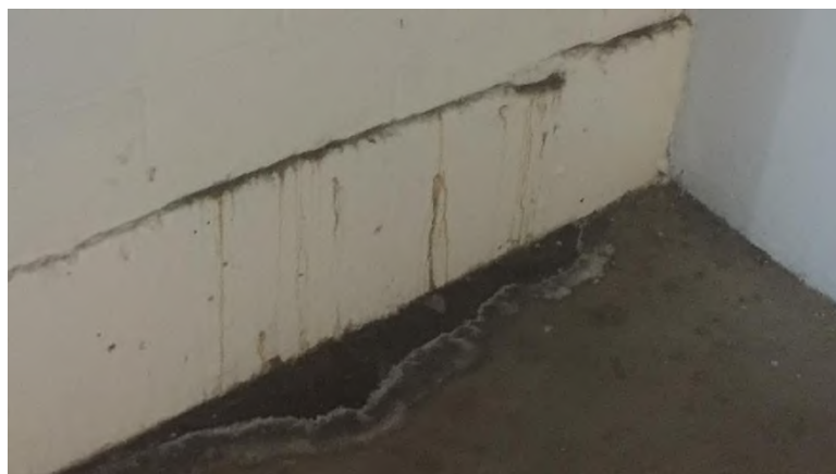
Mech 119.06: Water leaking through foundation retaining wall
