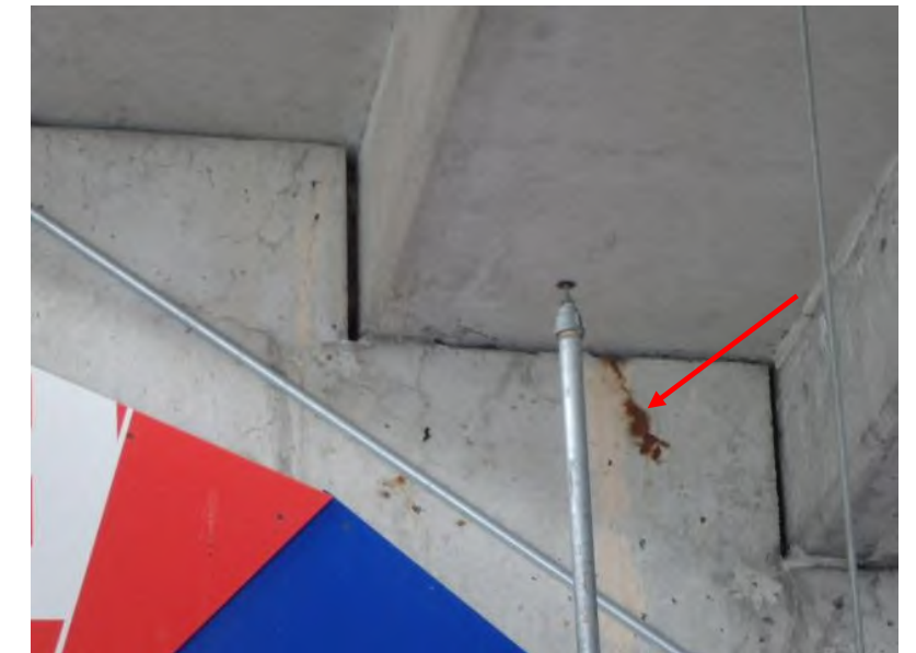
Cast-in-Place Concrete Frame: Arrow indicates previous overhead concrete repair by epoxy injection applications.
