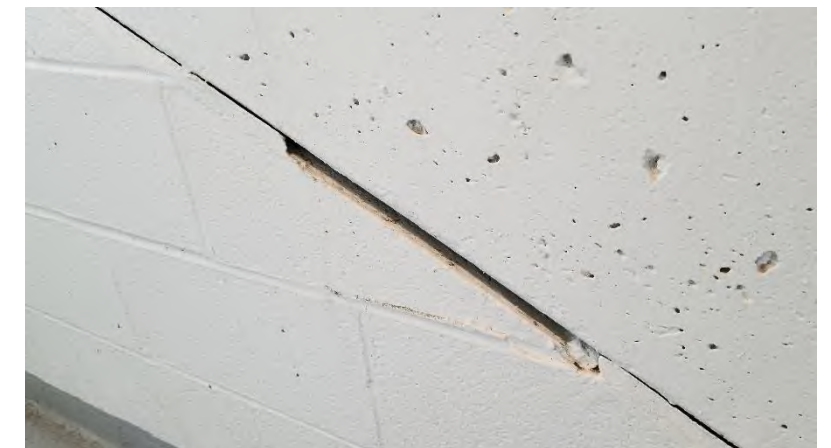
200 Level Corner Retail Stands: Sealant joints between masonry walls and the concrete stair structure above have failed, allowing water into the interior.
