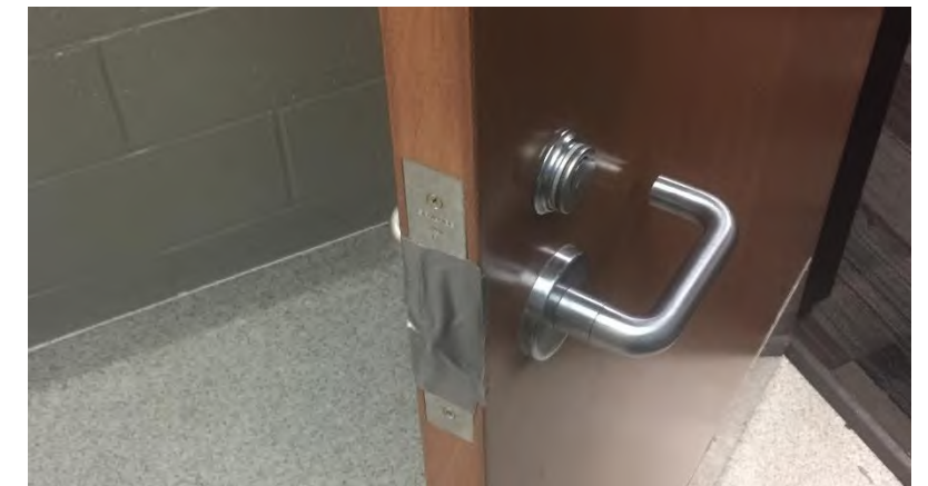
West End Support Spaces (restrooms, janitors): Hardware either does not work or locksets need to be updated to facilitate appropriate access to proper keys. 3-4 instances.
