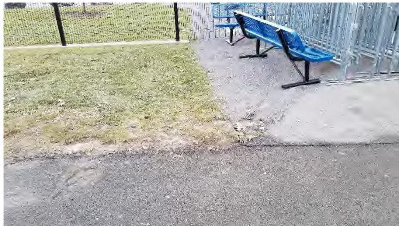
Crushed Granite: Crushed granite surfacing is subject to erosion and mechanical displacement.
