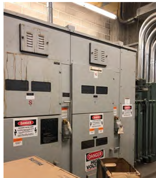
Existing Substation with 1972 transformer
