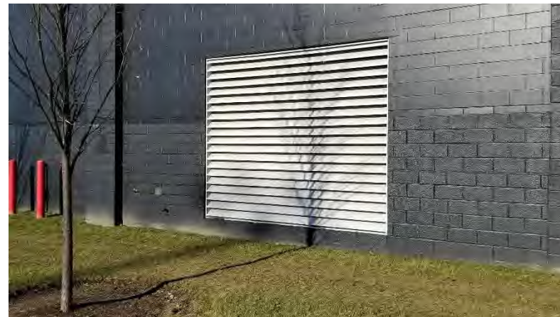
Exterior Mechanical Louvers : Six louvers on sidelines located near ground, subject to potential terrorist attack. DHS Safety Act.
