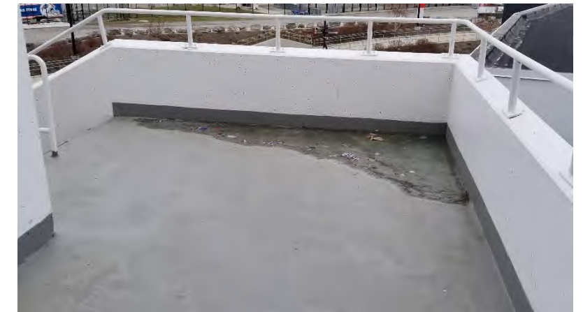
300 Level Stair Landings: Slabs do not slope toward drains.
