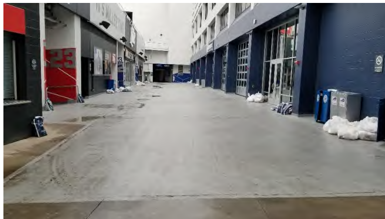
100 Level East Concourse: Traffic coatings are damaged by snow removal, and allow water to leak into spaces below.
