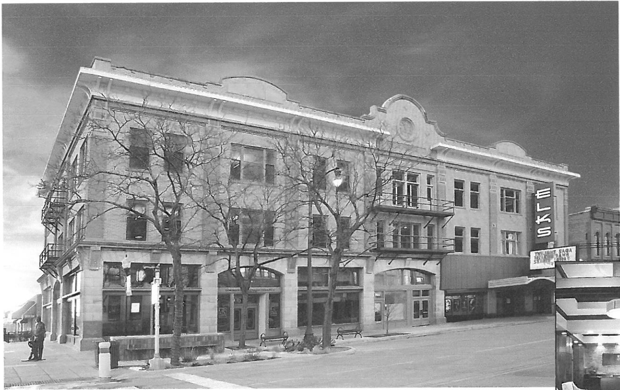
Name: Downtown Elks Building (Historic Remodel) Owner: Downtown Elks LLC Square ft: 20,000 Date completed: 2011 Cost: 3.5 million
