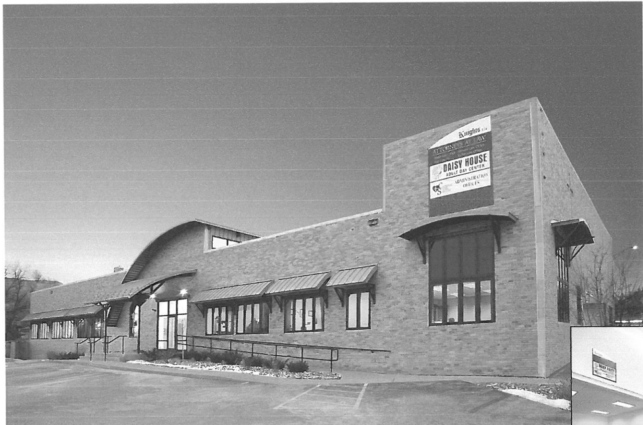
Name: Knights of Columbus Office Building (Remodel) Owner: Knights LLC Square ft: 13,000 Date Completed: 2008 Cost: 2 million
