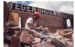
The Forget It floral shop at the corner of South 27th Street and Minnesota Avenue is demolished in July 1990. The site is a parking lot today. Source: The Press
