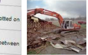
Polison as the Club was a popular hangout for the local community. It was demolished to make way for the new building. Source: The Press
