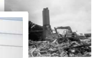
Club demolition at the intersection of 11th Street and 20th Street in June 1964. The club was formerly known as the Beacon Club and was a popular hangout for the local community. It was demolished to make way for the new building. Source: The Press
