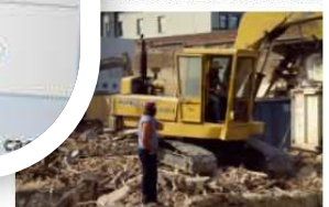
A building is demolished at the corner of North 29th Street and Second Avenue North in October 1992. The site is a parking lot today. Source: The Press
