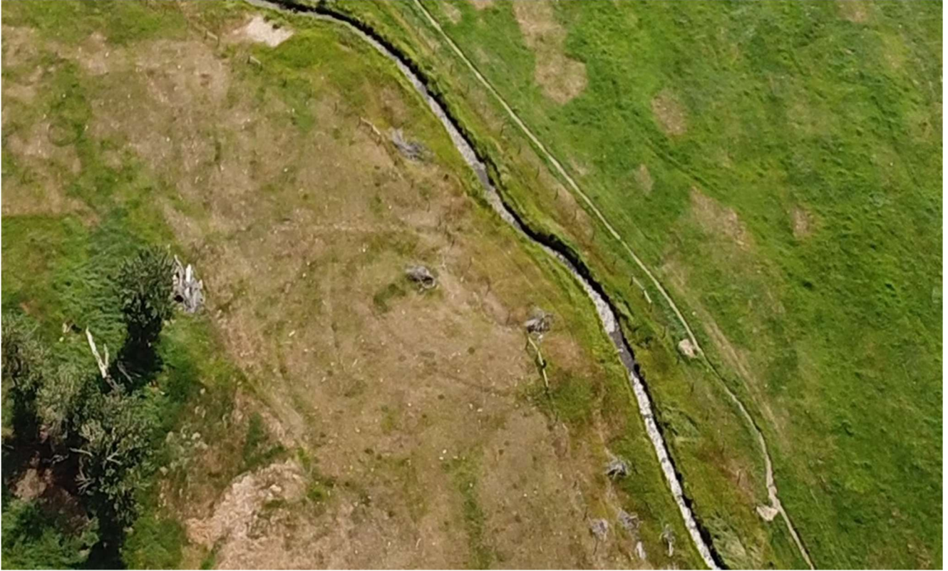
Figure 21. - Aerial view of project reach showing channel straightening-Photo courtesy of Madison Conservation District.
