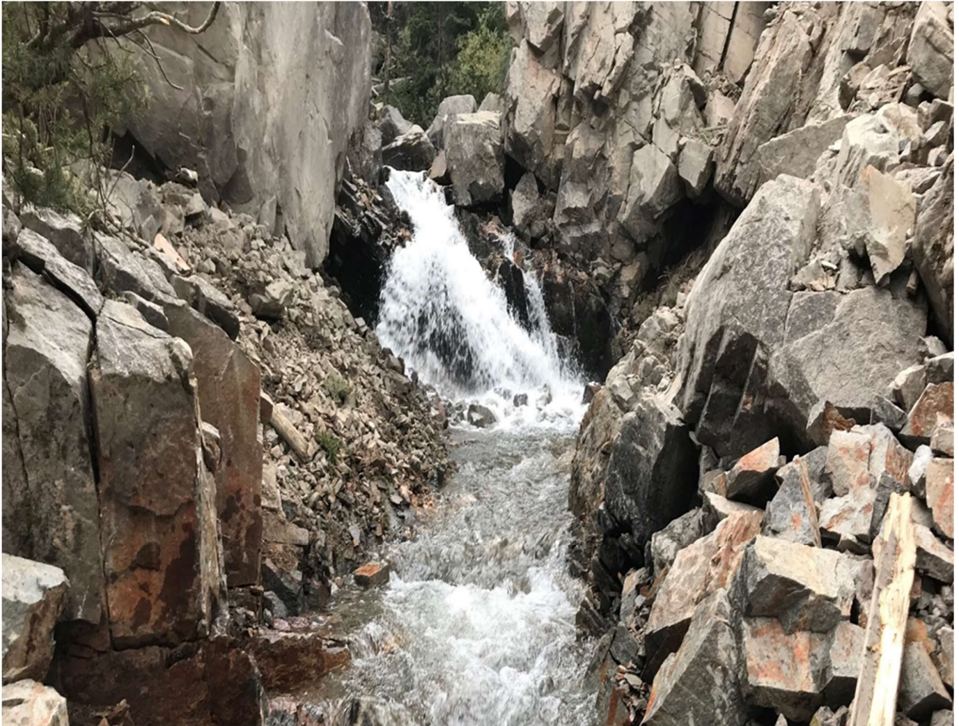
Figure 18. - Tepee creek enhanced waterfall after blasting of bedrock and removal of plunge pool. Photo courtesy of Allison Stringer Custer-Gallatin National Forest Service.
