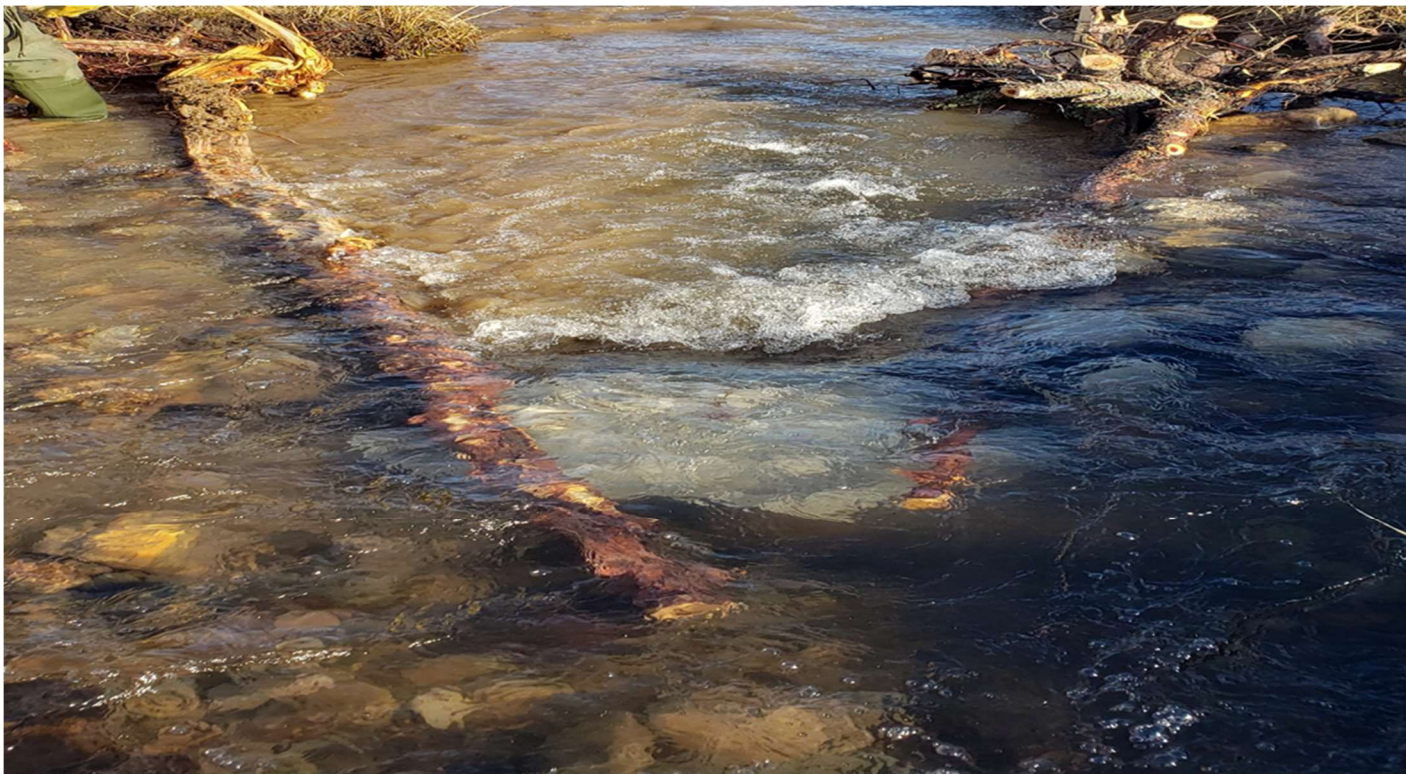
Figure 23.- Placement of instream structure for pool development.
