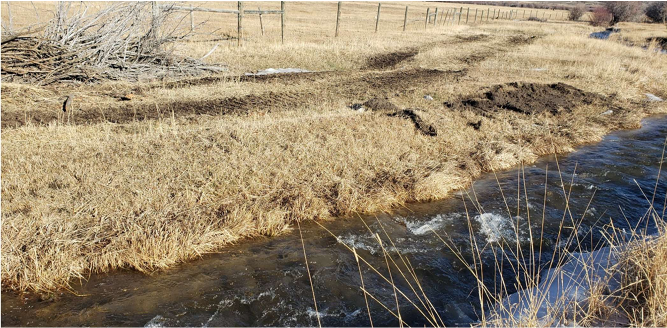
Figure 22. -Berm material removed to reconnect flood plain.
