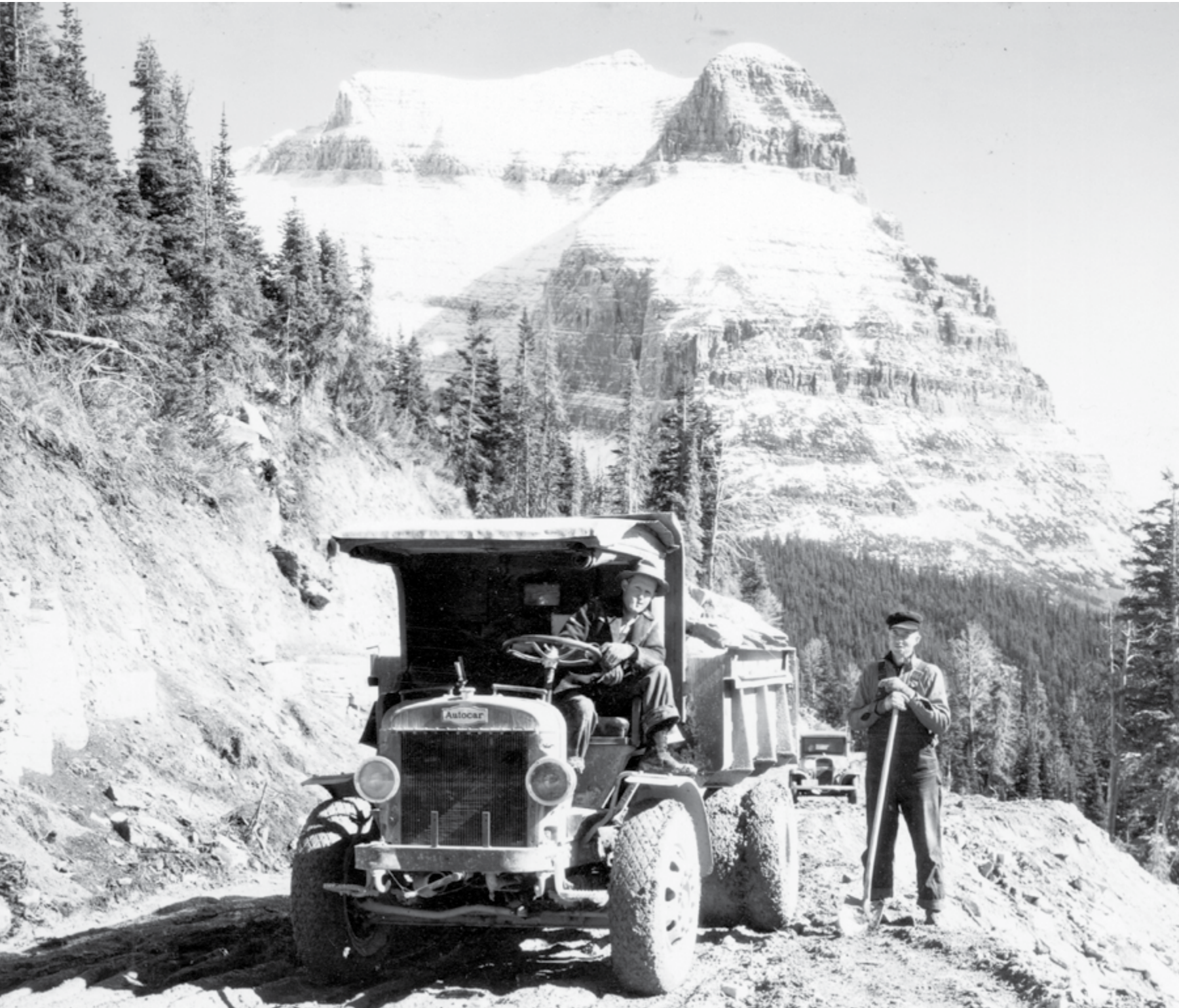
Construction equipment near Going-to-the-Sun Mountain, ca. 1932 / Glacier National Park Archives
