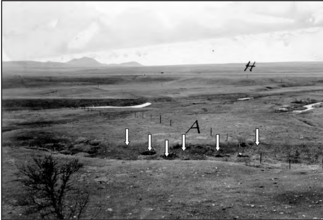
Figure 12. An annotated 1930s photograph of Nez Perce shelter pits located in the ravine at the siege area.
