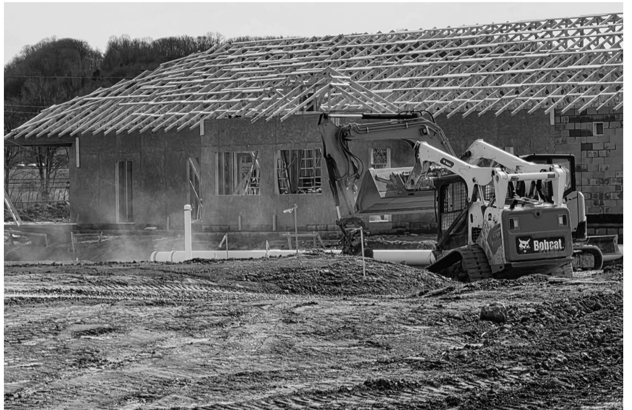
Staff photo by Charles Owens The unseasonably warm weather the region experienced earlier this month has allowed construction crews to make significant progress on Princeton's new wave pool and bath house project with both the walls and roofing on the bath house now going iup.
