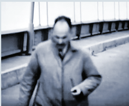
Coatsworth shuffles off the bridge, moments before it collapses.
